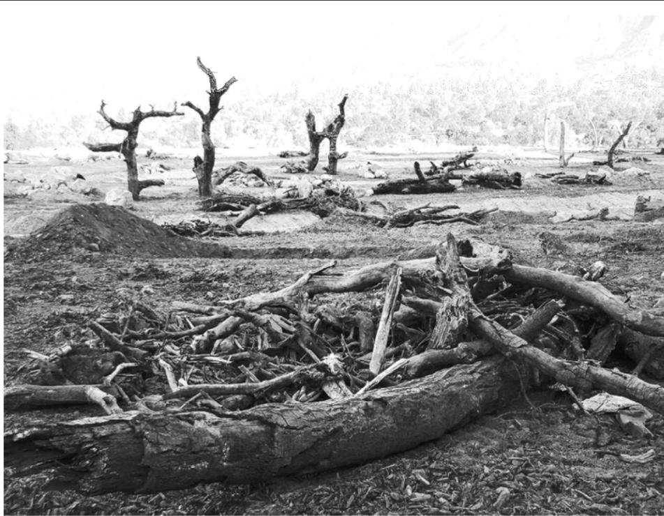
**October 2013.** The Lower Sediment Placement Site (SPS) following soil improvements (decompaction and incorporation of large volume of salvaged mulch) and the placement of salvaged natural snags, boulders, and coarse woody debris.
