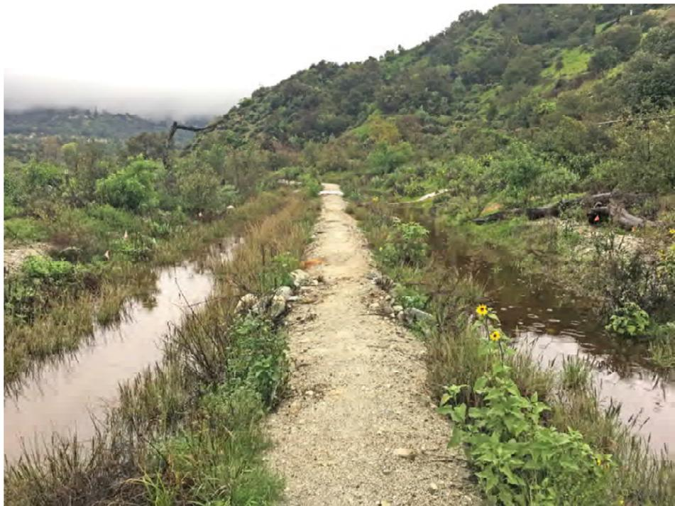
**February 2019.** Ephemeral flows occur in the designed spiraling drainages that convey off-site/on-site flows to an outlet tower in the center of the Lower Sediment Placement Site (SPS). Vegetation in the drainages is managed to facilitate the inspection/treatment activities of the San Gabriel Valley Vector Control District.
