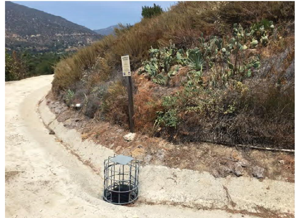
**August 2019.** In addition to providing project mitigation, the Lower SPS is part of a flood control facility; therefore, Public Works regularly monitors the SPS to ensure the integrity of the created landform. The Restoration Contractor periodically removes sediment and vegetative debris from the various v-ditches and inlets.
