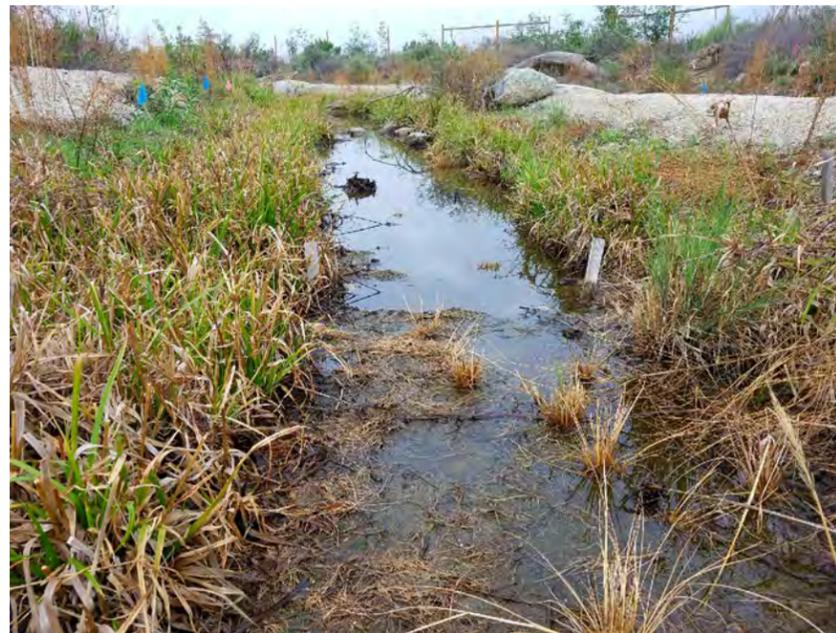
**March 2018.** Ephemeral flows occur in the designed spiraling drainages that convey off-site/on-site flows to an outlet tower in the center of the Lower SPS.
