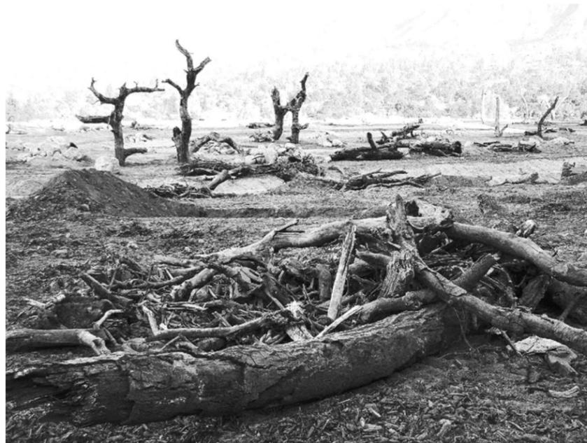
**October 2013.** The Lower Sediment Placement Site (SPS) following soil improvements (decompaction and incorporation of large volume of salvaged mulch) and the placement of salvaged natural snags, boulders, and coarse woody debris.
