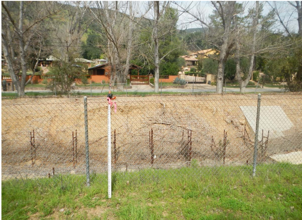
HEC-RAS RIVER STATION 19+06, CHANNEL AND RIGHT OVERBANK
