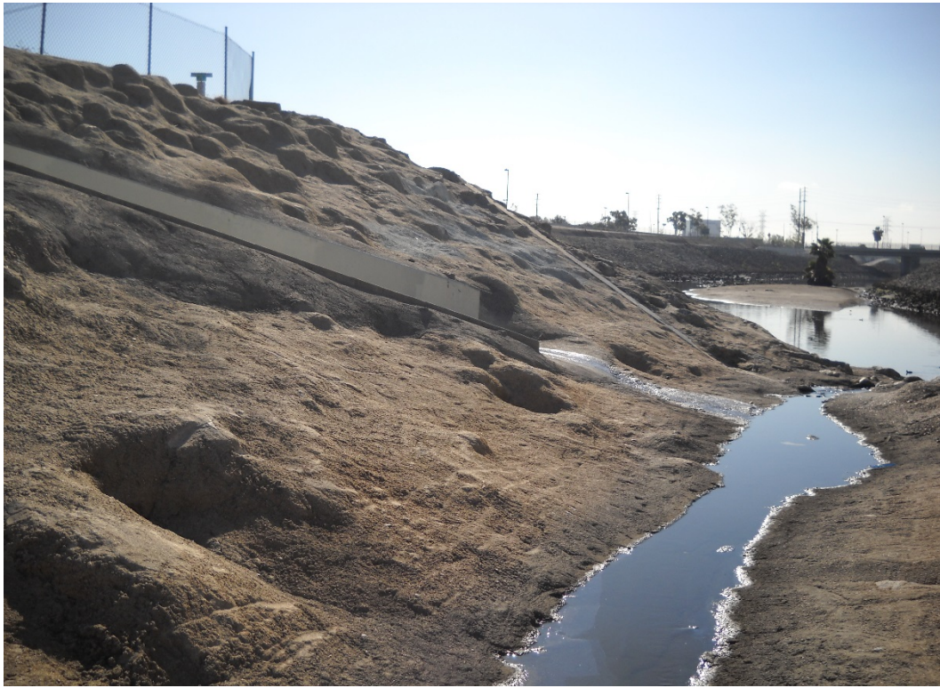
HEC-RAS RIVER STATION 01+01, DOWNSTREAM DIRECTION
