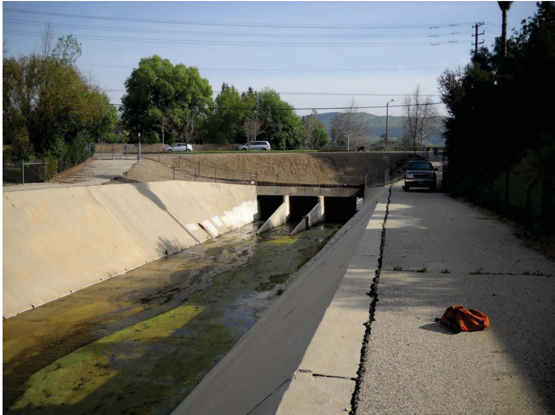
Figure 6-4. Box Culvert at Kanan Road
