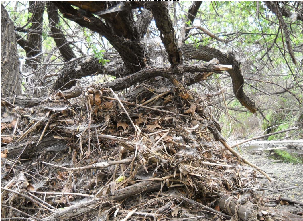
HEC-RAS RIVER STATION 31+89, DOWNSTREAM DIRECTION
