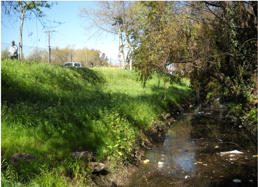
HEC-RAS RIVER STATION 7+74, UPSTREAM DIRECTION
