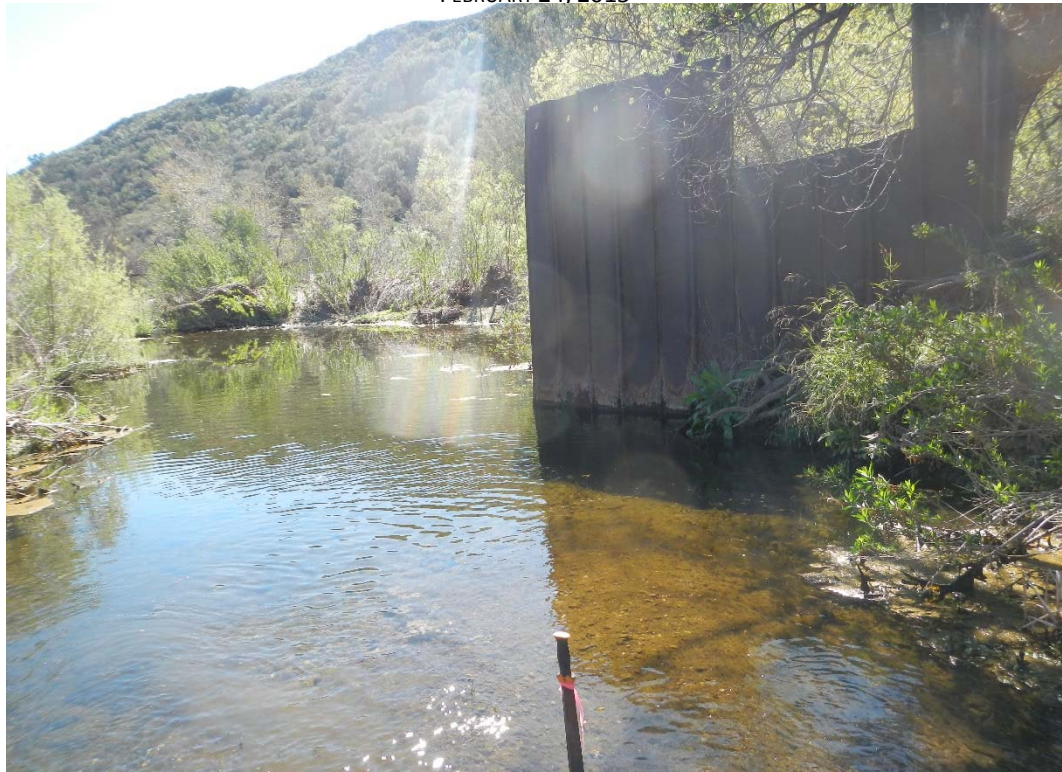
HEC-RAS RIVER STATION 7+67, DOWNSTREAM DIRECTION
