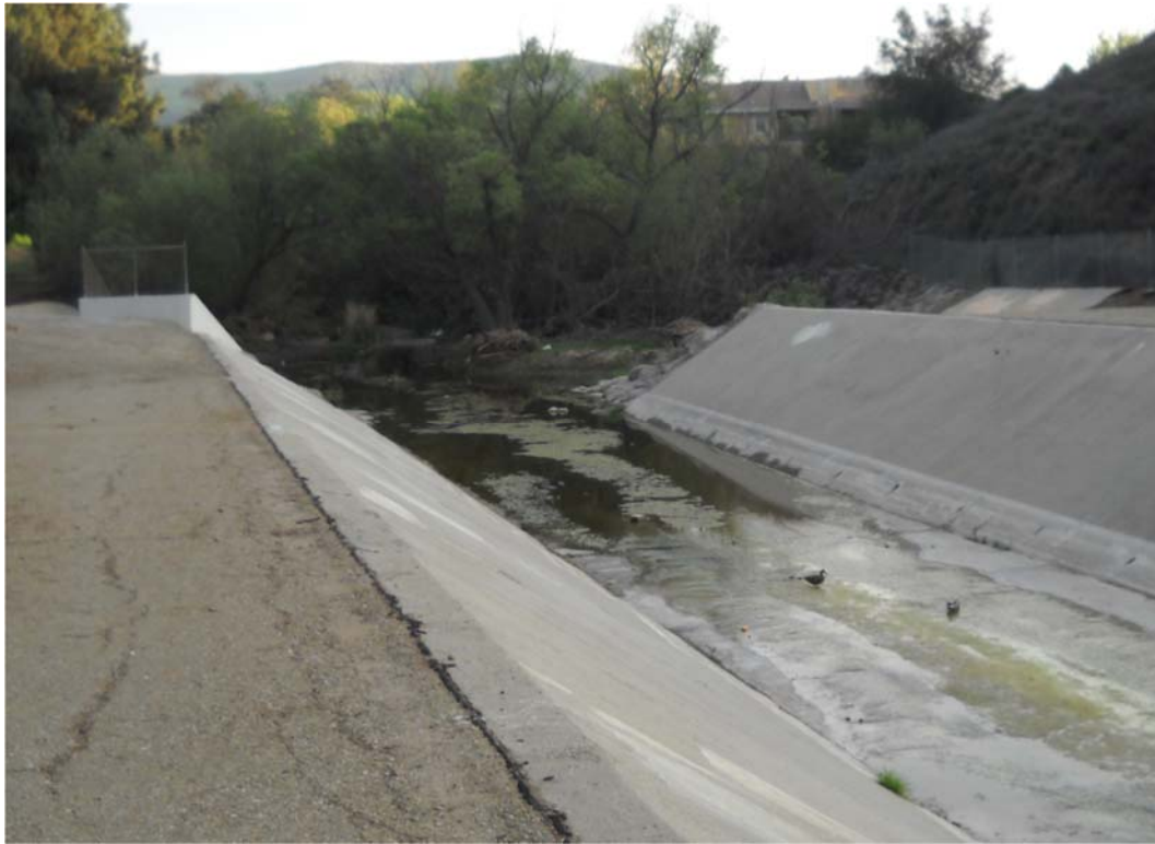
UPSTREAM EXTENT OF REACH NO. 34, HEC-RAS RIVER STATION 39+69, DOWNSTREAM DIRECTION
