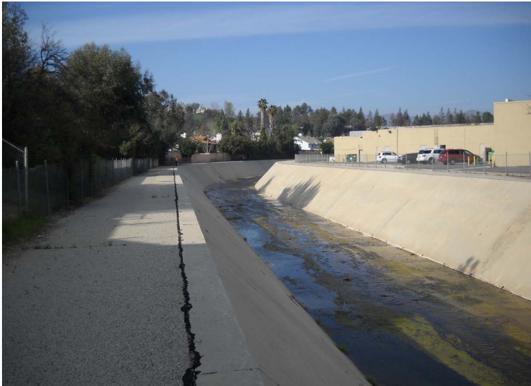
160 FT. UPSTREAM OF HEC-RAS RIVER STATION 46+40, UPSTREAM DIRECTION
