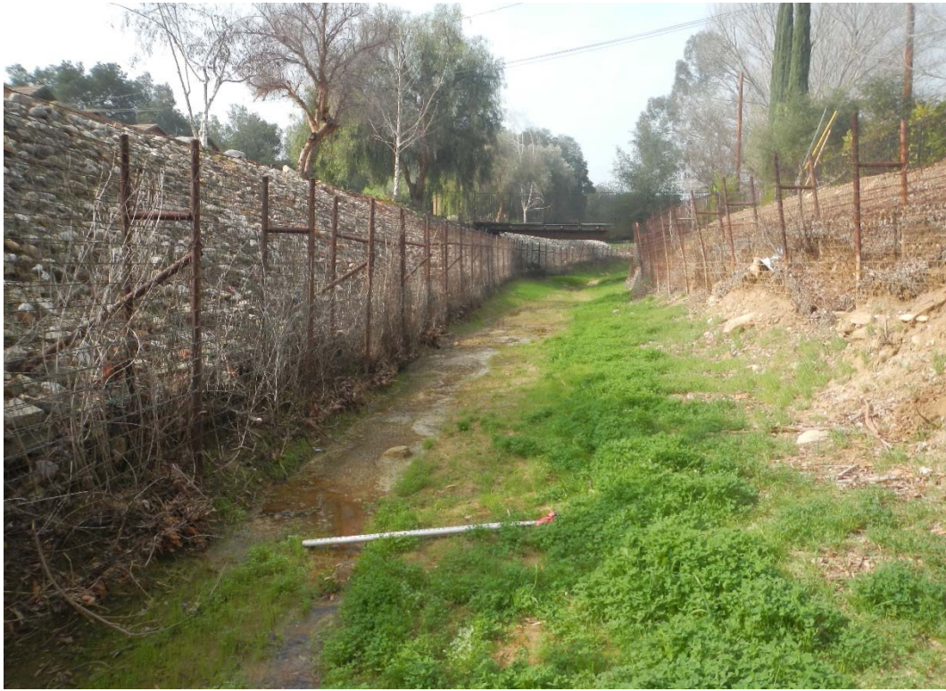
88 FT. DOWNSTREAM OF HEC-RAS RIVER STATION 22+78, DOWNSTREAM DIRECTION (PRIVATE DRIVEWAY BRIDGE)
