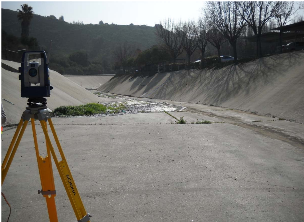
REACH DOWNSTREAM EXTENT, HEC-RAS RIVER STATION 7+88, DOWNSTREAM DIRECTION
