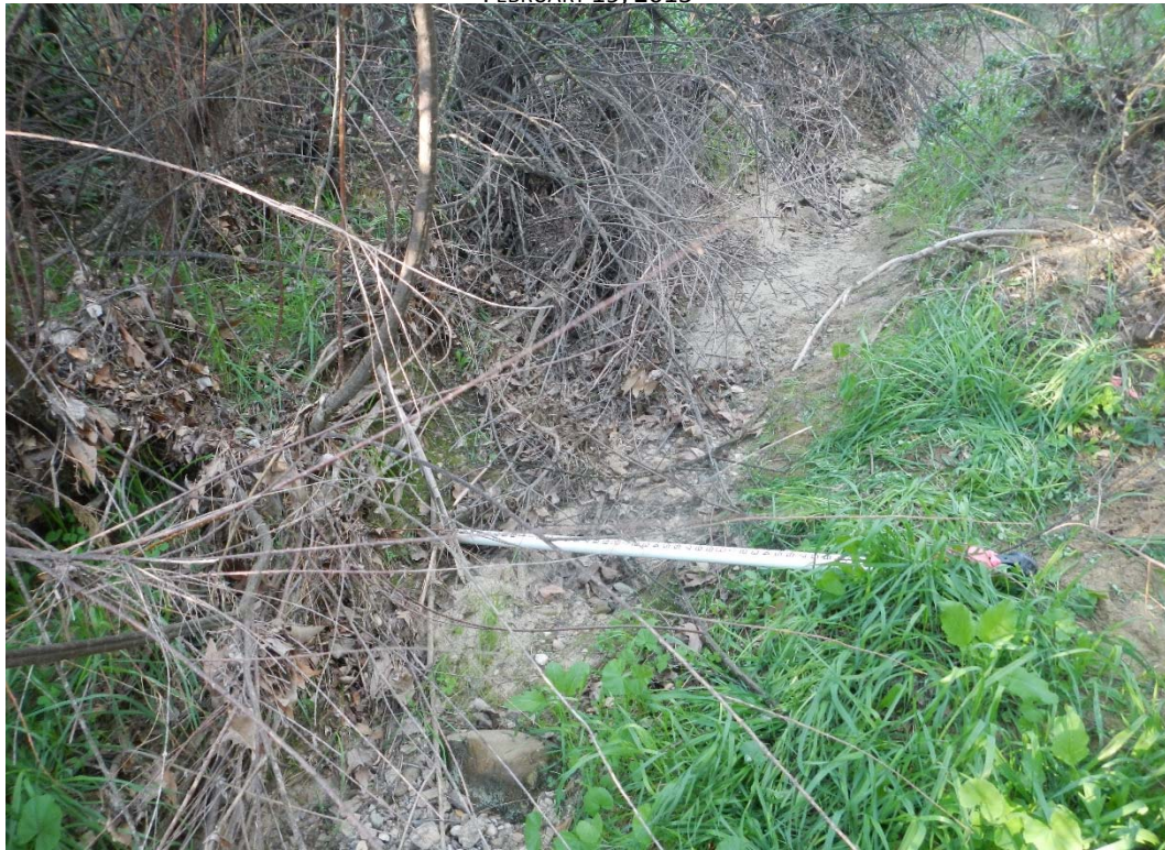
HEC-RAS RIVER STATION 5+69, UPSTREAM DIRECTION
