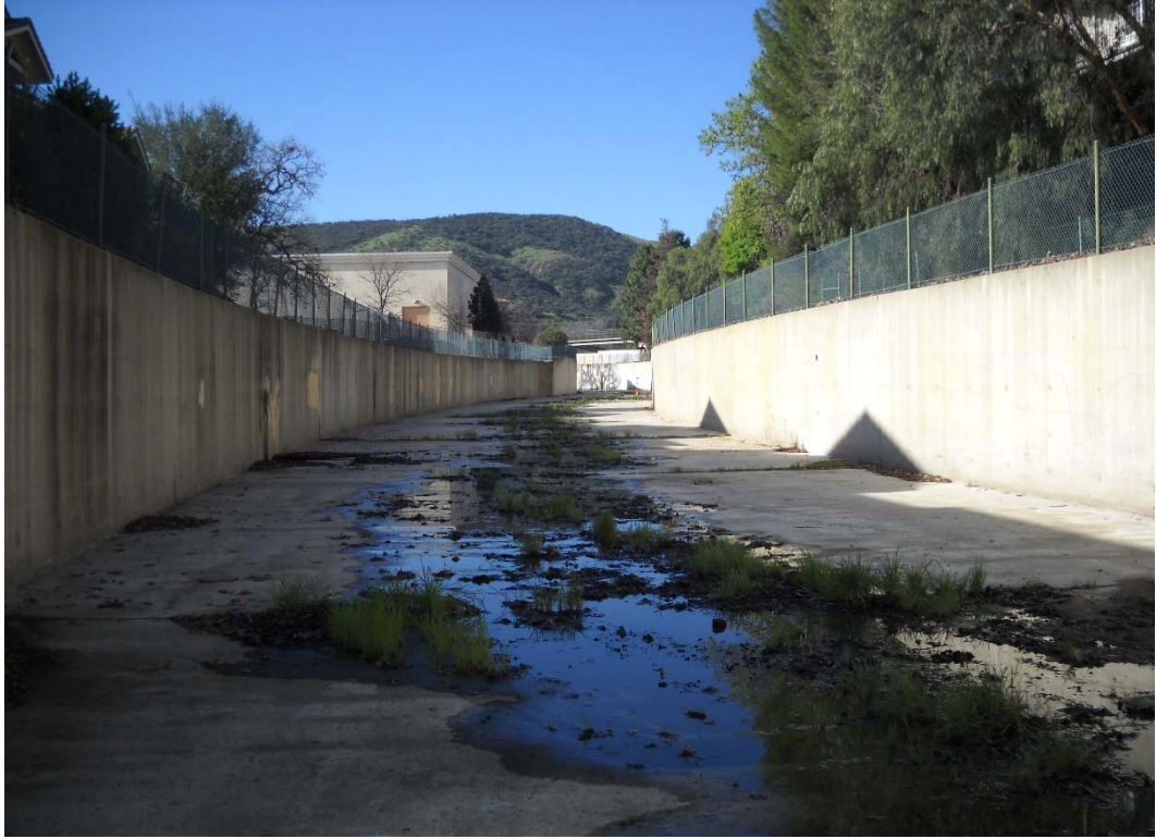
HEC-RAS RIVER STATION 7+00, DOWNSTREAM DIRECTION
