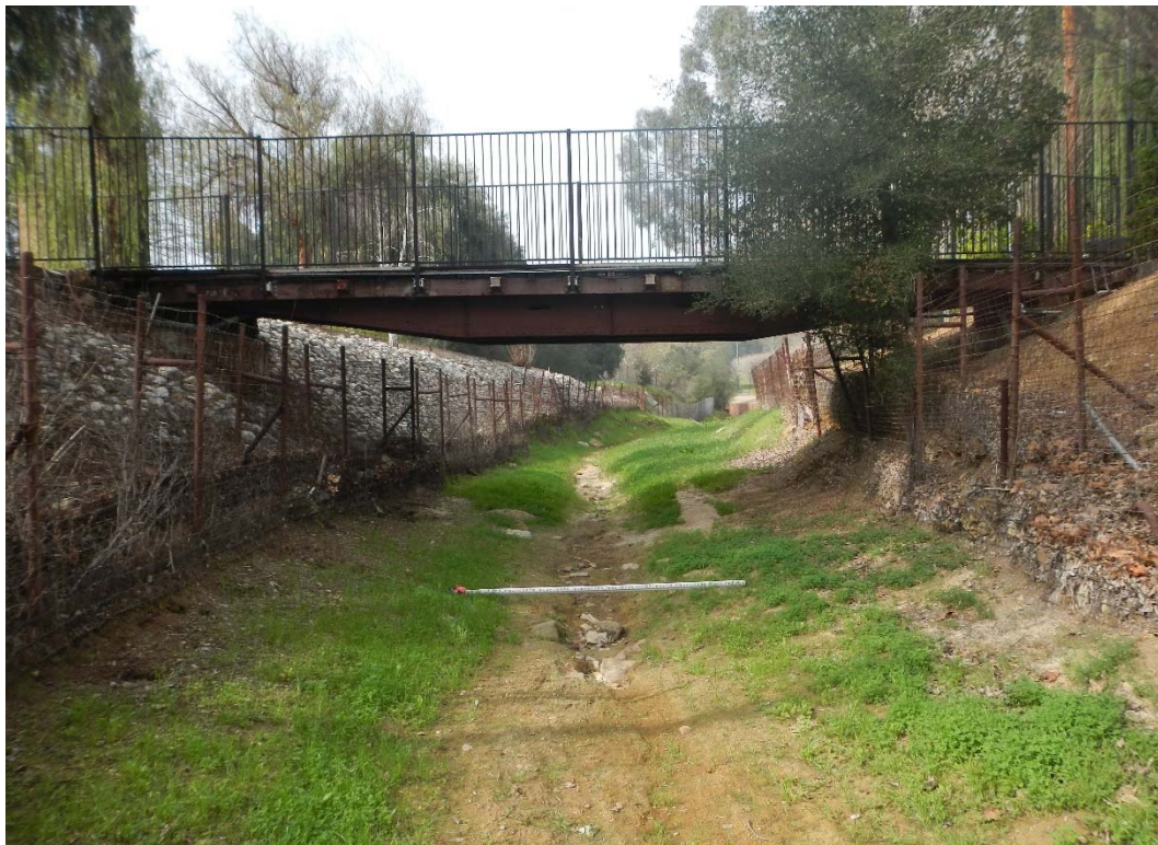
HEC-RAS RIVER STATION 21+54, DOWNSTREAM DIRECTION (PRIVATE DRIVEWAY BRIDGE)
