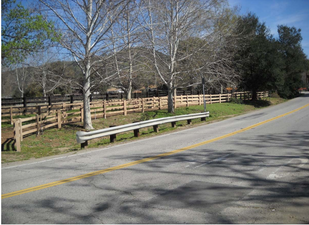
DOWNSTREAM REACH EXTENT, HEC-RAS RIVER STATION 10+04, LEFT OVERBANK
