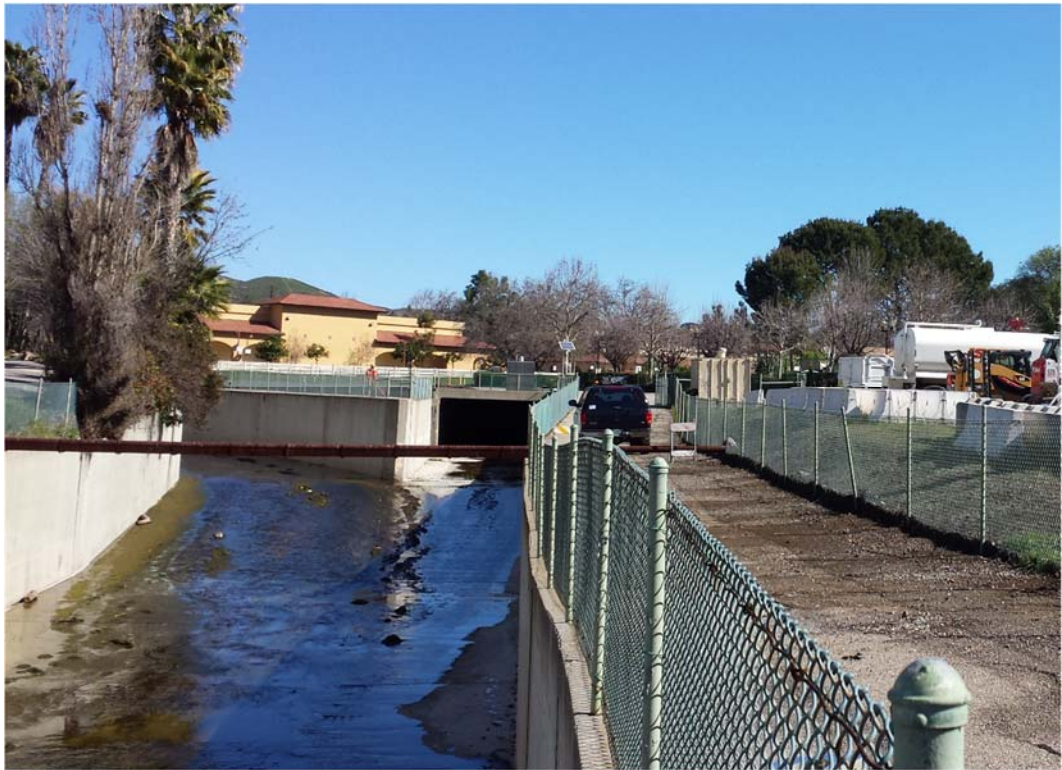
HEC-RAS RIVER STATION 11+39, UPSTREAM DIRECTION
