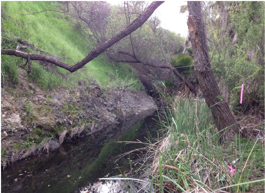
HEC-RAS RIVER STATION 7+38, UPSTREAM DIRECTION
