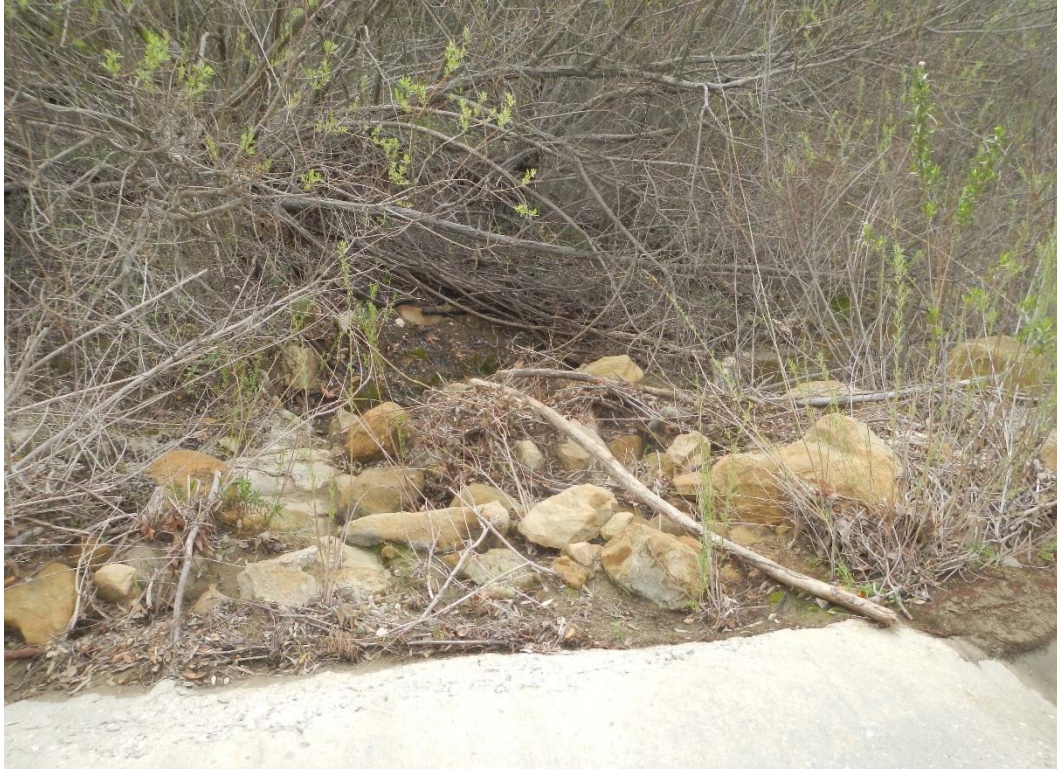
HEC-RAS RIVER STATION 33+47, DOWNSTREAM DIRECTION
