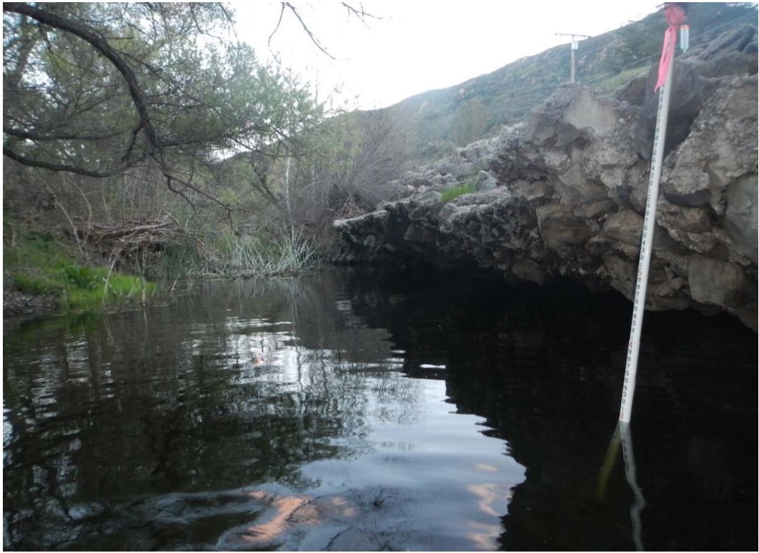
HEC-RAS RIVER STATION 15+39, DOWNSTREAM DIRECTION
