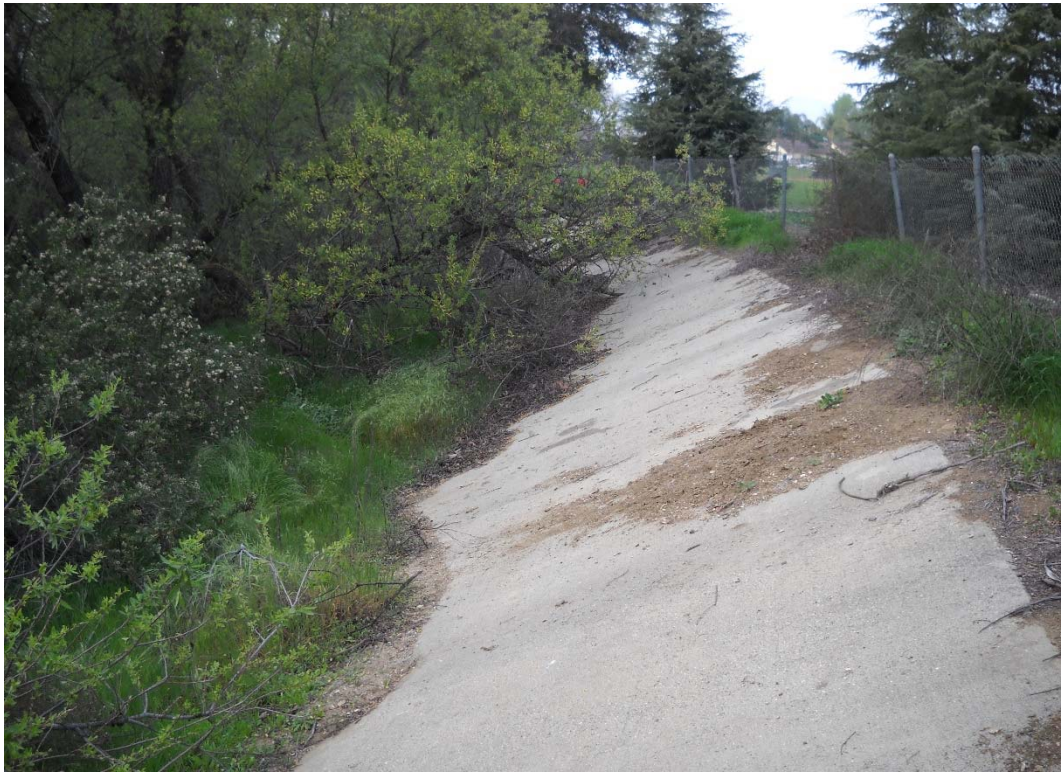
HEC-RAS RIVER STATION 35+52, LEFT BANK, UPSTREAM DIRECTION
