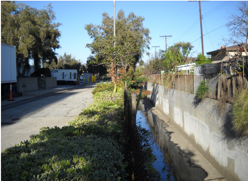
HEC-RAS RIVER STATION 13+50, UPSTREAM DIRECTION
