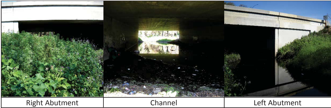
Figure 2-2. Artesia Blvd Bridge
