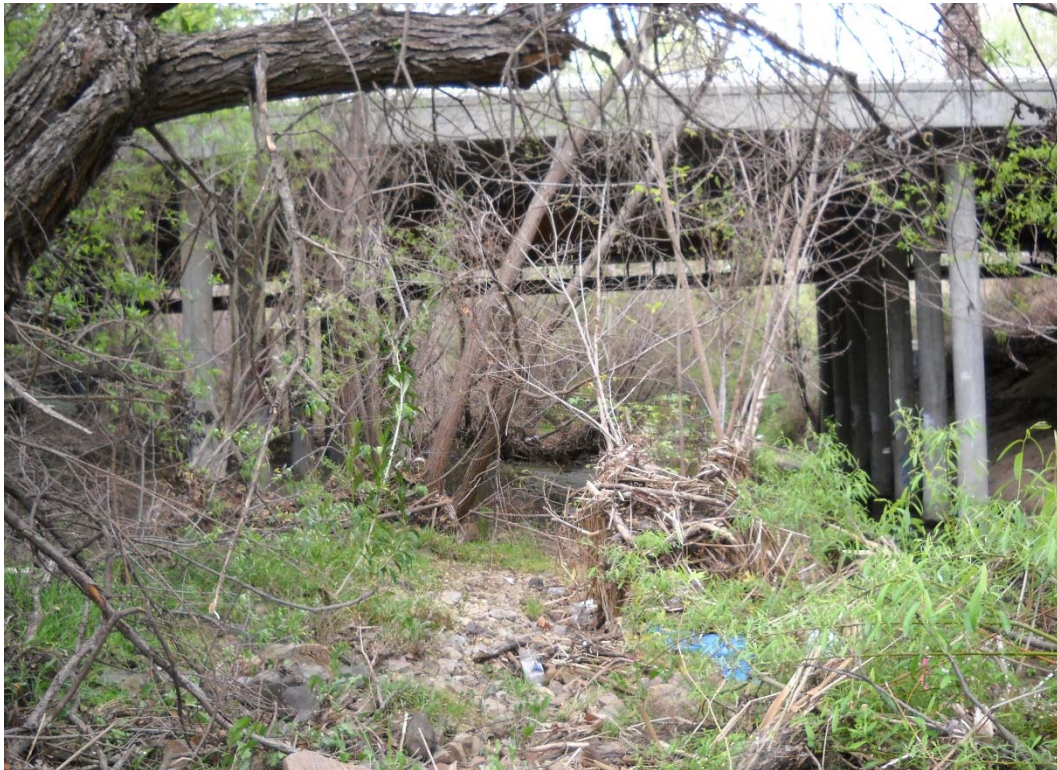
HEC-RAS RIVER STATION 32+96, DOWNSTREAM DIRECTION (OAK CREEK LN. BRIDGE)
