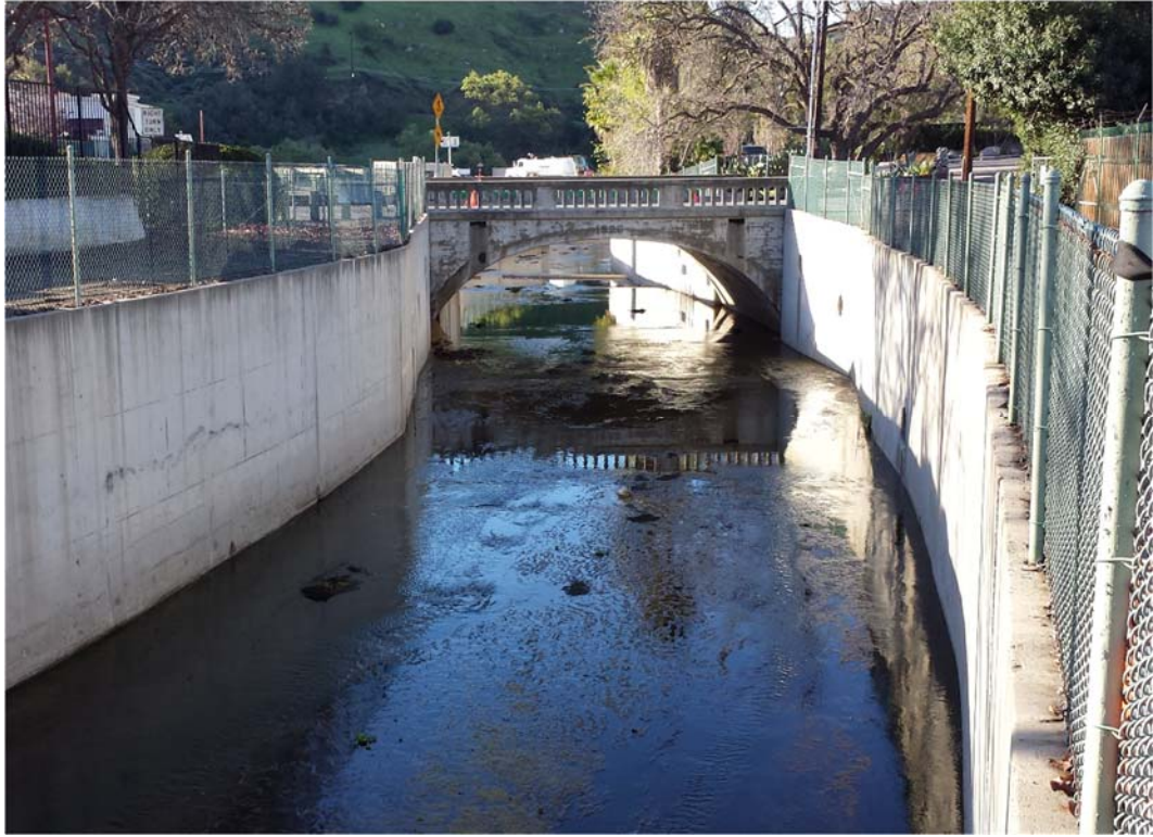
HEC-RAS RIVER STATION 17+34, DOWNSTREAM DIRECTION (AGOURA RD. BRIDGE)
