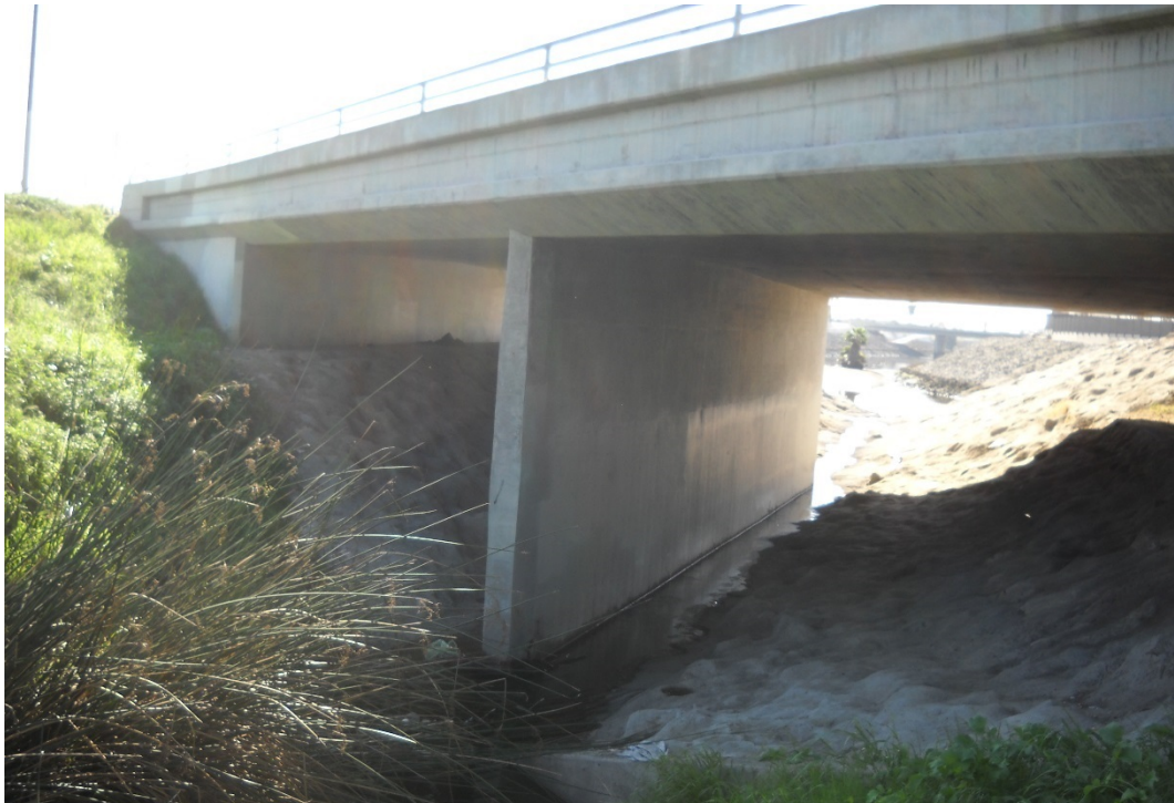
REACH DOWNSTREAM EXTENT, HEC-RAS RIVER STATION 2+21, DOWNSTREAM DIRECTION
