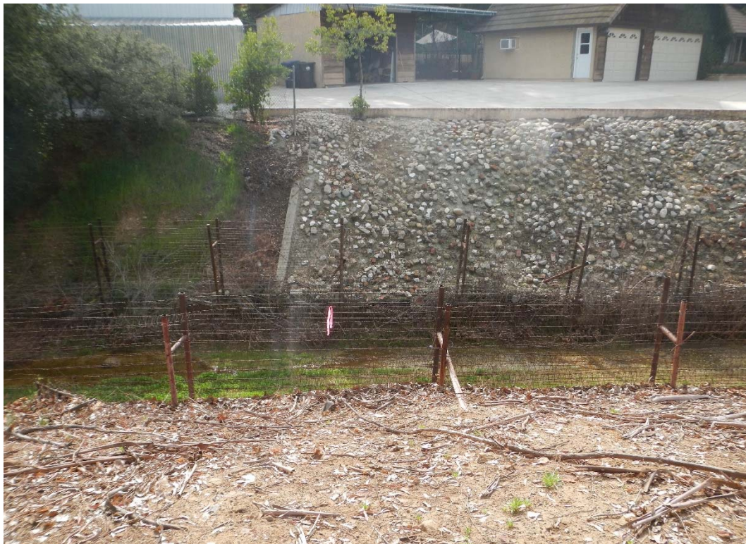
92 FT. UPSTREAM OF HEC-RAS RIVER STATION 22+78, LEFT BANK
