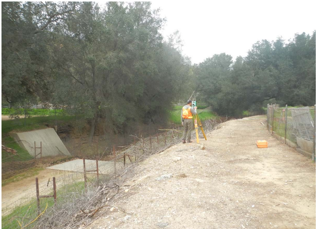
HEC-RAS RIVER STATION 12+33, DOWNSTREAM DIRECTION
