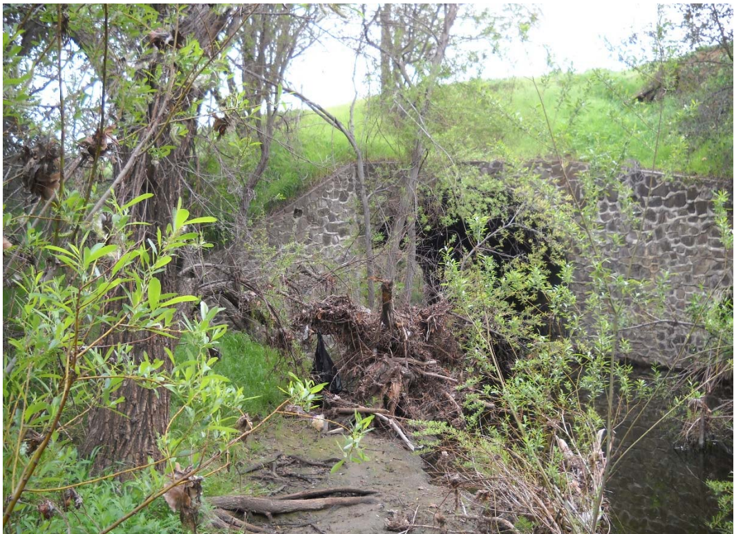
HEC-RAS RIVER STATION 0+78, DOWNSTREAM DIRECTION
