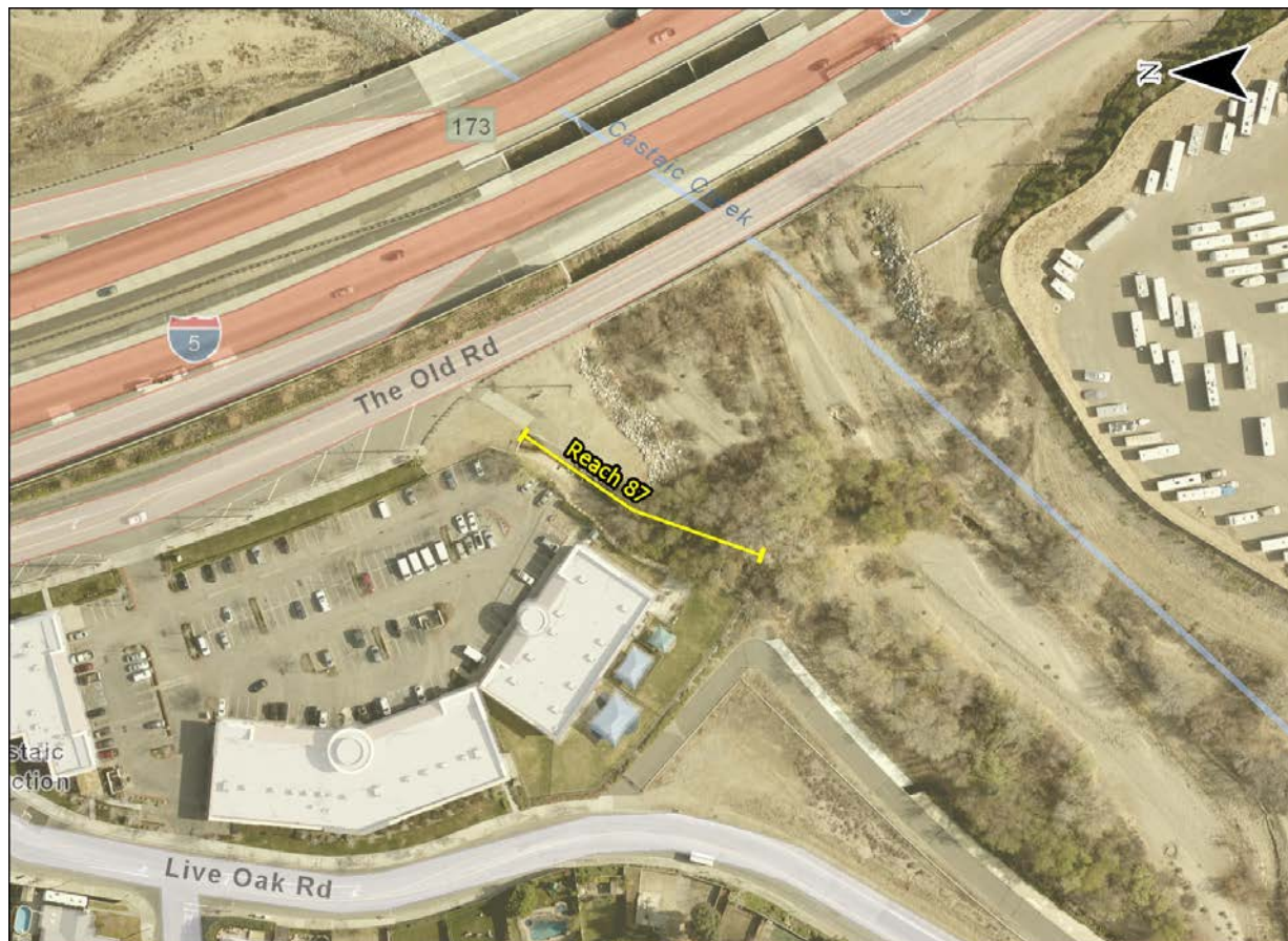
Figure 15-1: Reach 87 – Castaic Old Road Drain Outlet
