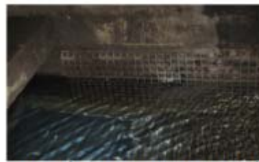
Low-Flow Diversion Dam and Inlet in a Storm Drain
