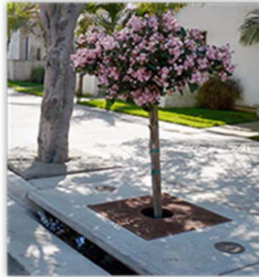
Curb Inlet Biofilter
