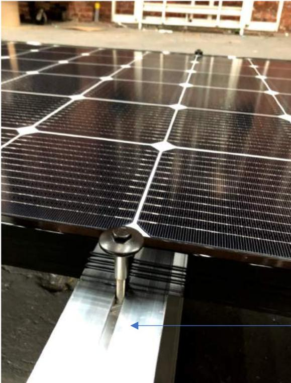
Ensure T-bolt fully engages with rail channel
