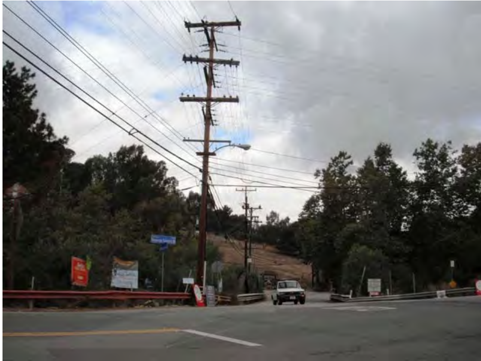
Figure 2-5 Existing Overhead Utility Lines Facing West at the Intersection of Old Topanga Canyon Road and Topanga Canyon Boulevard
