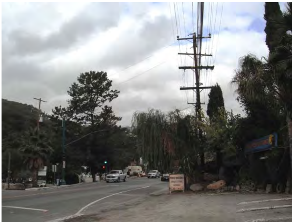
Figure 2-6 Existing Overhead Utility Lines Looking North From S. Topanga Canyon Boulevard
