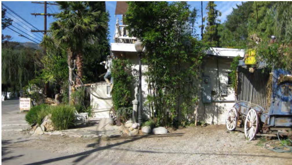
Plate 5. Hidden Treasures business building. View to west.
