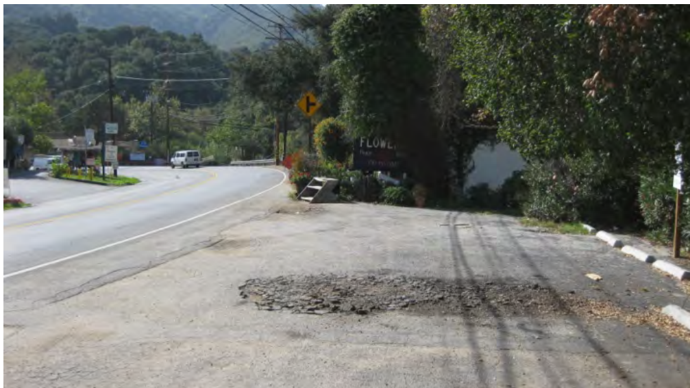
Plate 30. Parking lot next to flower shop. View to west.
