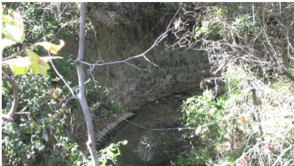
Plate 24. Concrete and cobble lined reinforcement of Topanga Canyon Boulevard side wall. View to northwest.
