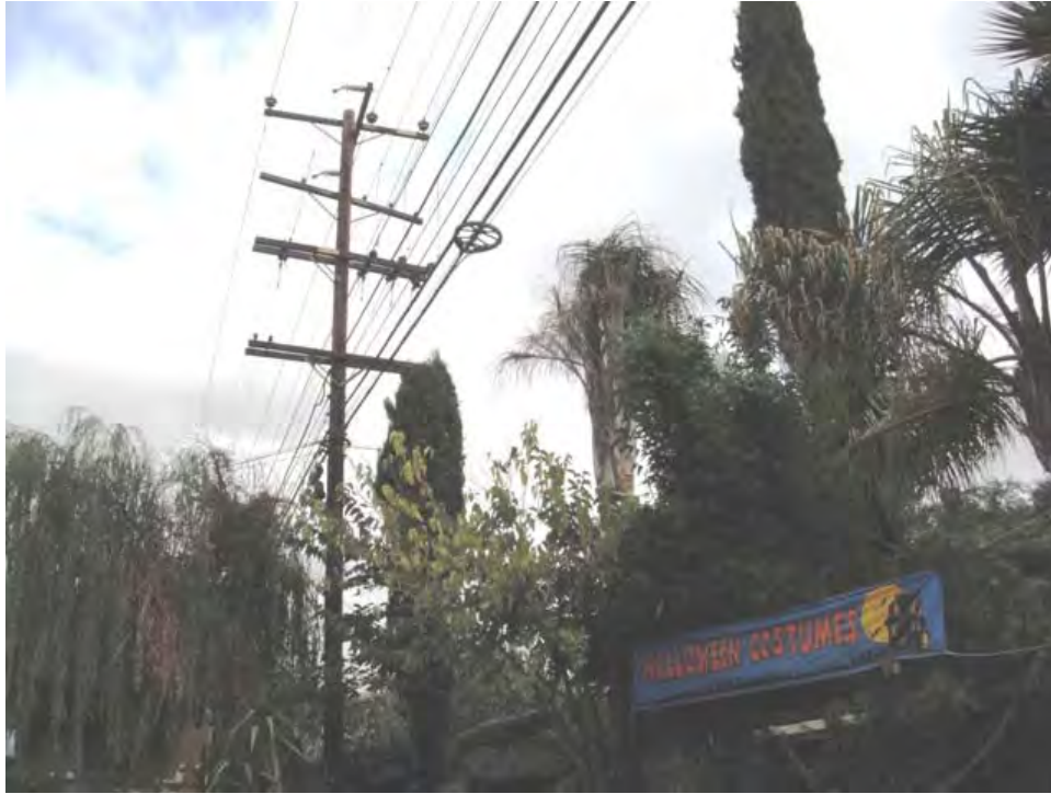
Figure 2-7 Existing Overhead Utility Lines and Trees Fronting Retail Store at the Intersection of South Topanga Canyon Boulevard and Cuesta Cala Road
