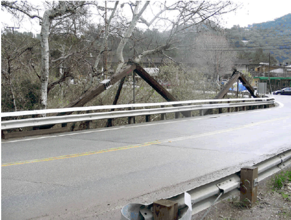
Plate 31. Topanga Canyon Creek Bridge (53C0939). View to northeast.
