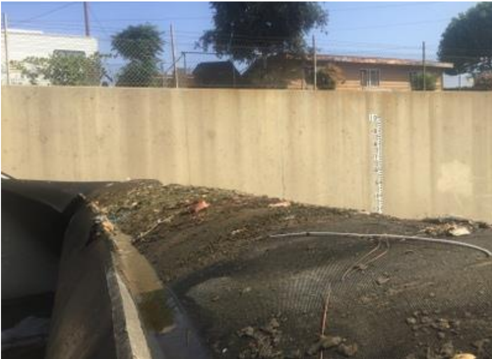
PHOTO 6 INFLATED RUBBER DAM TOP VIEW LEFT ABUTMENT
