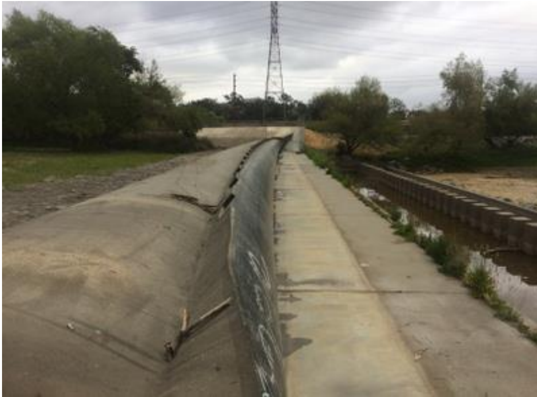
PHOTO 5 INFLATED RUBBER DAM UNDER FIN RIGHT ABUTMENT
