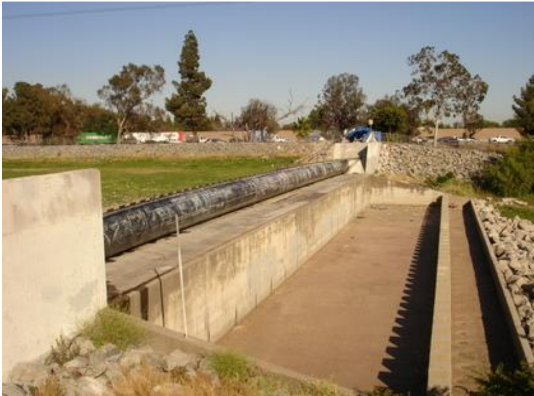
PHOTO 2 INFLATED RUBBER DAM DOWNSTREAM VIEW (2017)
