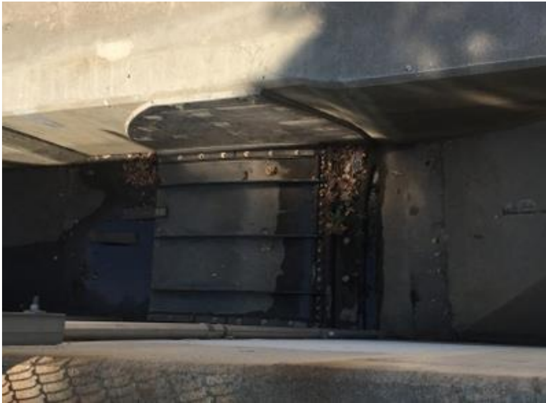
PHOTO 1 DEFLATED RUBBER DAM UPSTREAM VIEW
