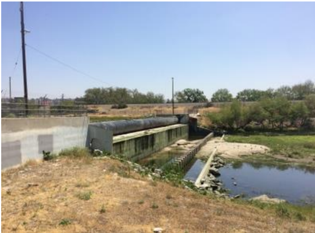
PHOTO 2 INFLATED RUBBER DAM DOWNSTREAM VIEW
