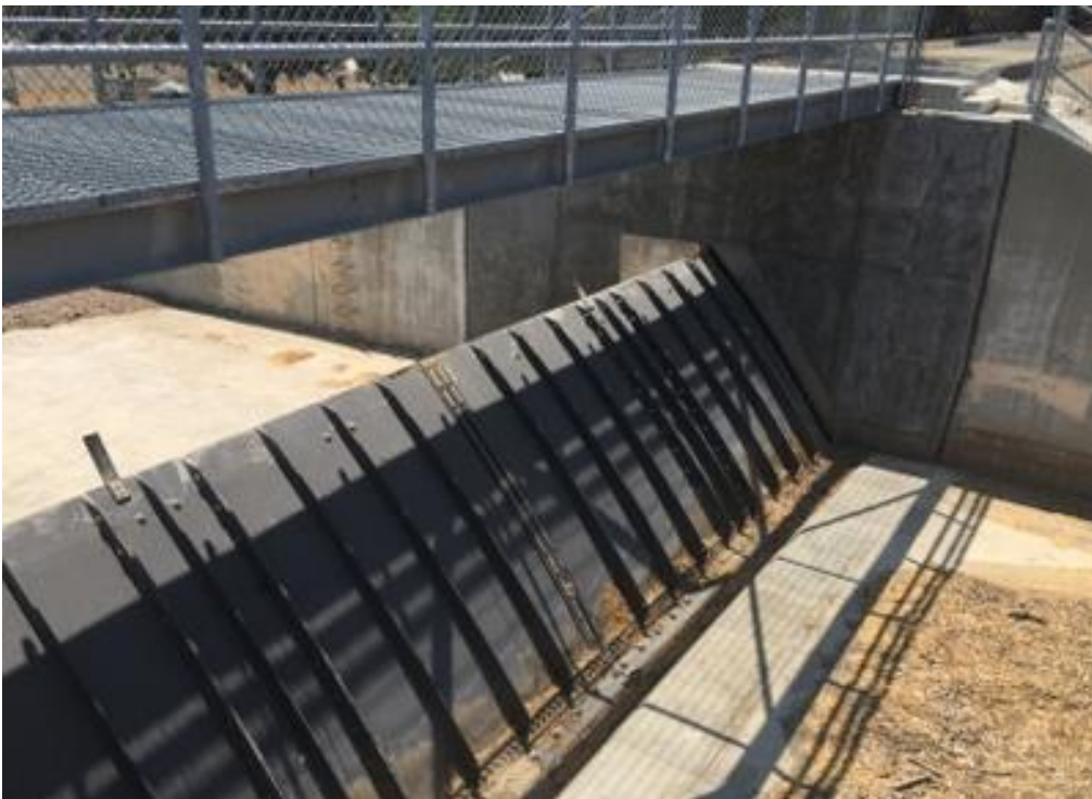
INFLATED RUBBER DAM DOWNSTREAM VIEW
