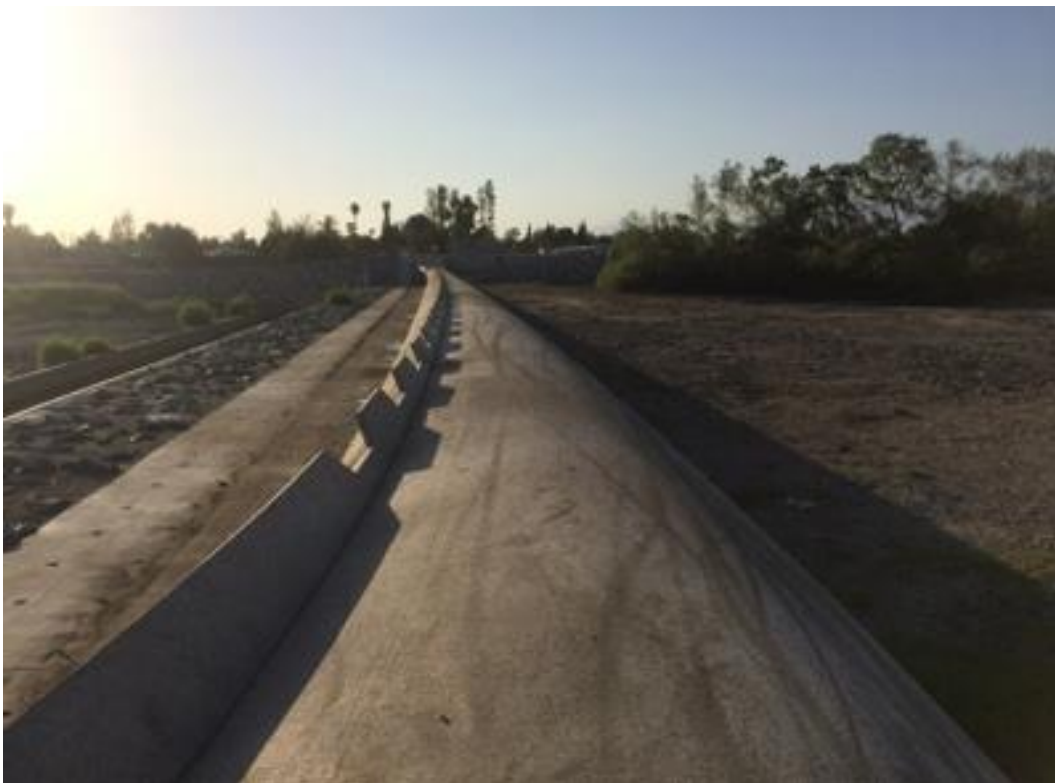
INFLATED RUBBER DAM TOP VIEW LEFT ABUTMENT
