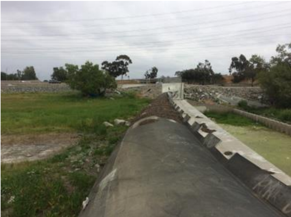
PHOTO 6 INFLATED RUBBER DAM TOP VIEW RIGHT ABUTMENT
