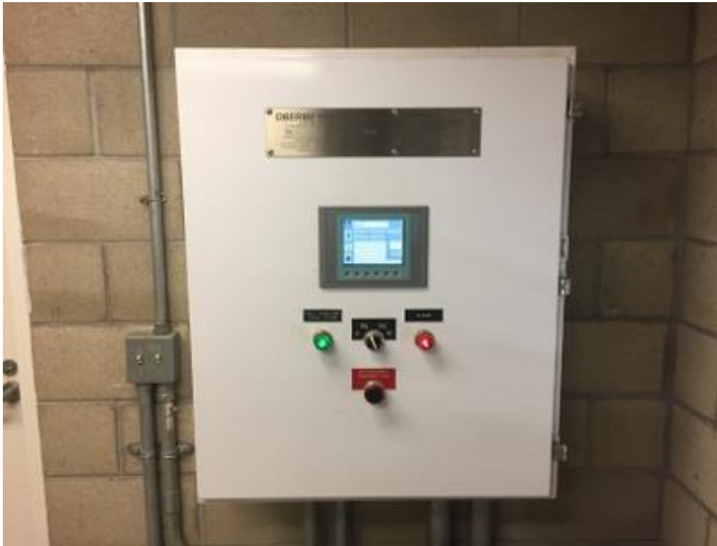
PLC CONTROL PANEL EXTERIOR VIEW
