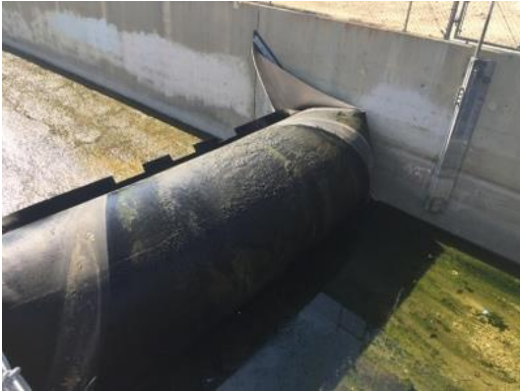
PHOTO 2 INFLATED RUBBER DAM DOWNSTREAM VIEW
