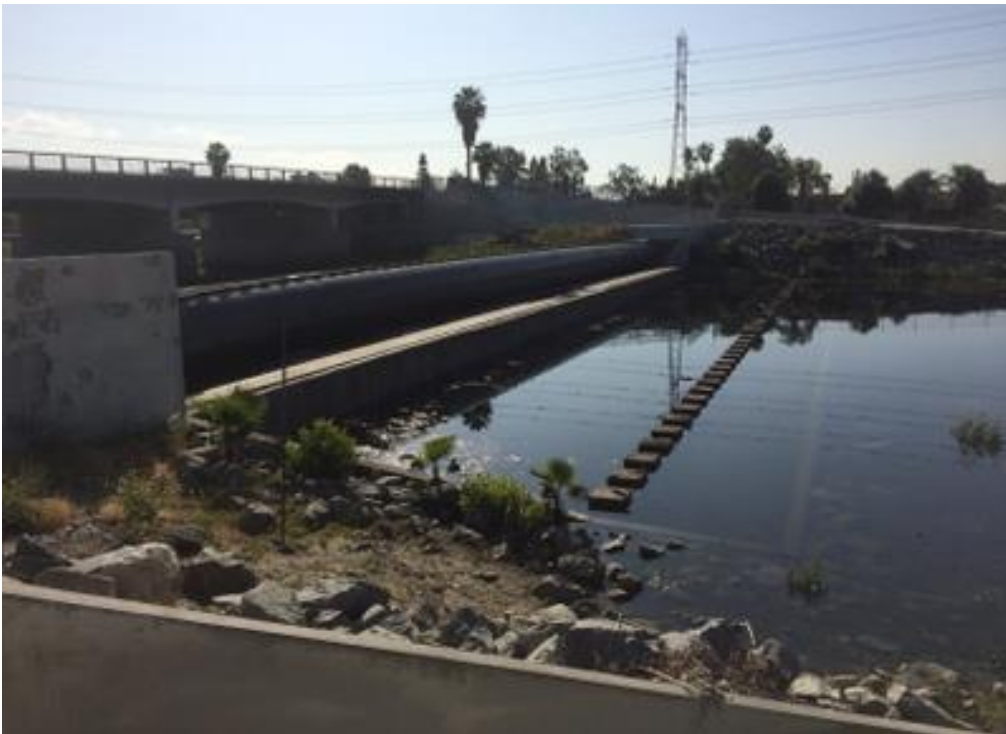
PHOTO 4 INFLATED RUBBER DAM DOWNSTREAM VIEW
