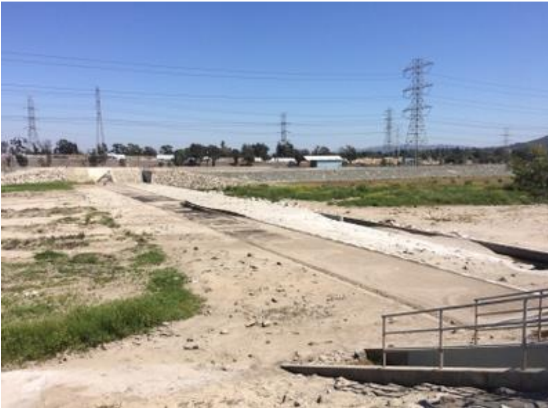
PHOTO 1 DEFLATED RUBBER DAM UPSTREAM VIEW
