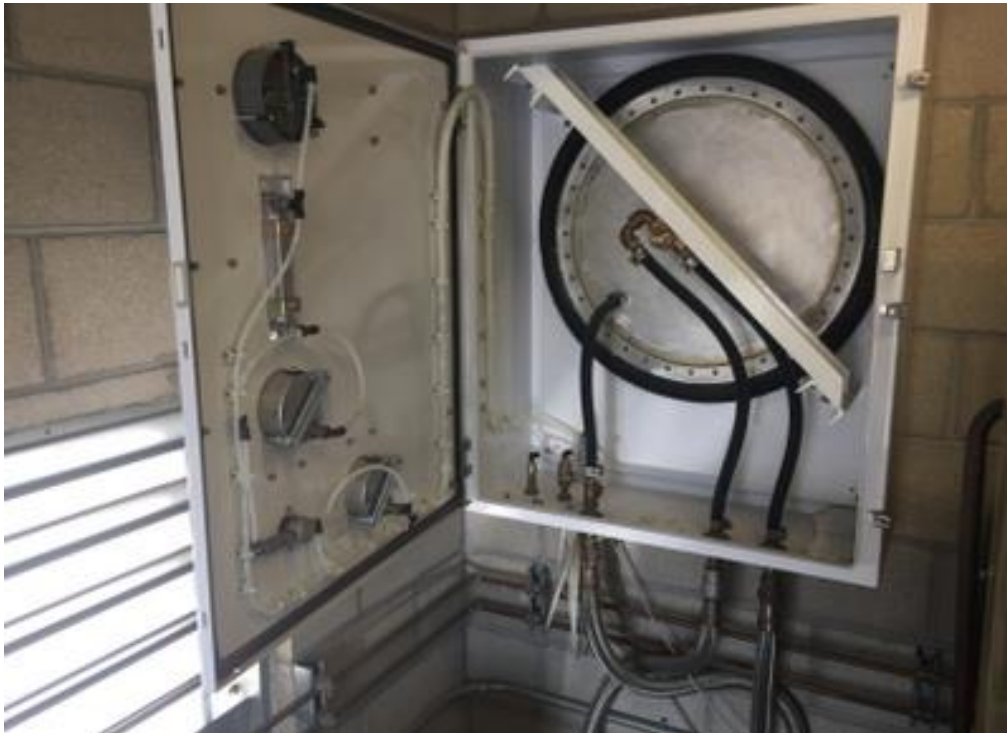
PRESSURE RELIEF PANEL INTERIOR
