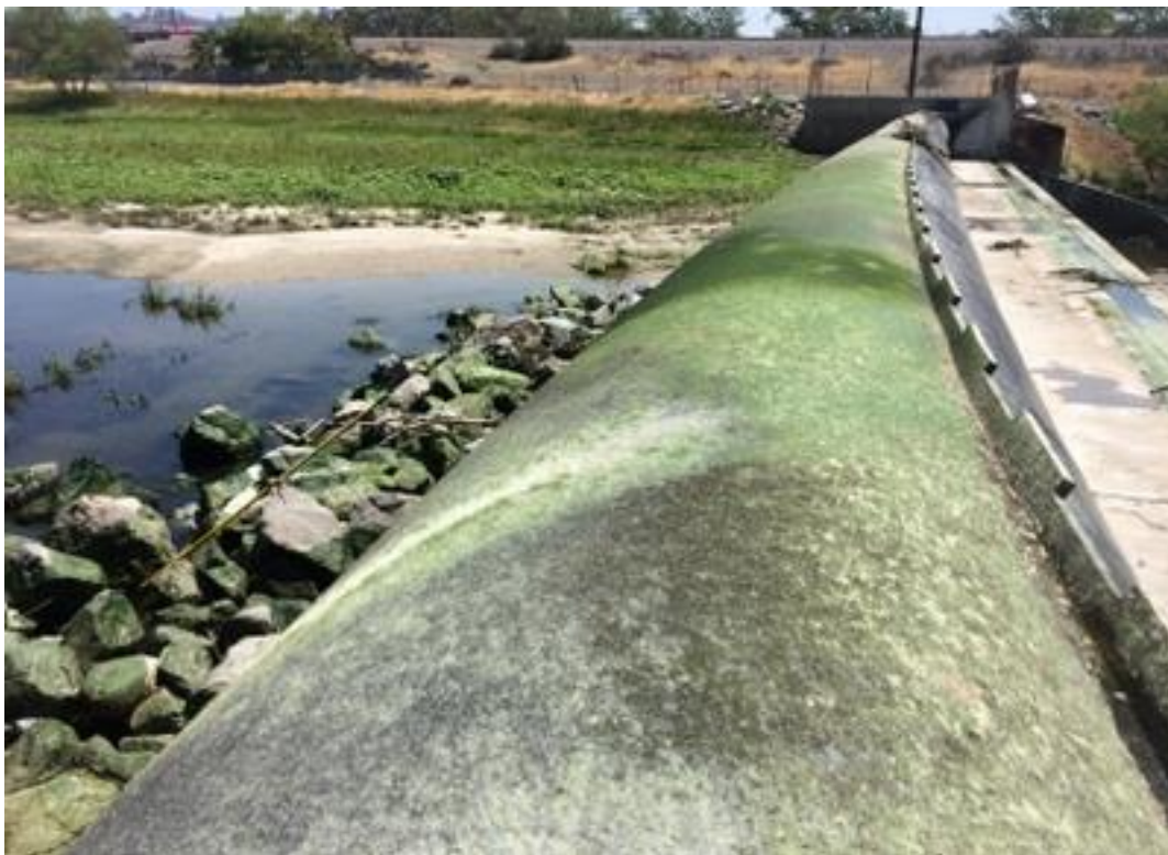
PHOTO 4 INFLATED RUBBER DAM TOP VIEW RIGHT ABUTMENT
