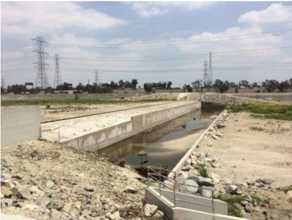
PHOTO 2 DEFLATED RUBBER DAM DOWNSTREAM VIEW
