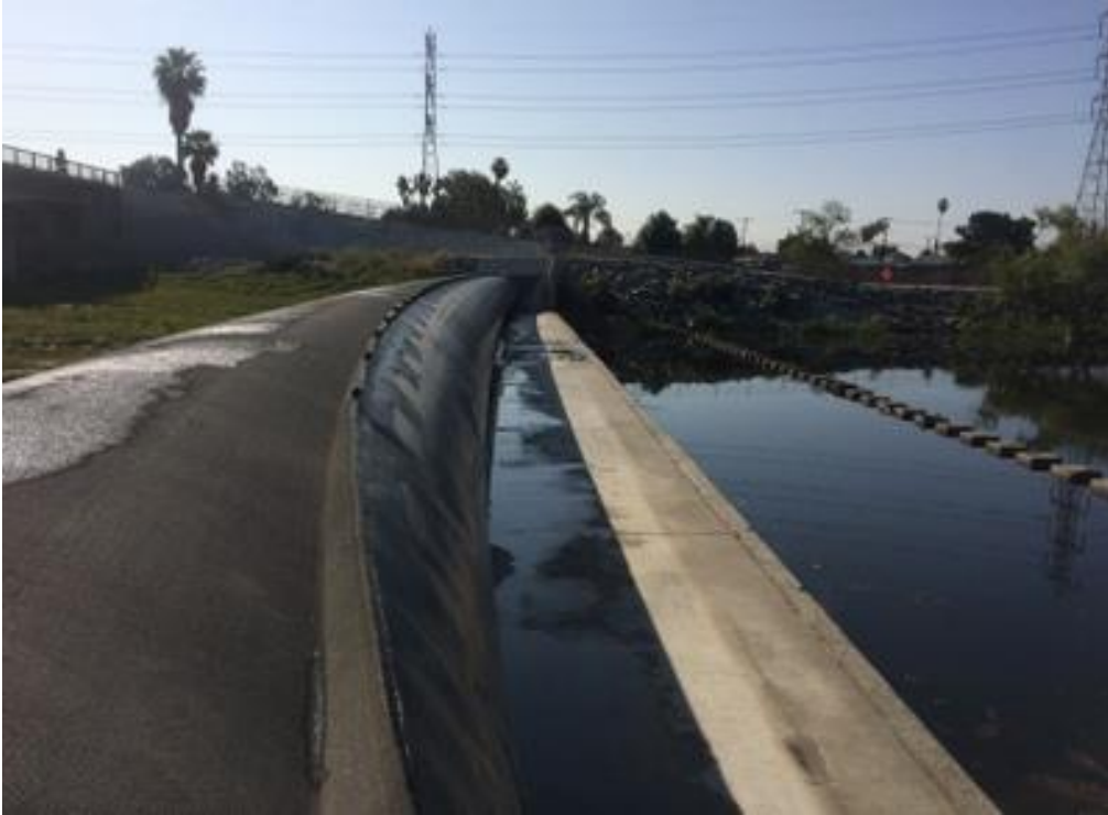
PHOTO 5 INFLATED RUBBER DAM UNDER FIN RIGHT ABUTMENT
