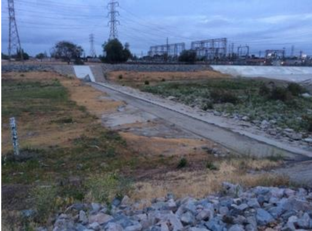
PHOTO 1 DEFLATED RUBBER DAM UPSTREAM VIEW
