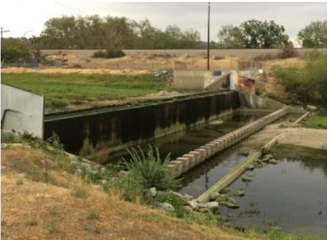
DEFLATED RUBBER DAM DOWNSTREAM VIEW
