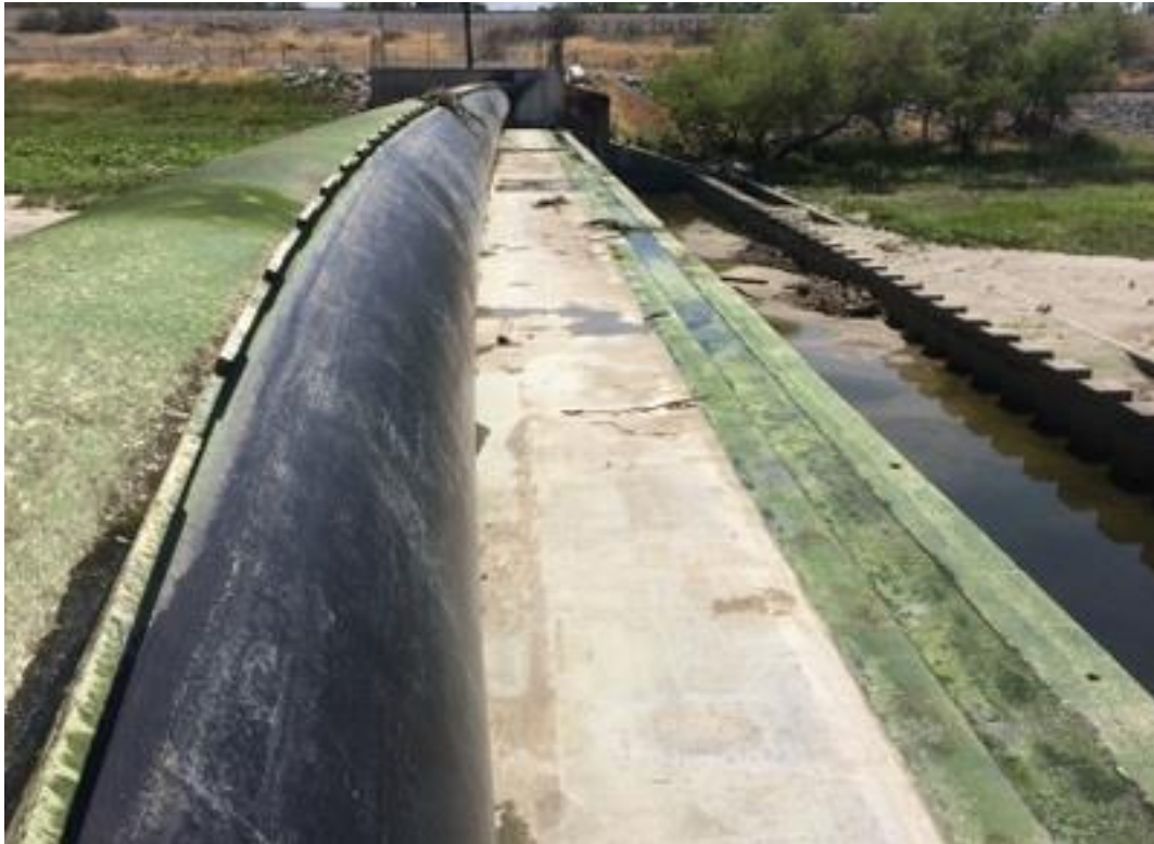
PHOTO 3 INFLATED RUBBER DAM UNDER FIN RIGHT ABUTMENT
