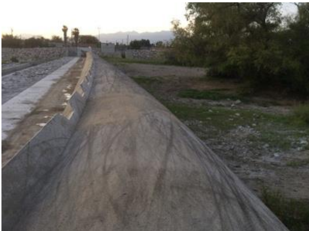
PHOTO 8 INFLATED RUBBER DAM TOP VIEW LEFT ABUTMENT
