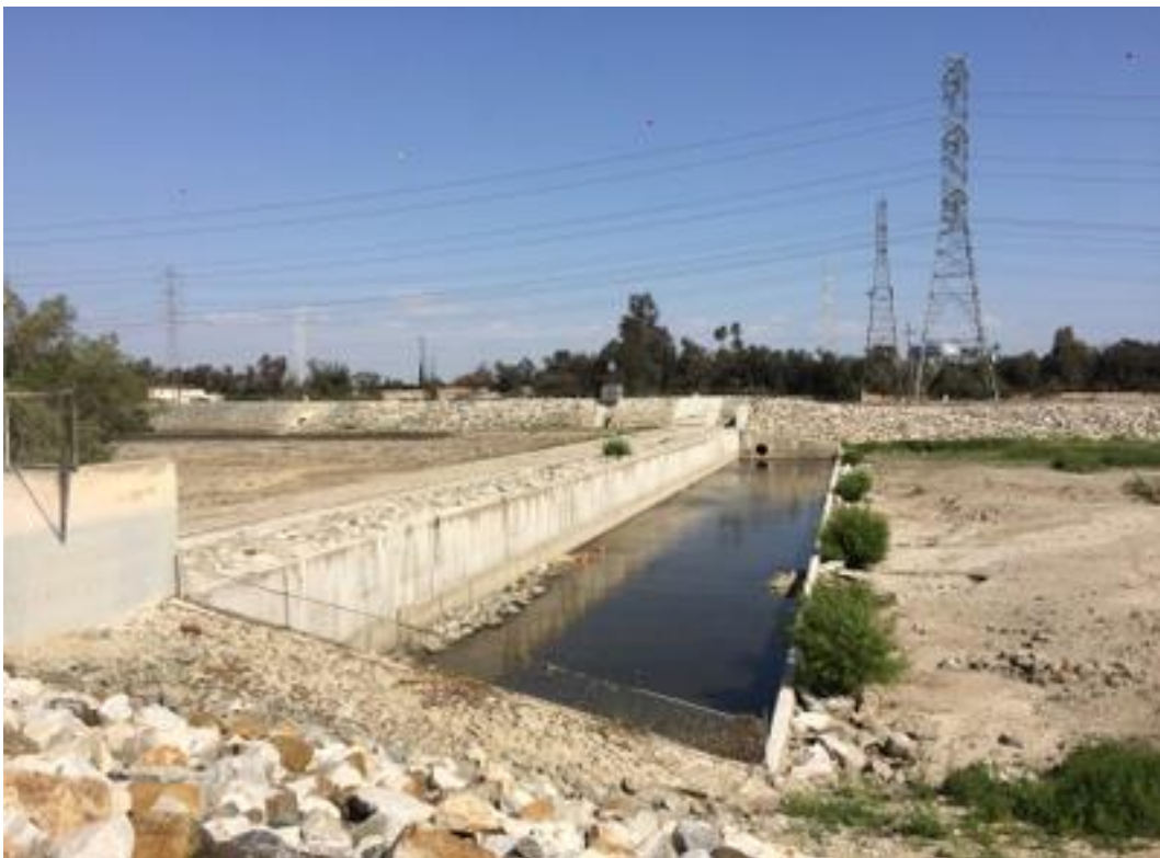
DEFLATED RUBBER DAM DOWNSTREAM VIEW
