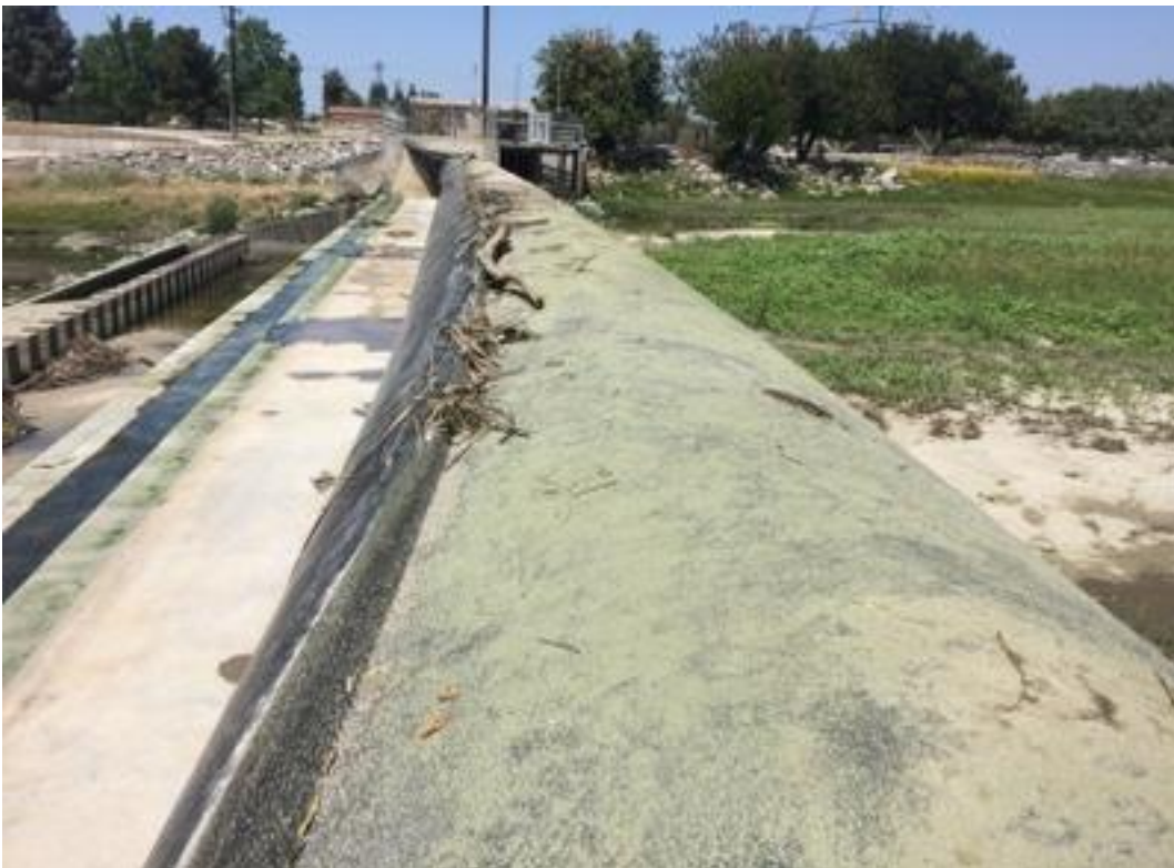
PHOTO 6 INFLATED RUBBER TOP VIEW LEFT ABUTMENT
