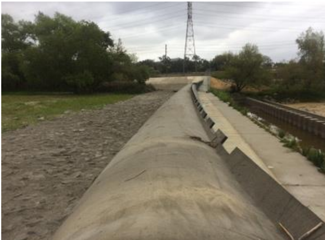
PHOTO 6 INFLATED RUBBER DAM TOP VIEW RIGHT ABUTMENT
