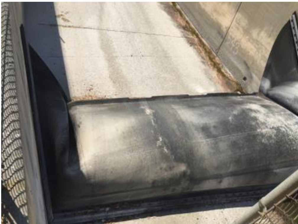
PHOTO 6 INFLATED RUBBER DAM TOP VIEW LEFT ABUTMENT
