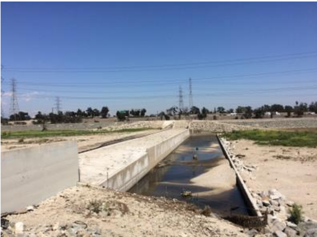
PHOTO 2 DEFLATED RUBBER DAM DOWNSTREAM VIEW
