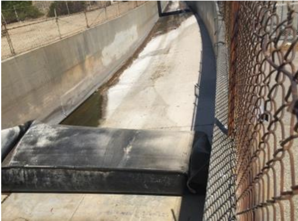
PHOTO 5 INFLATED RUBBER DAM UNDER FIN LEFT ABUTMENT
