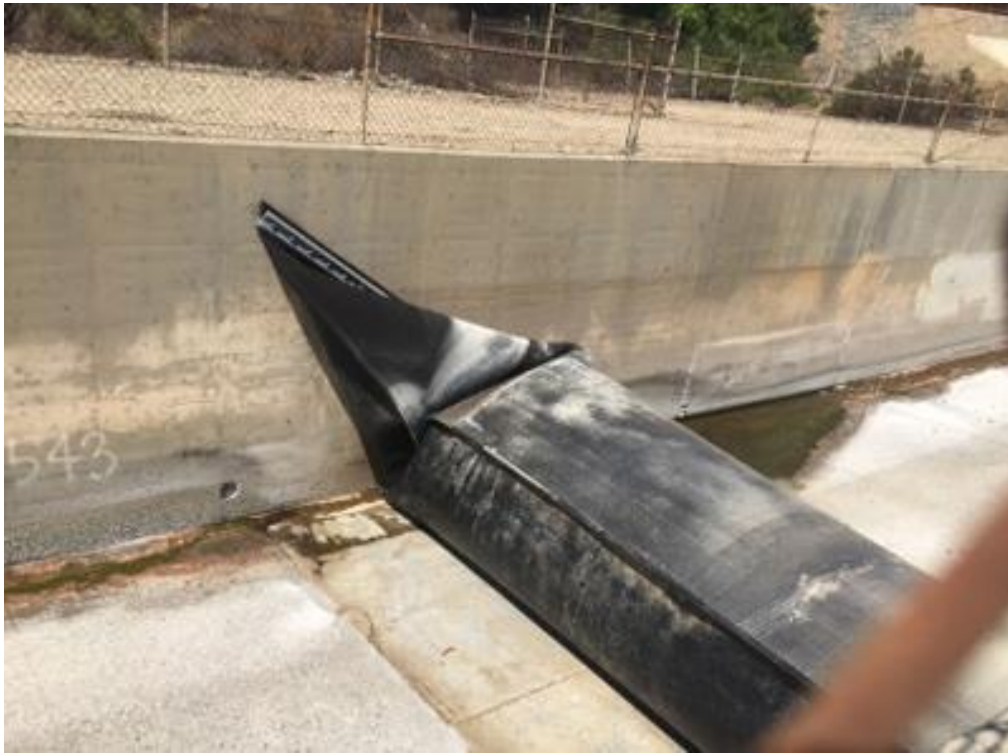
PHOTO 4 INFLATED RUBBER DAM TOP VIEW RIGHT ABUTMENT
