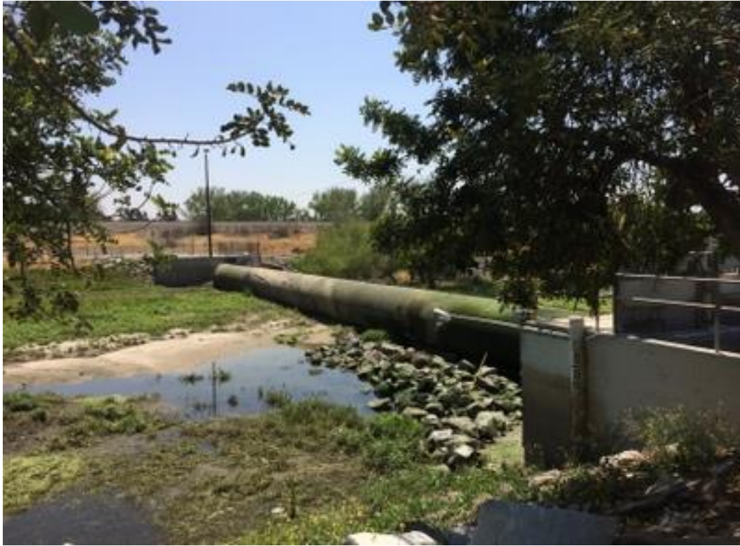
PHOTO 1 INFLATED RUBBER DAM UPSTREAM VIEW
