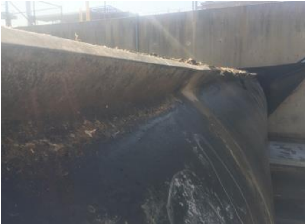
INFLATED RUBBER DAM UNDER FIN RIGHT ABUTMENT
