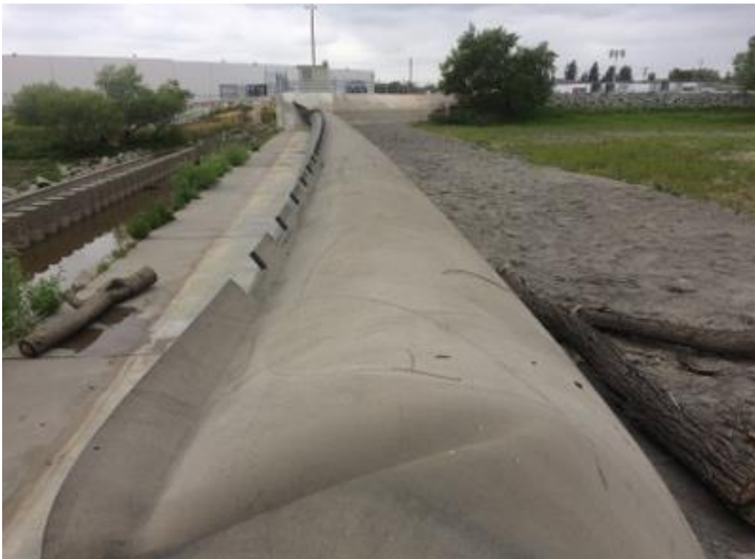
INFLATED RUBBER DAM TOP VIEW LEFT ABUTMENT
