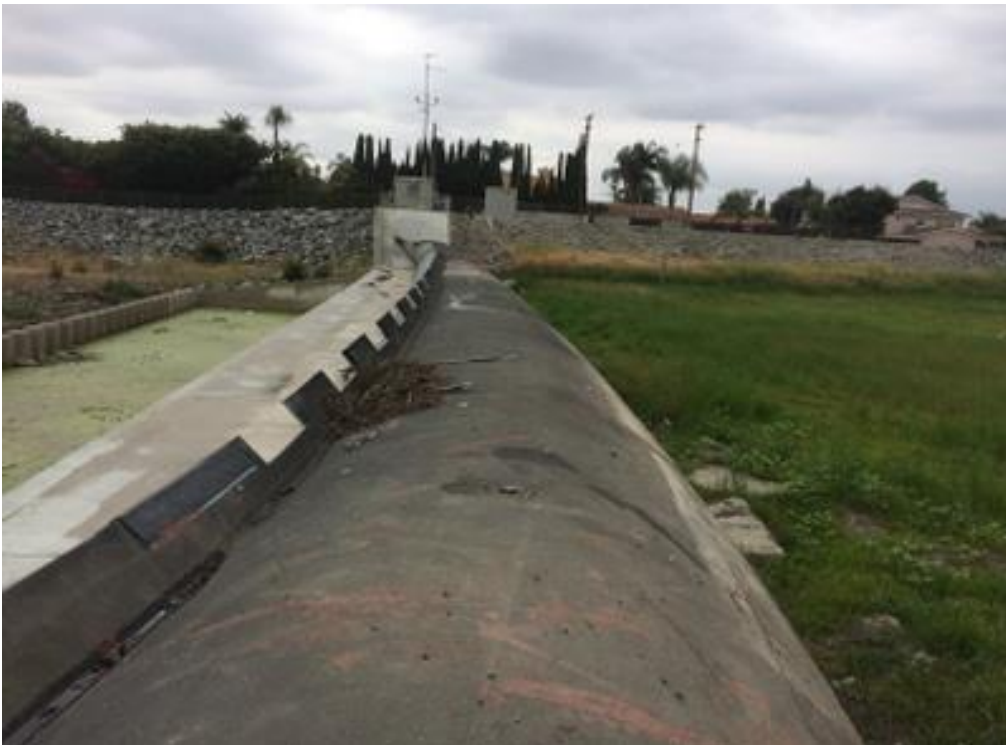
PHOTO 8 INFLATED RUBBER DAM TOP VIEW LEFT ABUTMENT
