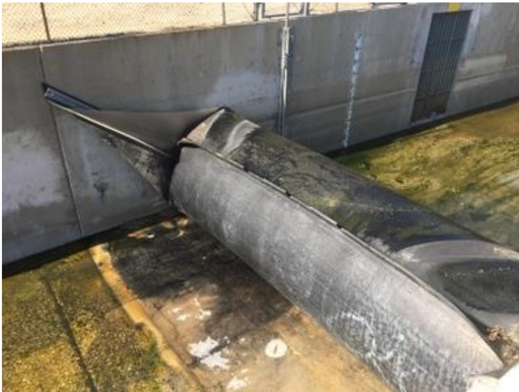
PHOTO 6 INFLATED RUBBER DAM TOP VIEW LEFT ABUTMENT
