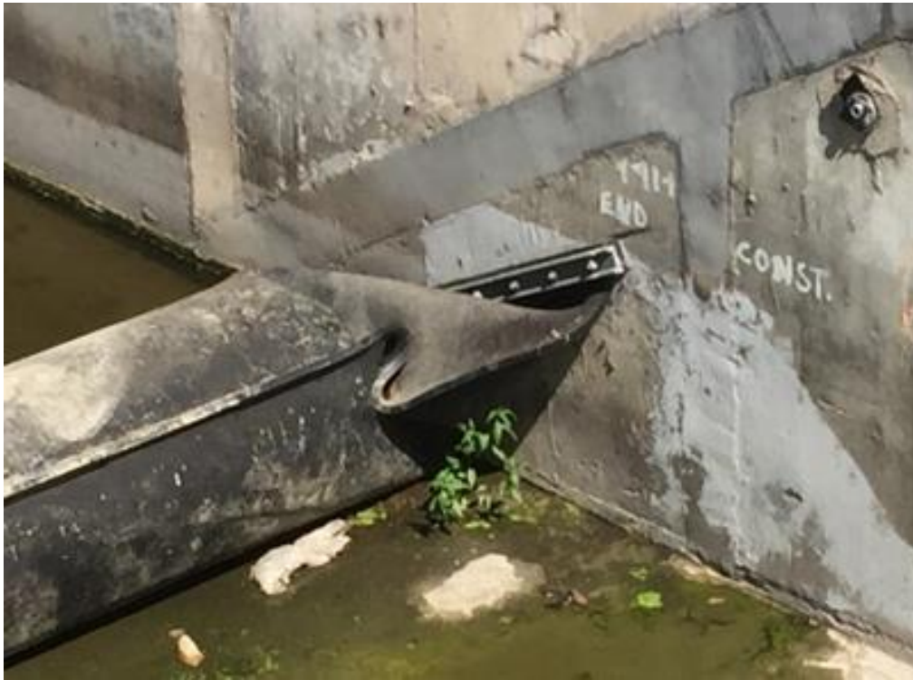
INFLATED RUBBER DAM UNDER FIN LEFT ABUTMENT
