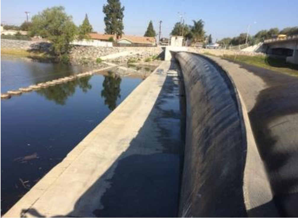
PHOTO 7 INFLATED RUBBER DAM UNDER FIN LEFT ABUTMENT
