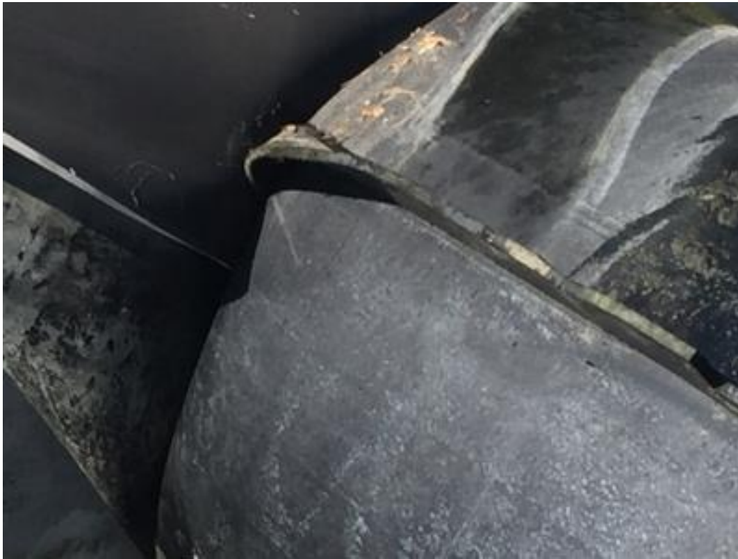
INFLATED RUBBER DAM UNDER FIN RIGHT ABUTMENT
