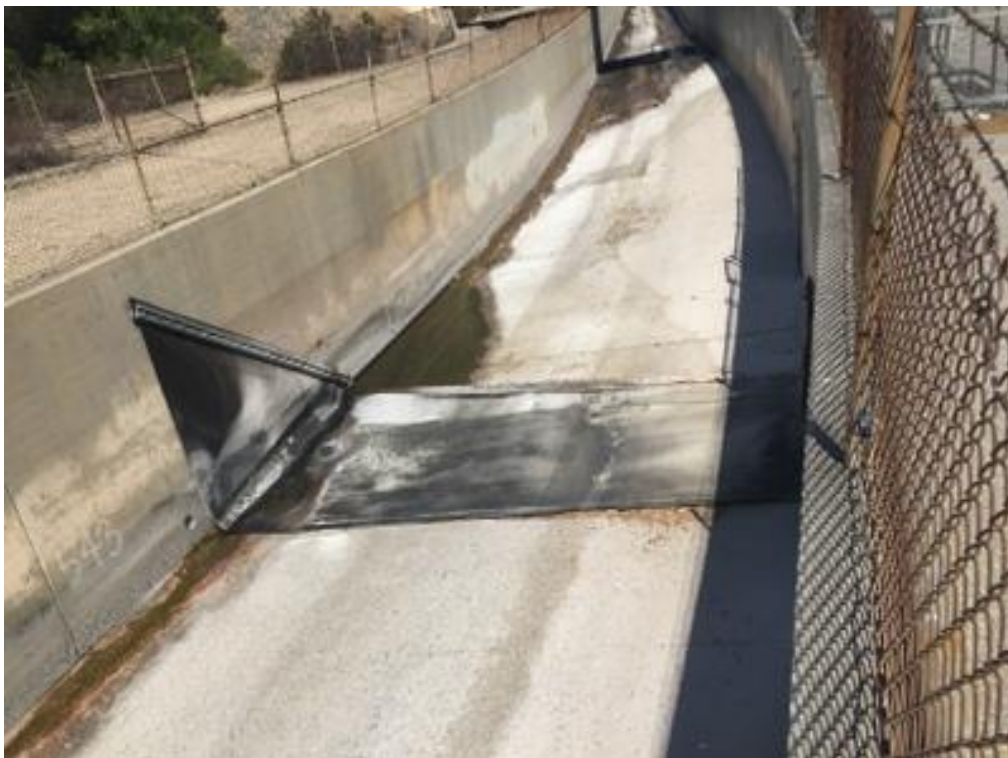
PHOTO 2 DEFLATED RUBBER DAM DOWNSTREAM VIEW
