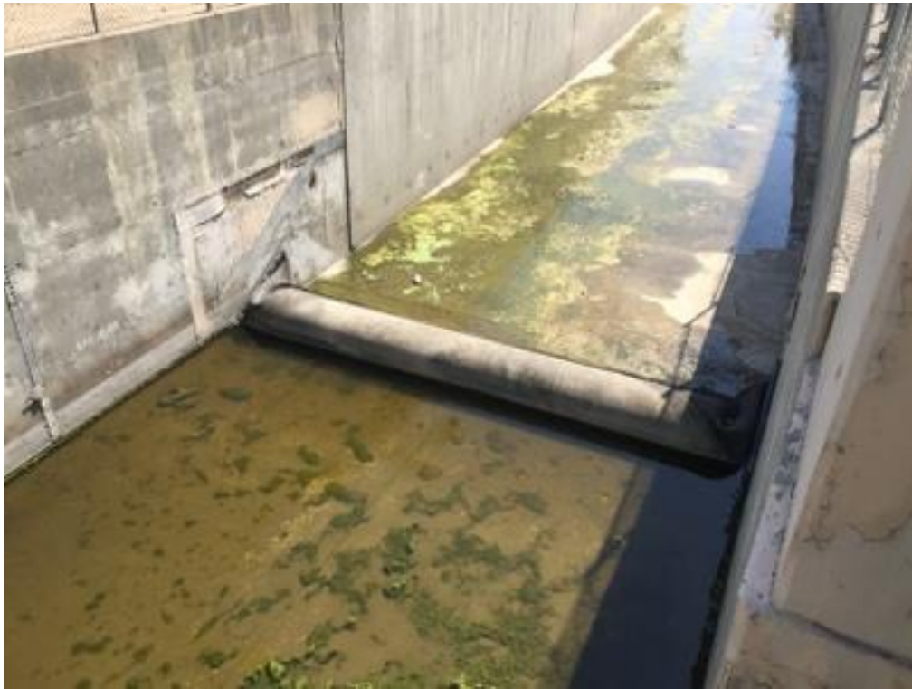
PHOTO 1 INFLATED RUBBER DAM UPSTREAM VIEW
