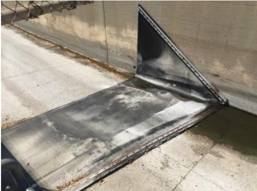
PHOTO 1 DEFLATED RUBBER DAM UPSTREAM VIEW
