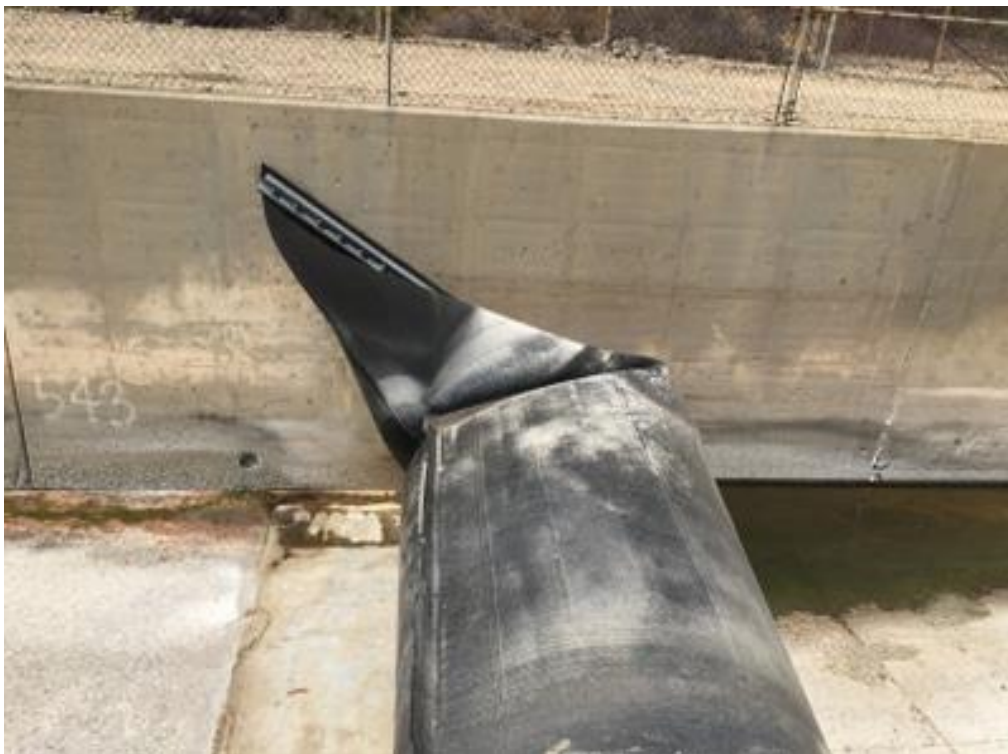
PHOTO 4 INFLATED RUBBER DAM TOP VIEW RIGHT ABUTMENT
