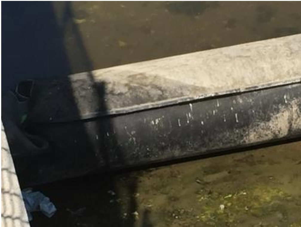
PHOTO 5 INFLATED RUBBER DAM UNDER FIN RIGHT ABUTMENT
