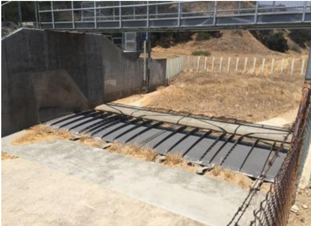
PHOTO 1 DEFLATED RUBBER DAM UPSTREAM VIEW
