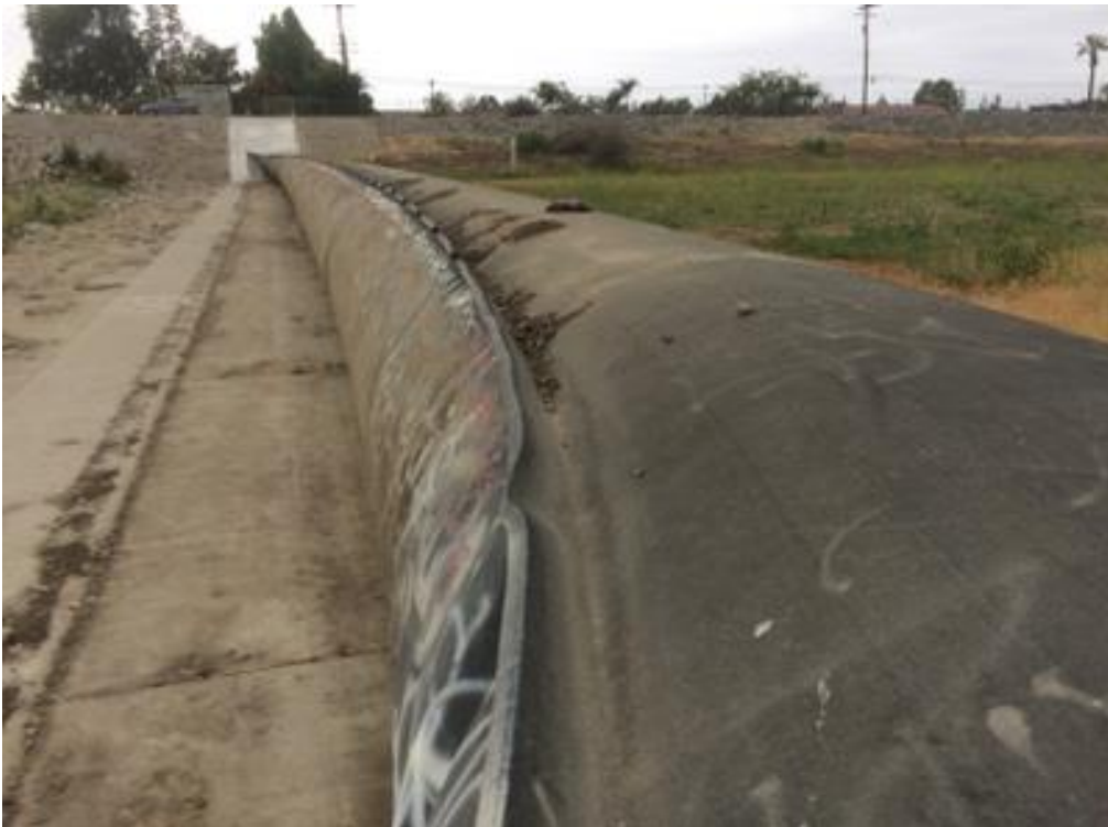
PHOTO 8 INFLATED RUBBER DAM TOP VIEW LEFT ABUTMENT
