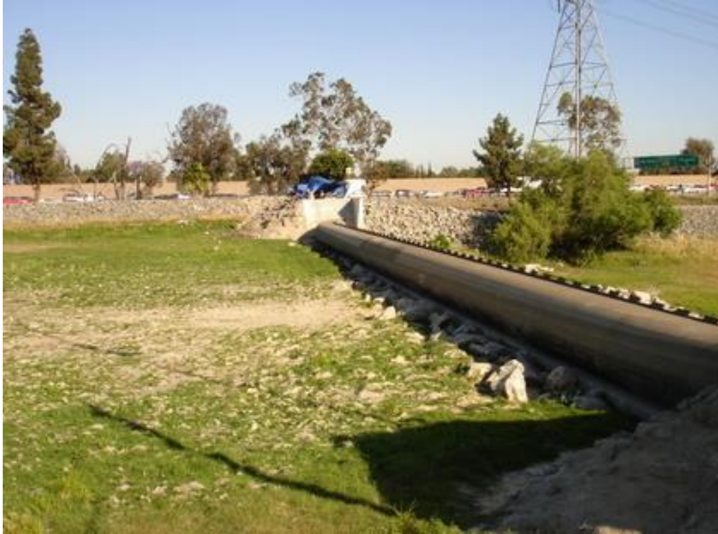
PHOTO 2 INFLATED RUBBER DAM DOWNSTREAM VIEW (2017)
