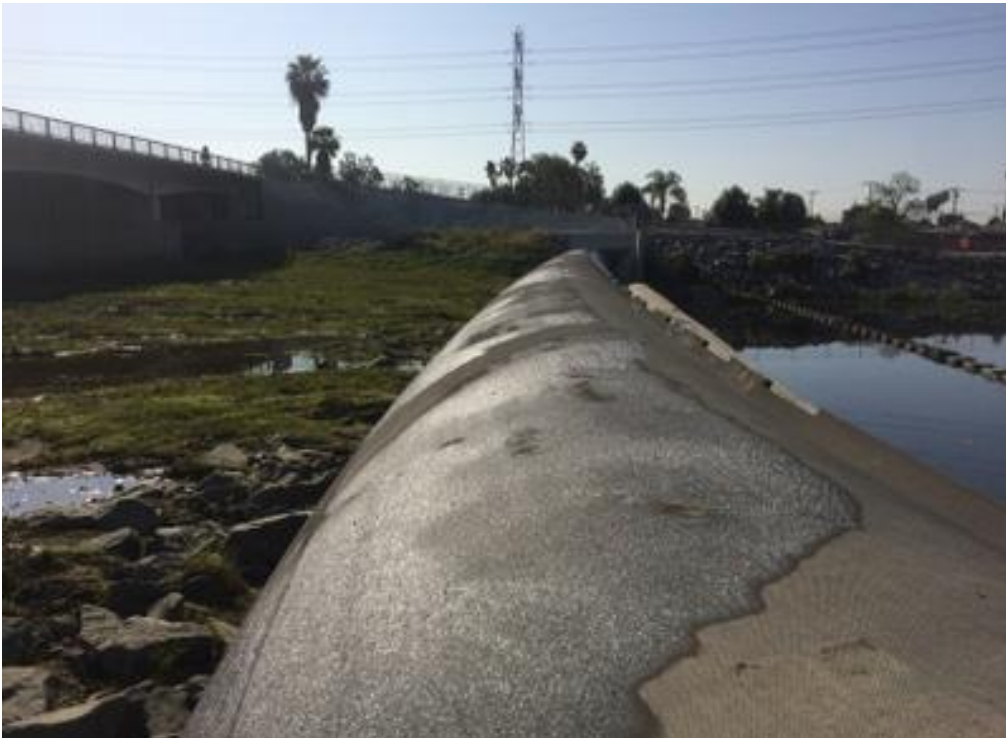
PHOTO 6 INFLATED RUBBER DAM TOP VIEW RIGHT ABUTMENT
