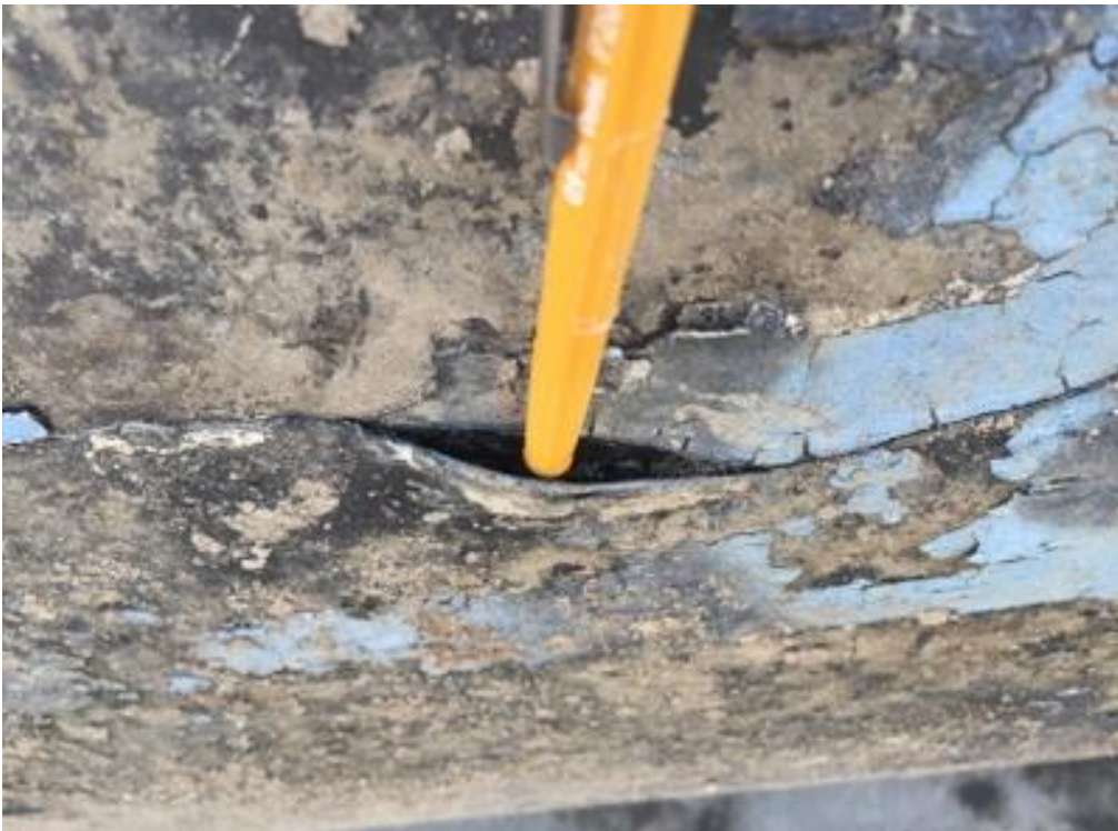
SEAM SEPERATION DOWNSTREAM
