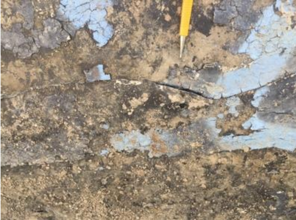
SEAM SEPERATION DOWNSTREAM
