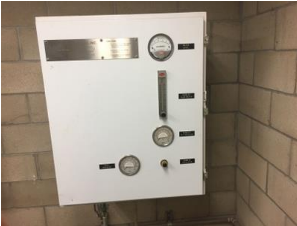
OVERPRESSURE RELIEF CONTROL PANEL EXTERIOR VIEW
