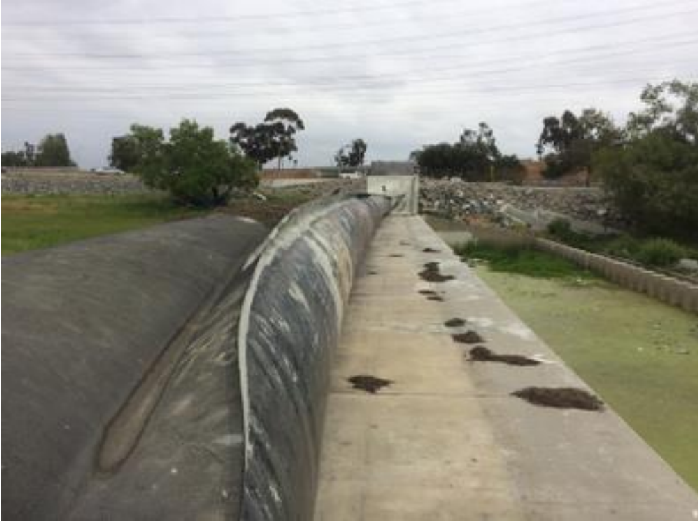
PHOTO 5 INFLATED RUBBER DAM UNDER FIN RIGHT ABUTMENT
