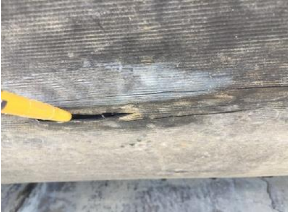
DOWNSTREAM CRACKING
