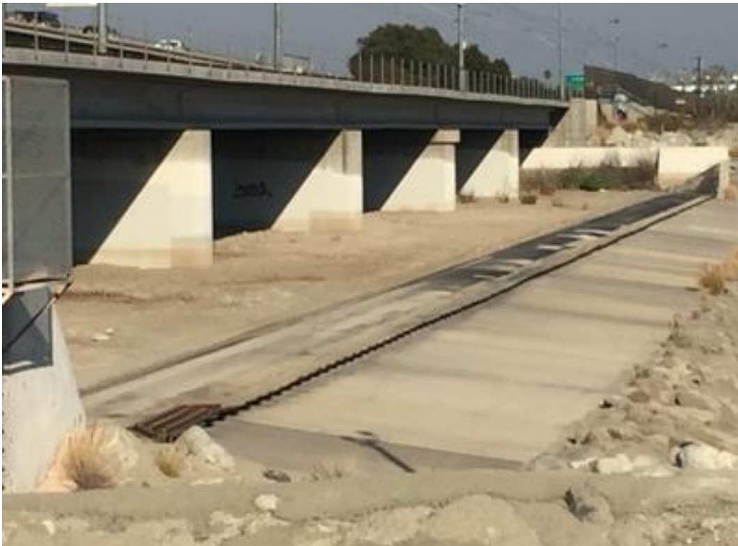
PHOTO 10 DEFLATED RUBBER DAM DOWNSTREAM VIEW
