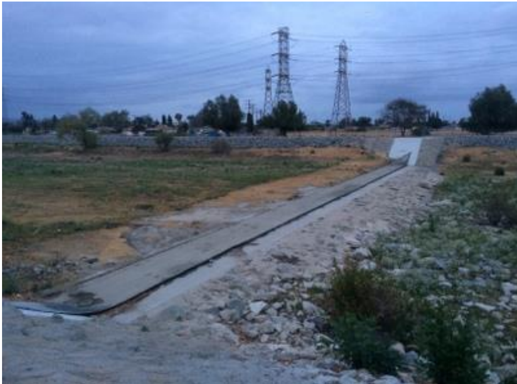
PHOTO 2 DEFLATED RUBBER DAM DOWNSTREAM VIEW
