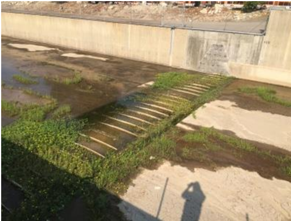
DEFLATED RUBBER DAM DOWNSTREAM VIEW (2016)
