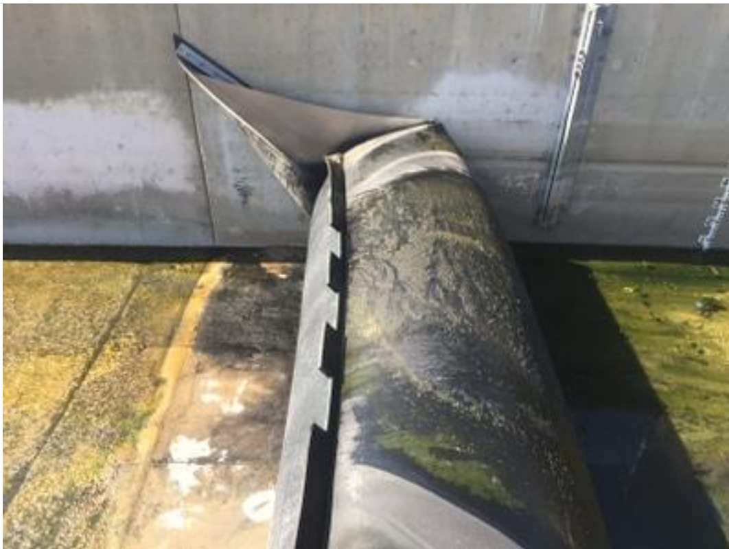
PHOTO 6 INFLATED RUBBER DAM TOP VIEW LEFT ABUTMENT
