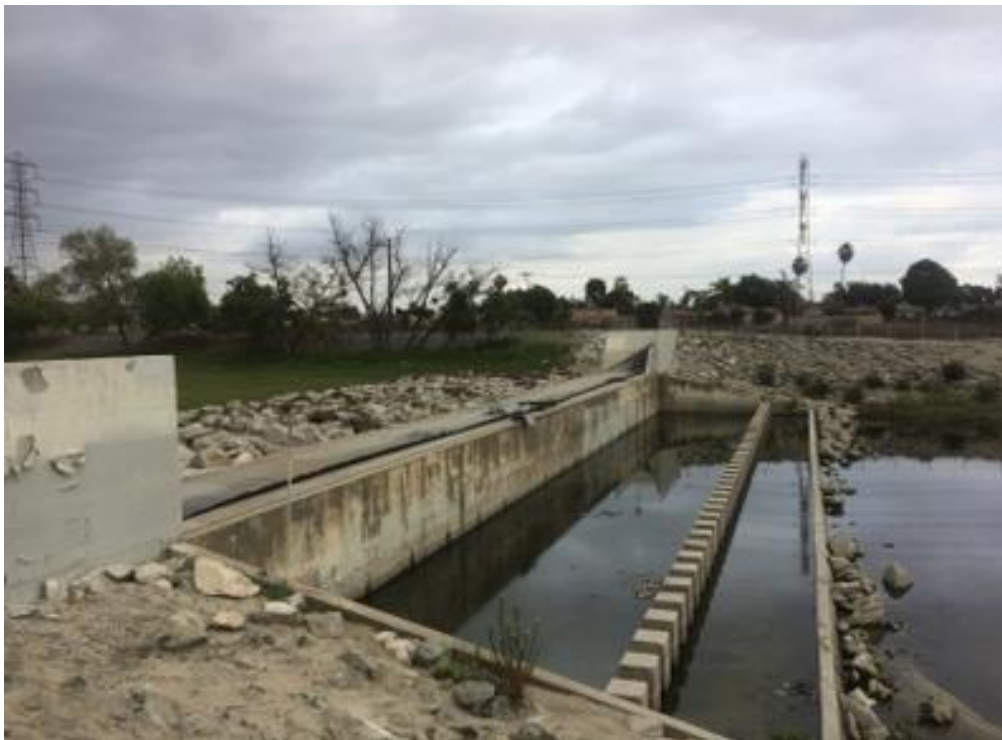
PHOTO 2 DEFLATED RUBBER DAM DOWNSTREAM VIEW
