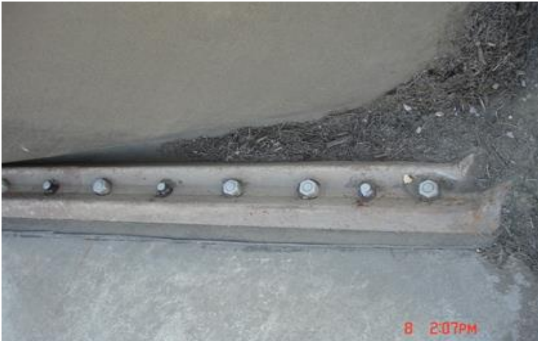
PHOTO 11 MISSING BOLT RIGHT AUTMENT
