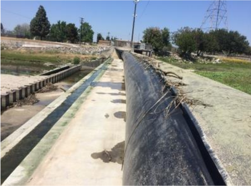
PHOTO 5 INFLATED RUBBER DAM UNDER FIN LEFT ABUTMENT DETAIL
