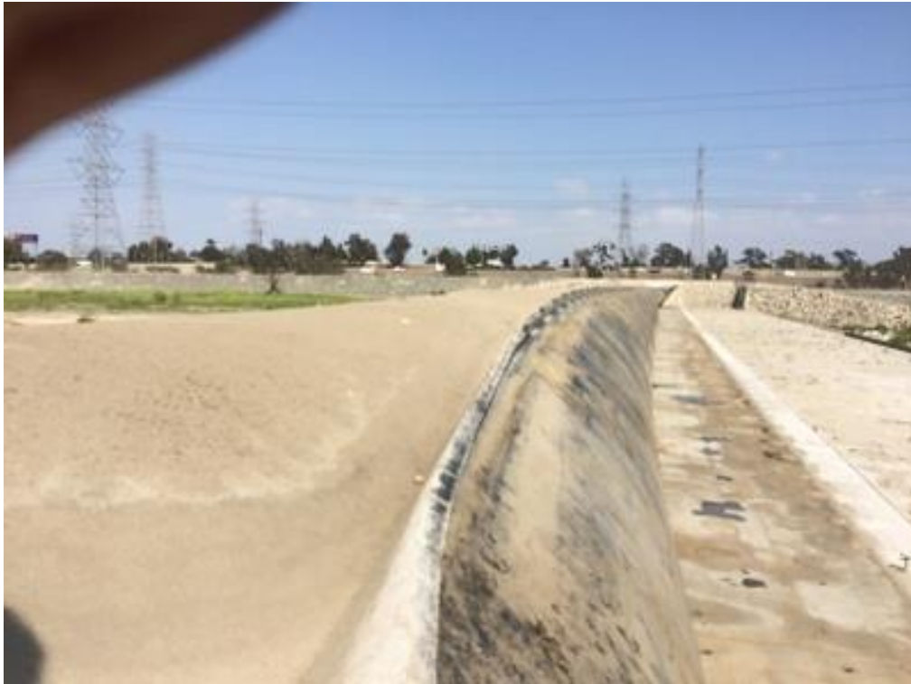
PHOTO 5 INFLATED RUBBER DAM UNDER FIN RIGHT ABUTMENT
