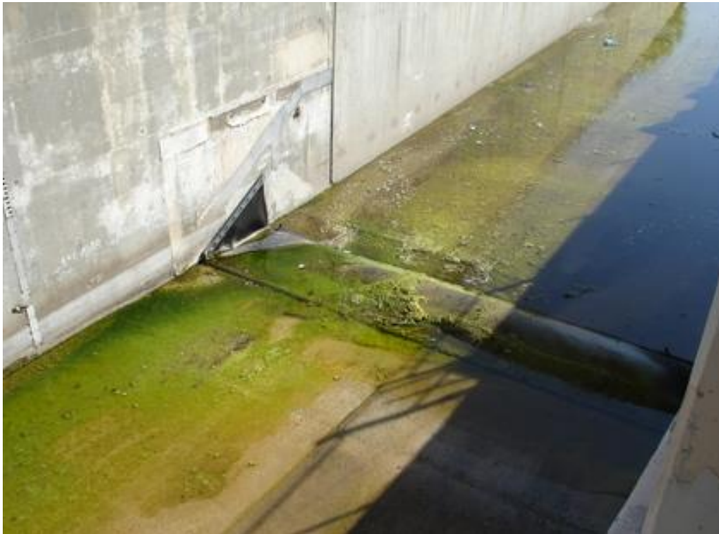
PHOTO 4 DEFLATED RUBBER DAM DOWNSTREAM VIEW (2017)
