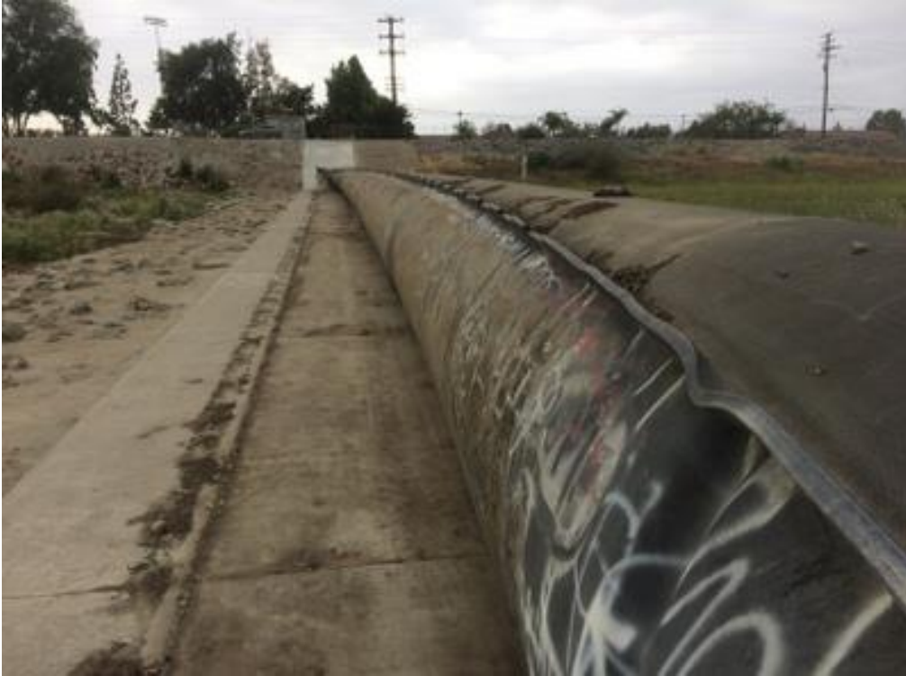
PHOTO 8 INFLATED RUBBER DAM TOP VIEW LEFT ABUTMENT
