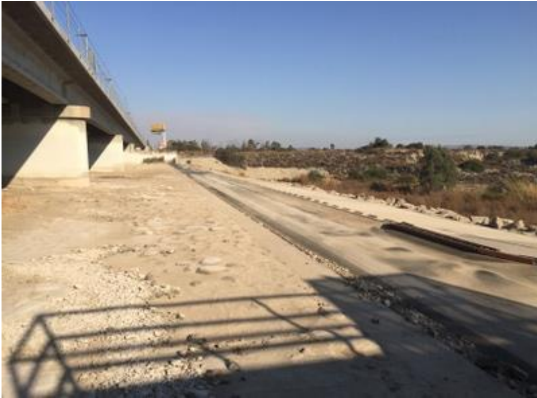
PHOTO 9 DEFLATED RUBBER DAM UPSTREAM VIEW
