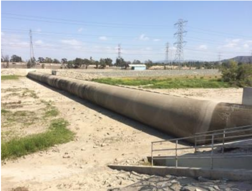
PHOTO 4 INFLATED RUBBER DAM DOWNSTREAM VIEW
