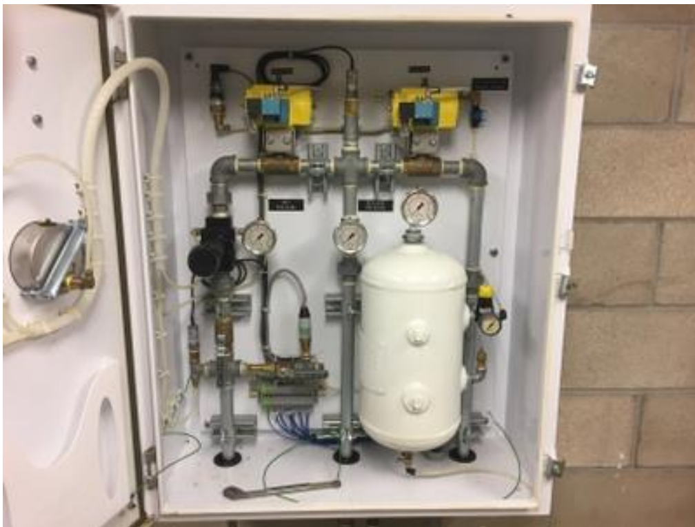
PRESSURE REGULATION CONTROL PANEL INTERIOR VIEW
