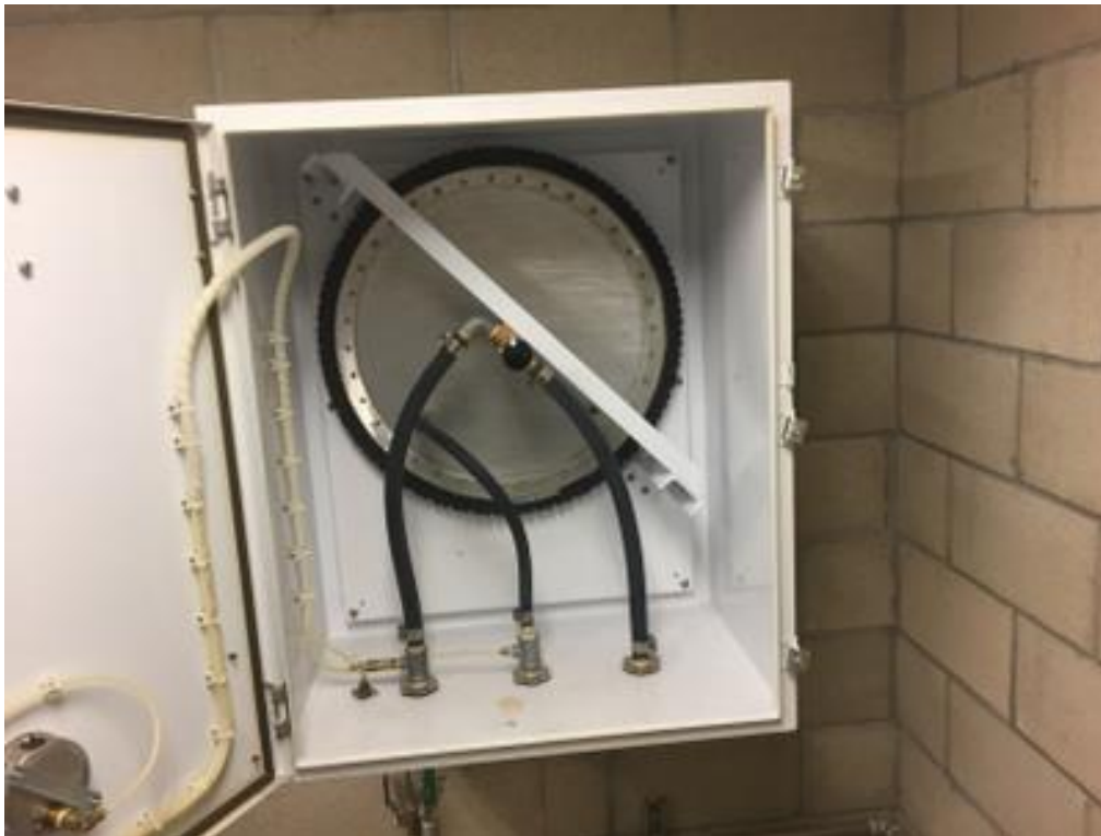
OVERPRESSURE RELIEF CONTROL PANEL INTERIOR VIEW
