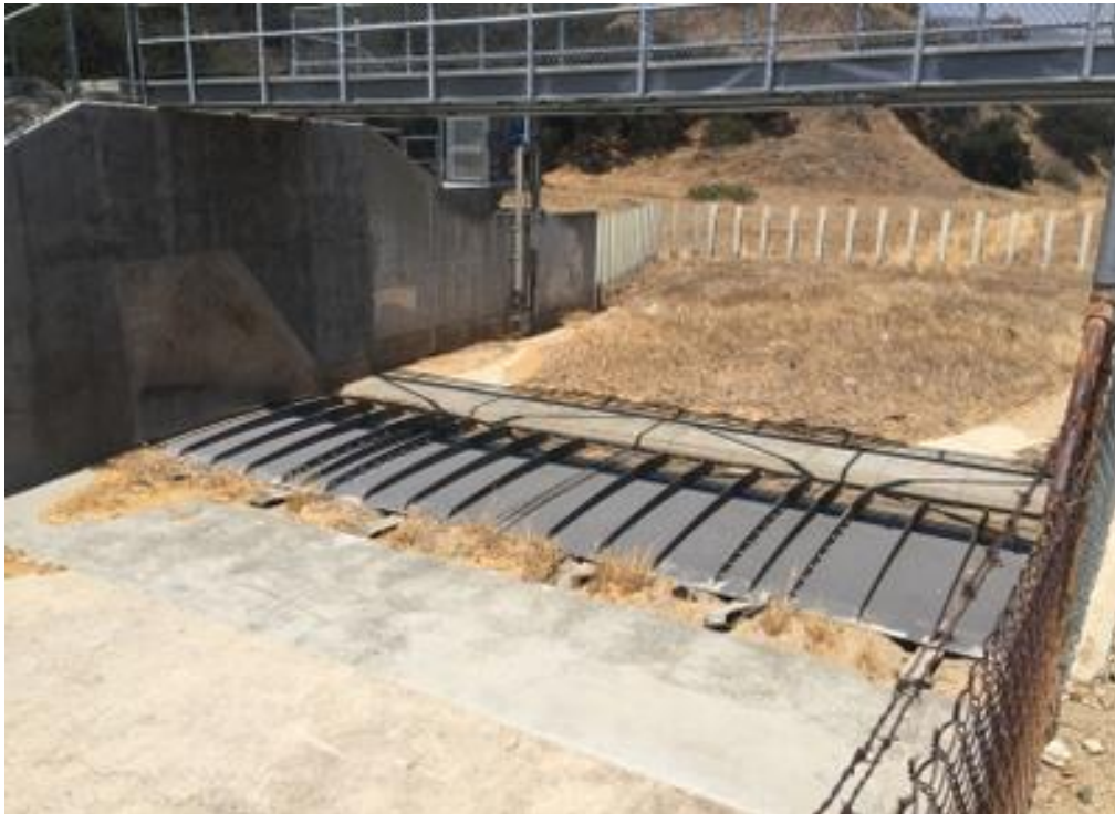
PHOTO 2 DEFLATED RUBBER DAM DOWNSTREAM VIEW
