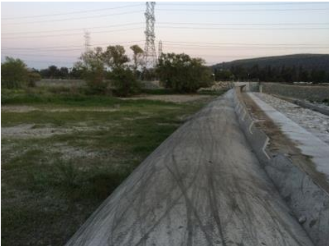
PHOTO 6 INFLATED RUBBER DAM TOP VIEW RIGHT ABUTMENT
