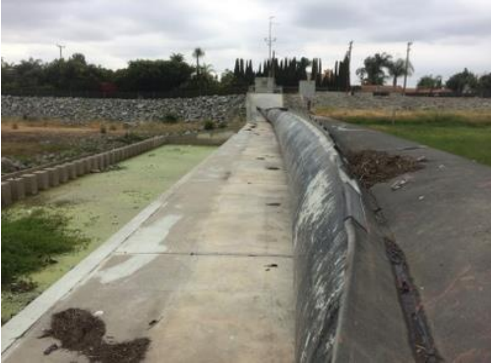
PHOTO 7 INFLATED RUBBER DAM UNDER FIN LEFT ABUTMENT
