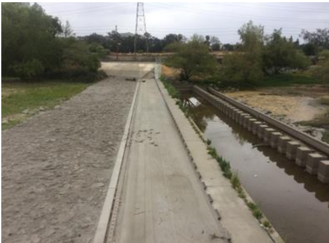
PHOTO 2 DEFLATED RUBBER DAM DOWNSTREAM VIEW
