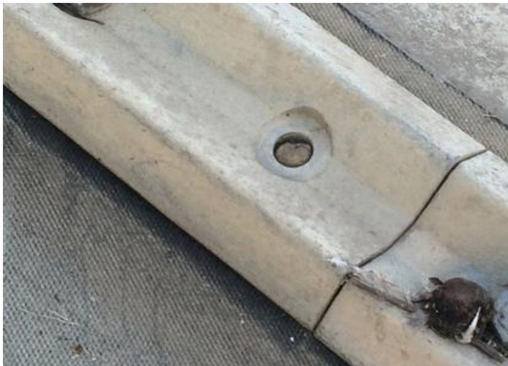
PHOTO 12 MISSING BOLT RIGHT AUTMENT DETAIL
