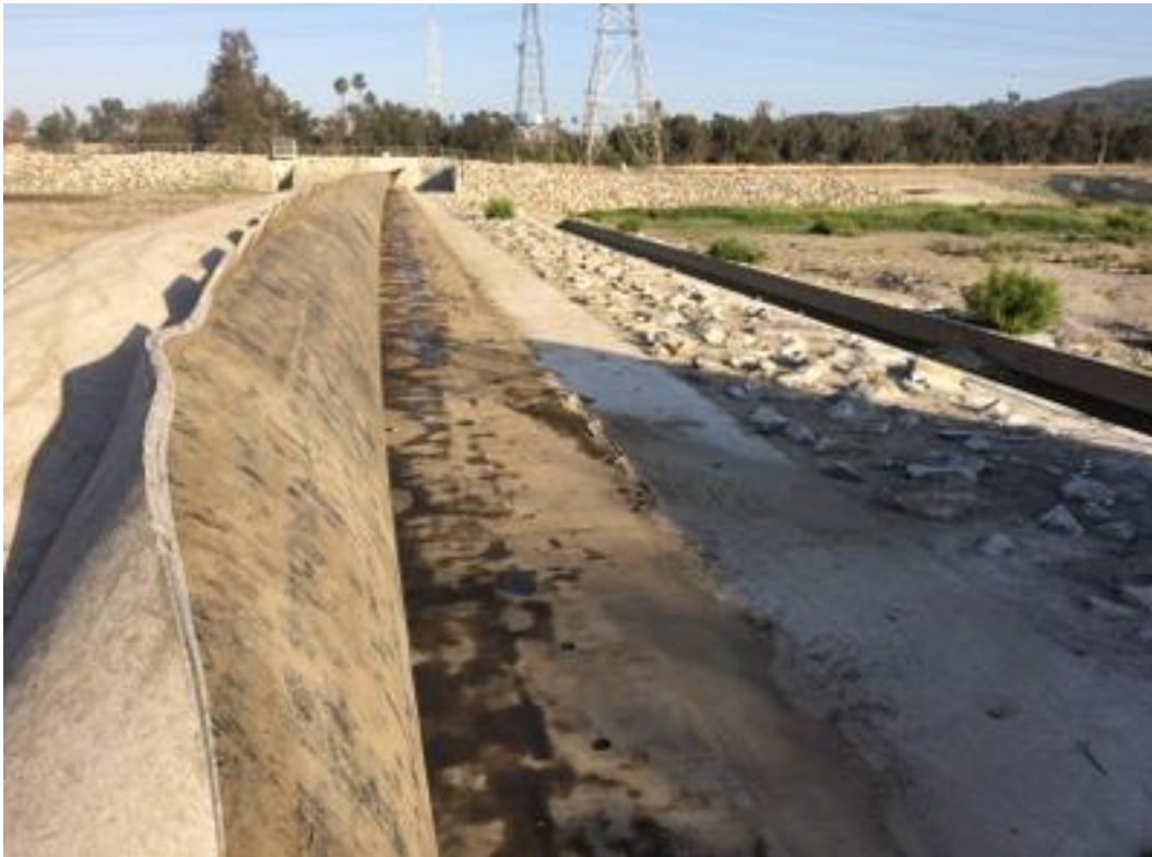
PHOTO 5 INFLATED RUBBER DAM UNDER FIN RIGHT ABUTMENT
