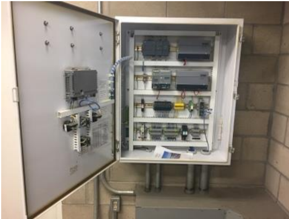
PLC CONTROL PANEL INTERIOR VIEW
