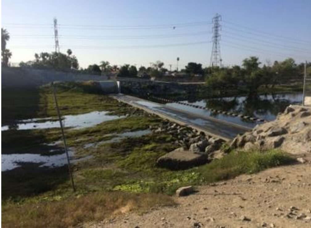
PHOTO 1 DEFLATED RUBBER DAM UPSTREAM VIEW
