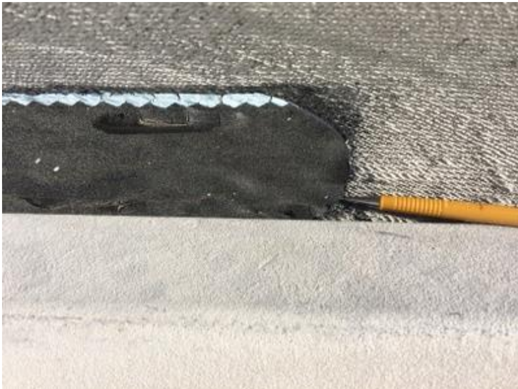
DETERIORATED CLASS D REPAIR
