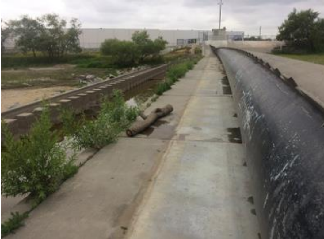
INFLATED RUBBER DAM UNDER FIN LEFT ABUTMENT
