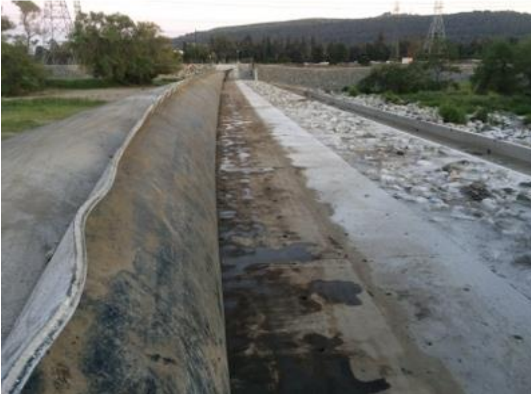
PHOTO 5 INFLATED RUBBER DAM UNDER FIN RIGHT ABUTMENT
