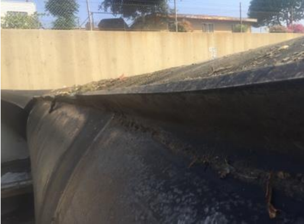
PHOTO 6 INFLATED RUBBER DAM TOP VIEW LEFT ABUTMENT
