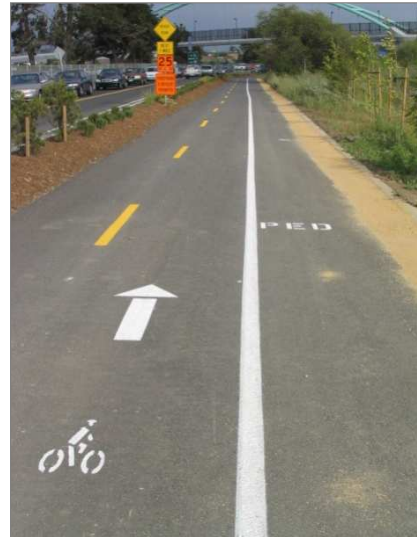
Centerline striping and directional arrows encourage trail users to provide space for other users to pass.
