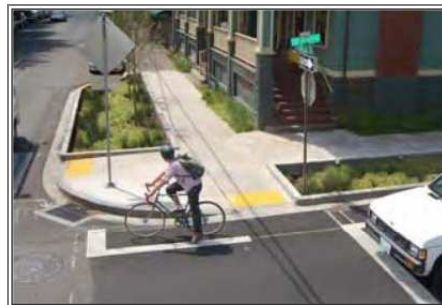
Bicycle forward stop bars encourage cyclists to wait where they are more visible.
