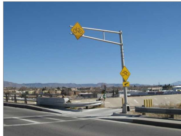
Type 1 crossings include signage and pavement markings.
