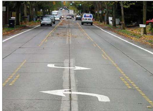
This road was re-striped to convert four vehicle travel lanes into three travel lanes with bike lanes.
