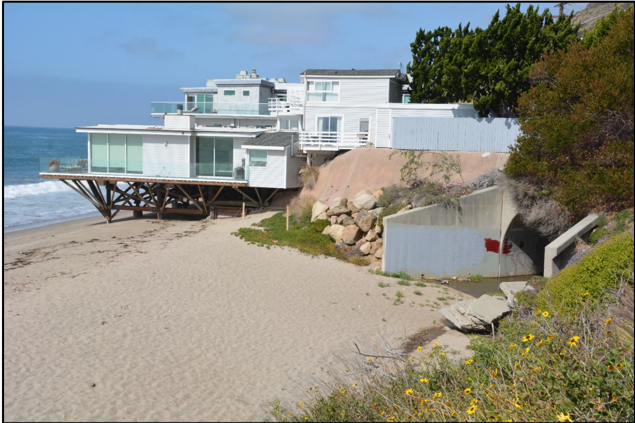
Figure 4-14. Property adjacent to culvert outlet that could be effected by increased sand buildup from any structure placed on the beach perpendicular to the ocean.
