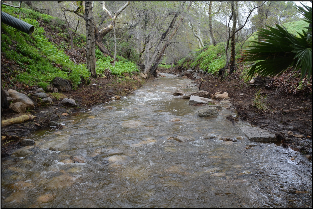
Figure 3-11. Solstice Creek looking upstream from the Highway 1 Culvert, February 21, 2017.
