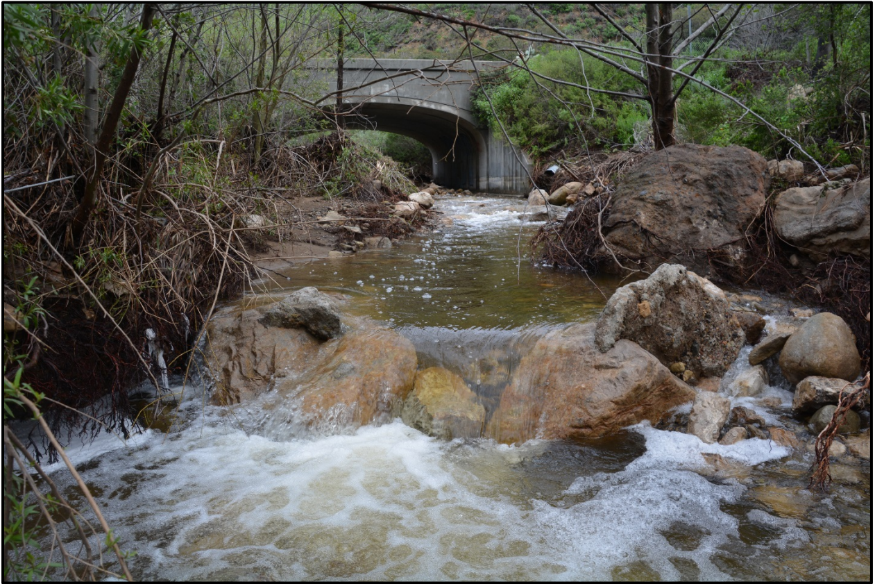
Figure 3-12. Solstice Creek looking upstream towards Corral Canyon Culvert, February 21, 2017.
