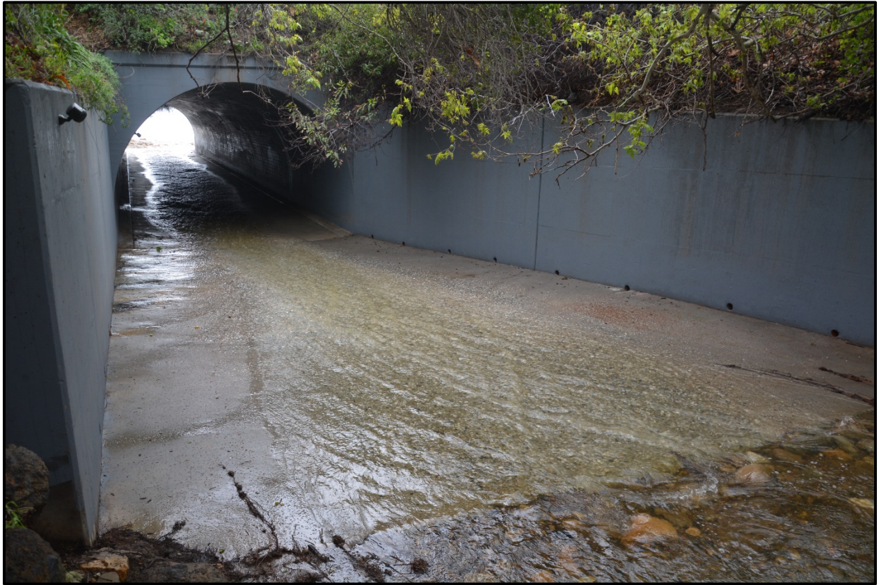
Figure 3-10. Highway 1 Culvert on Solstice Creek, February 21, 2017. No sediment deposits were observed in the culvert. Flow conditions in the culvert would be too shallow for passage.
