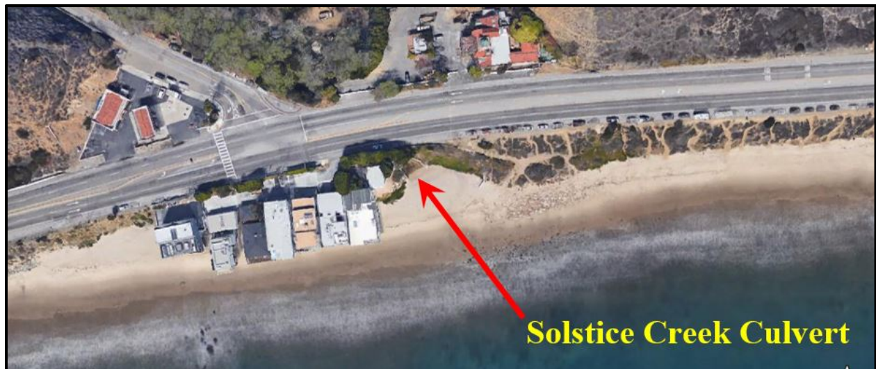
Figure 1-2. Solstice Creek Culvert at Dan Blocker State Beach, Malibu, California.
