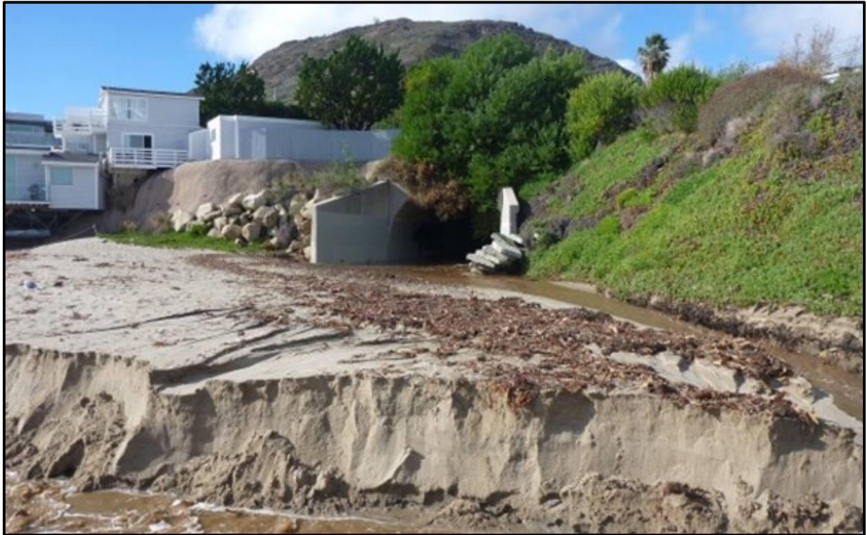
Figure 6-1. Solstice Creek (unknown date). After exiting the culvert, the creek took a sharp left turn, followed the base of the highway embankment, and then took a sharp right turn towards the ocean.
