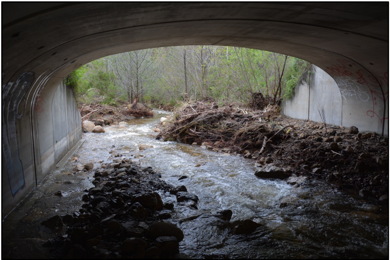
Figure 3-13. Solstice Creek looking downstream through Corral Canyon Culvert, February 21, 2017.
