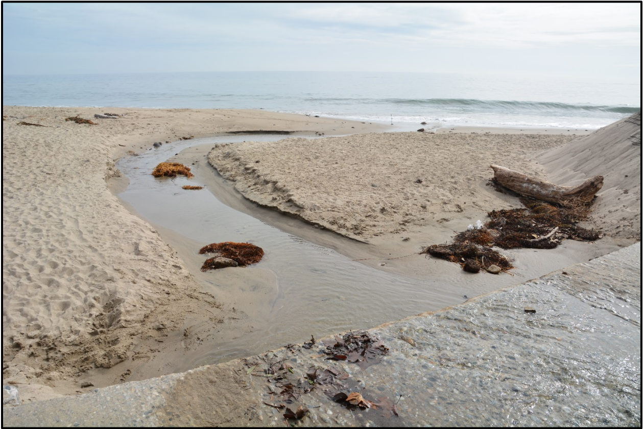
Figure 3-7. Solstice Creek, looking downstream from culvert on February 2, 2017. The creek carved out a channel with a bend.
