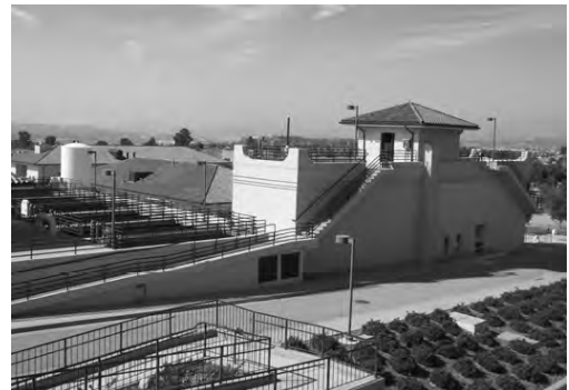
Rio Vista Water Treatment Plant
