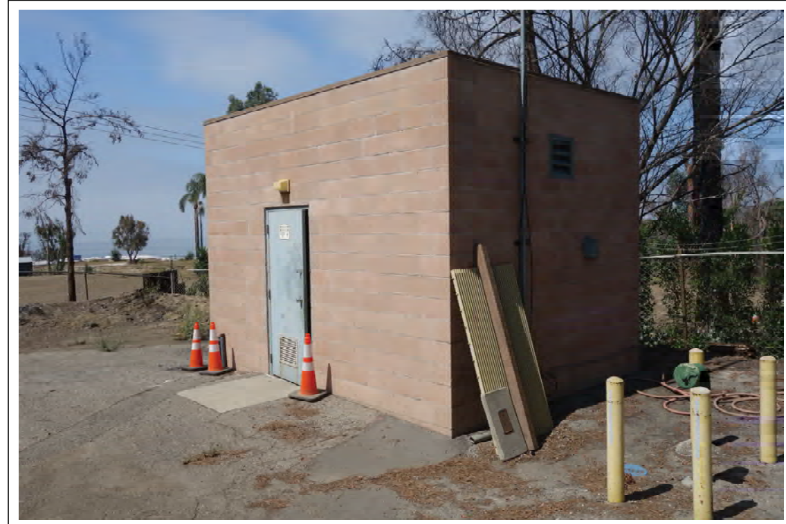
Photo 2: View looking southwest from the northwest part of the site of the electrical and restroom building in the west part of the site.
