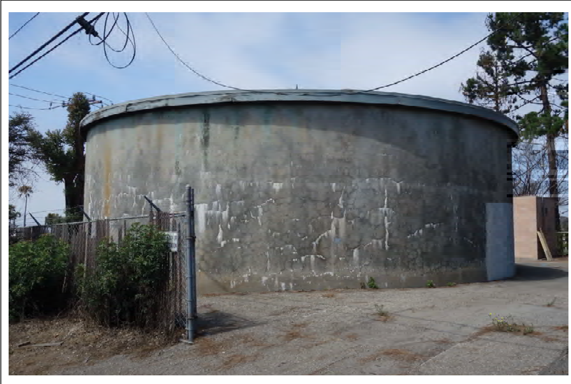
Photo 1: View southwest from the northeast corner of the project site showing the tank; part of the electrical and restroom building is visible on the right.
