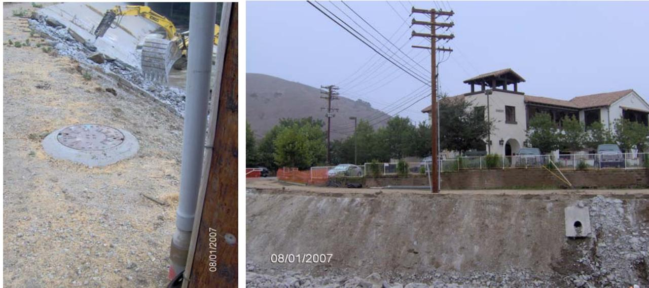
After the concrete removal the sewer line was inspected and it suffered no damage. Fortunately, the power pole was located on the bank and due to its elevation was not at risk of being hit by the excavators that were working in the channel. However, one of the power poles did hamper debris removal because it forced the dump trucks to have to use the downstream entrance, which exited directly onto a busy road.
