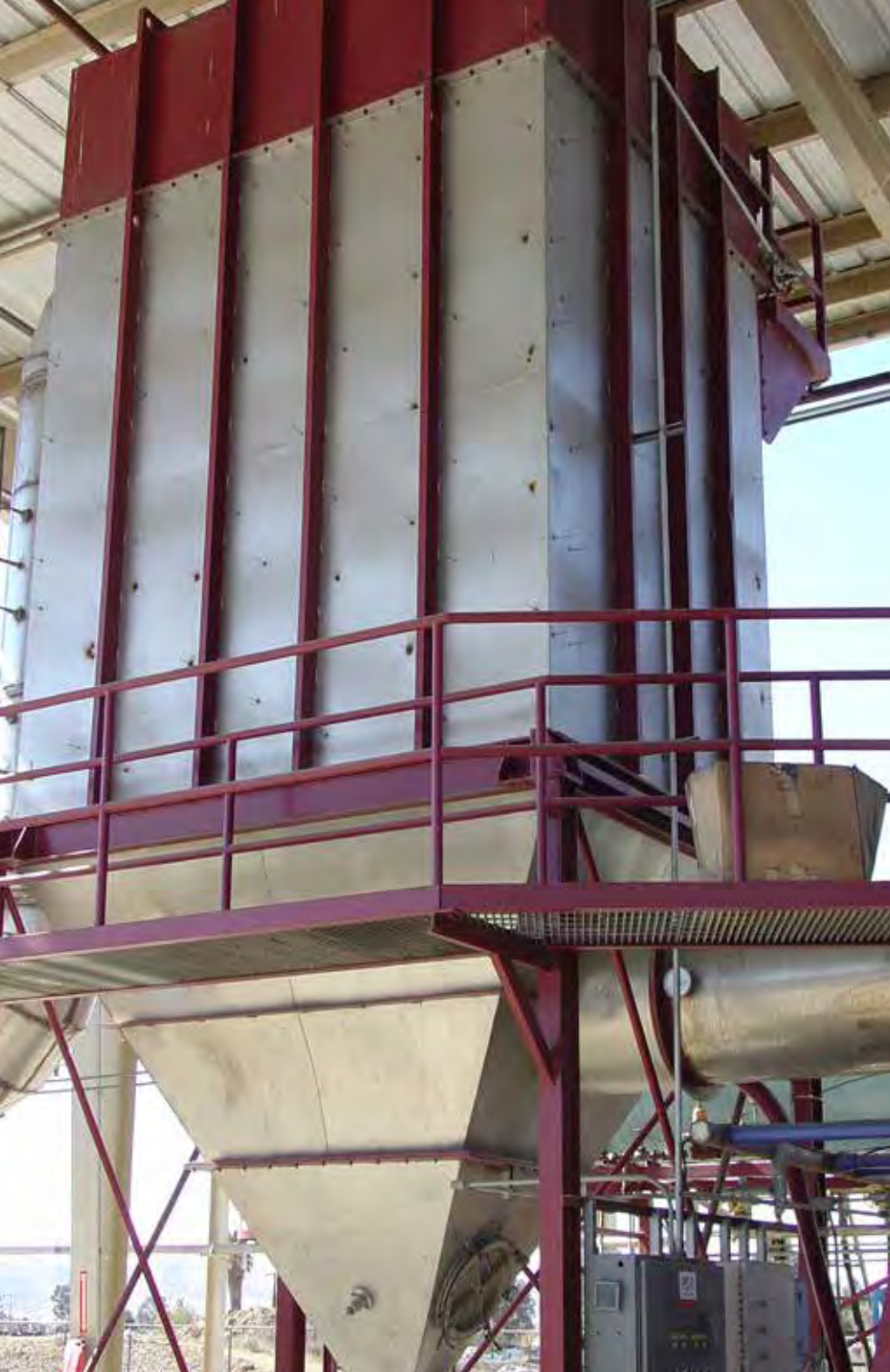
IES Pyrolysis Facility in Romoland, CA
