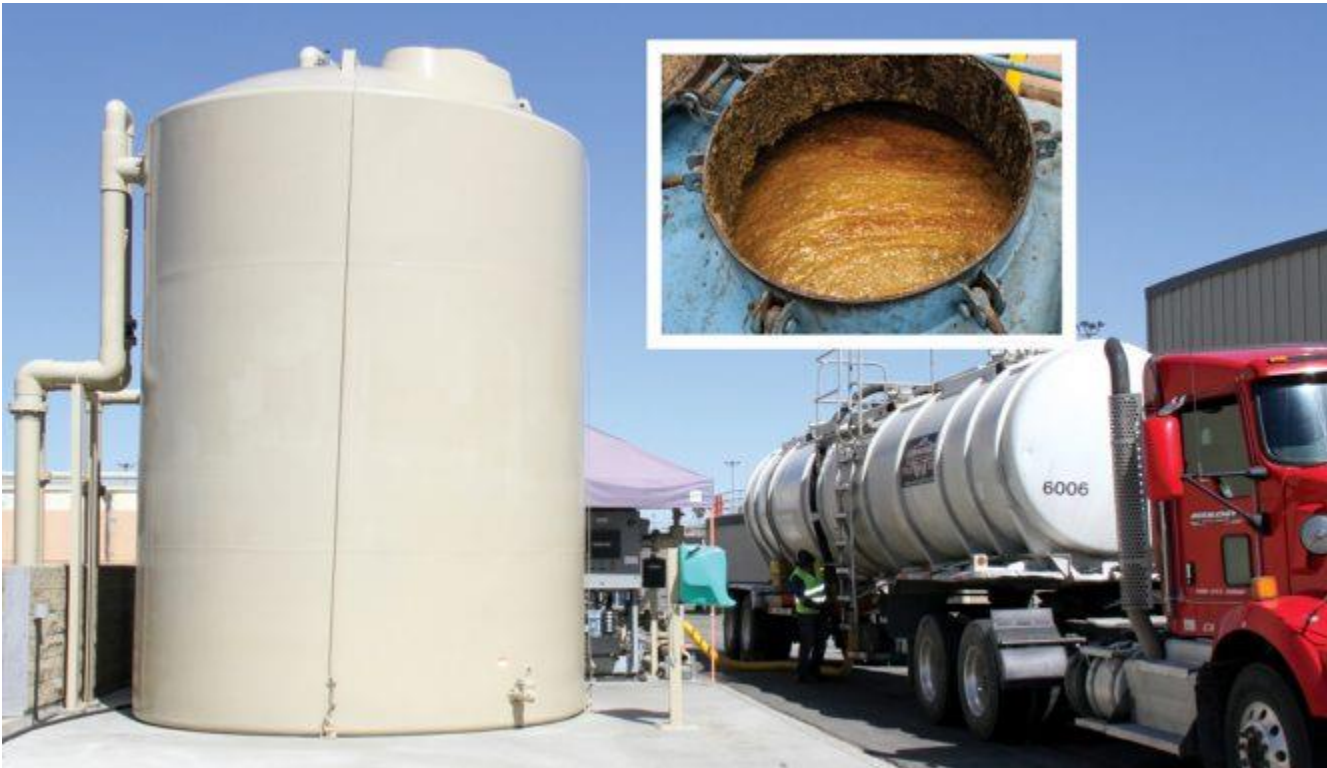
A tanker truck unloads processed food waste slurry (above, left) into 15,000 gallon storage tanks. A typical tanker load is 4,600 to 4,800 gallons. Photo courtesy of Los Angeles County Sanitation Districts, Inset photo by Kelly Sarber
