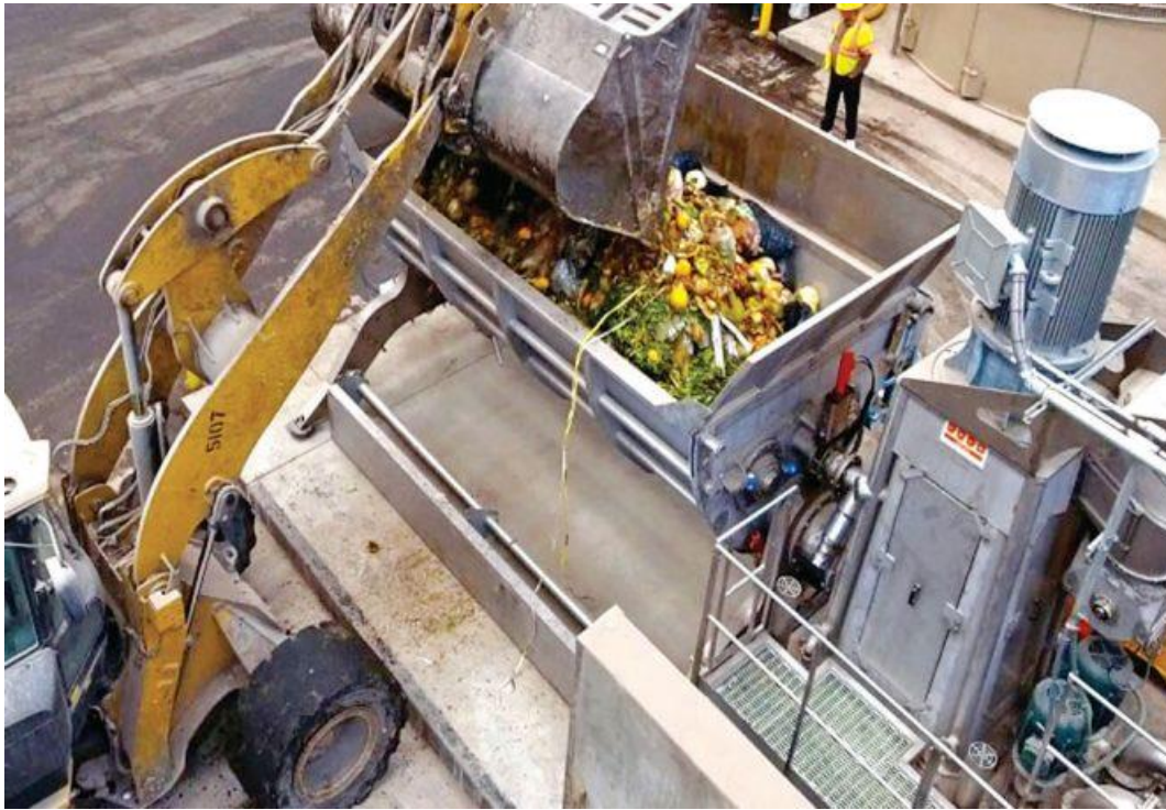
Food waste from commercial generators is loaded into a hopper with augers that move the material to the bioseparators. Photo courtesy of Los Angeles County Sanitation Districts
