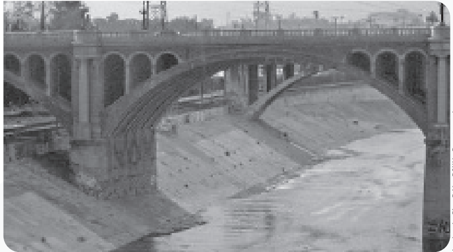
Los Angeles River Bridge B&W by Downtowngal
