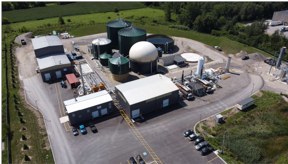
Aerial of StormFisher's London Biogas Facility
