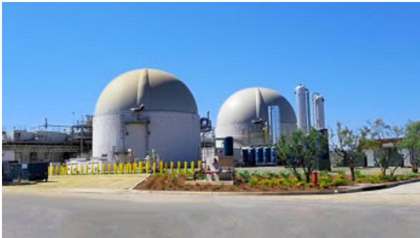
CR&R Anaerobic Digestion Facility Perris, CA
