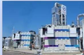
Tri-generation 2.35 MW net power 1,270 kg/day hydrogen 1,400 gal/day water
