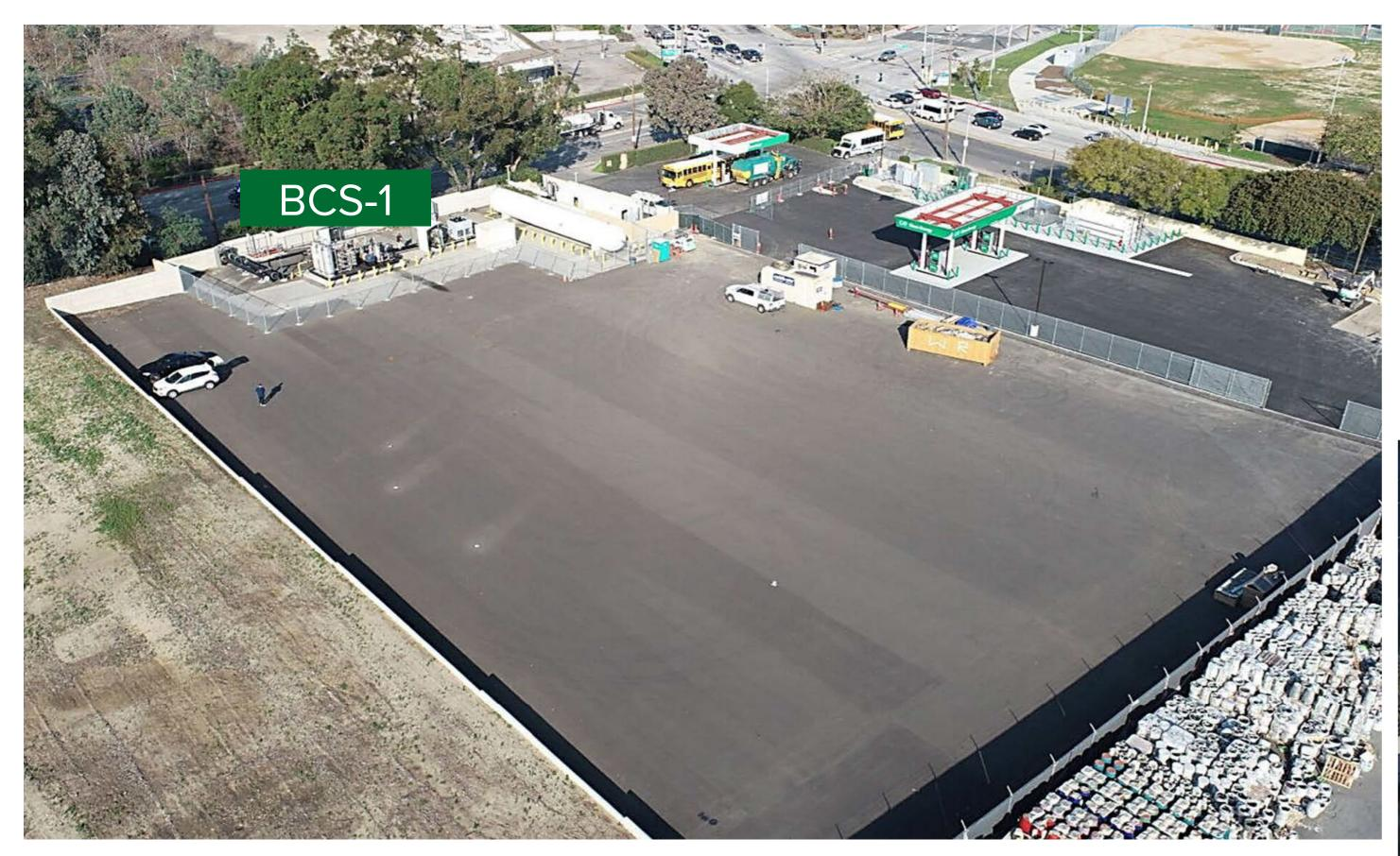
Gas is stored and feed to compressors with priority over pipeline gas. Pipeline gas needed when JWPCP RNG is unavailable or has insufficient pressure
