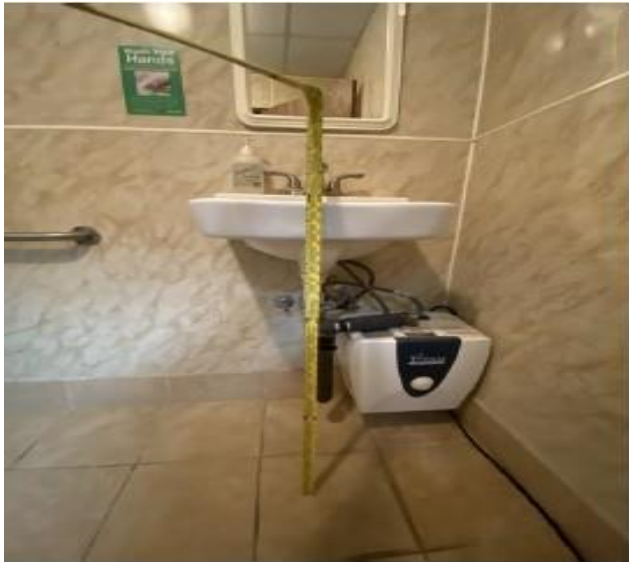
Maintain toe and knee clearance under lavatory. Left photo shows equipment stored under sink that is encroaching on the clearance space.
