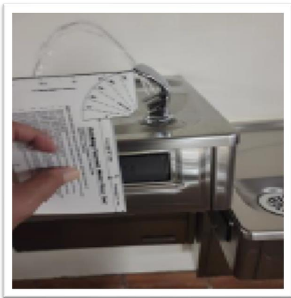
Good water flow at Santa Clarita facility at time of inspection.
