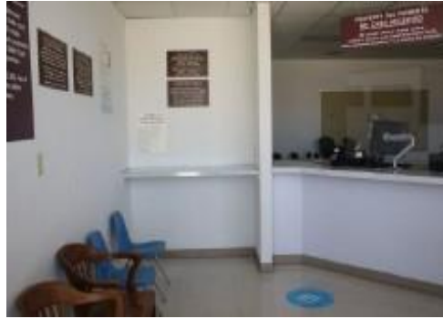
Counters in the top and right photos are mounted too high. Photo below shows counter height is 5" higher than the 34" maximum above the finished floor allowed.
