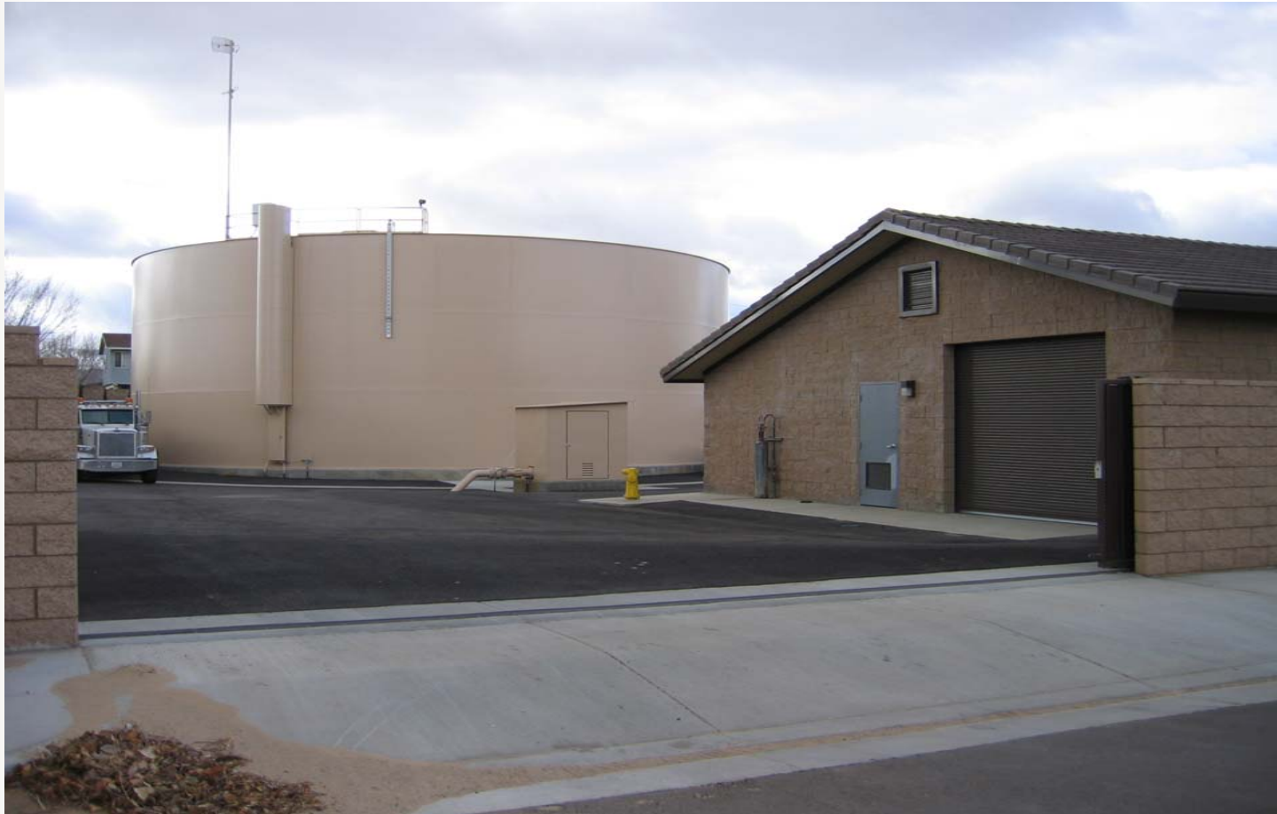
Well 5A Pump Station
