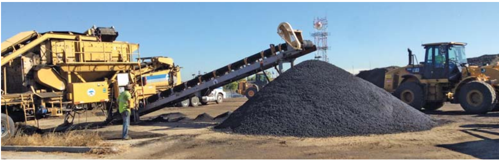
More than 21,000 tons of material was kept out of landfills via the employment of recycling tactics on-site—which also produced a cost savings of $1.1 million.
