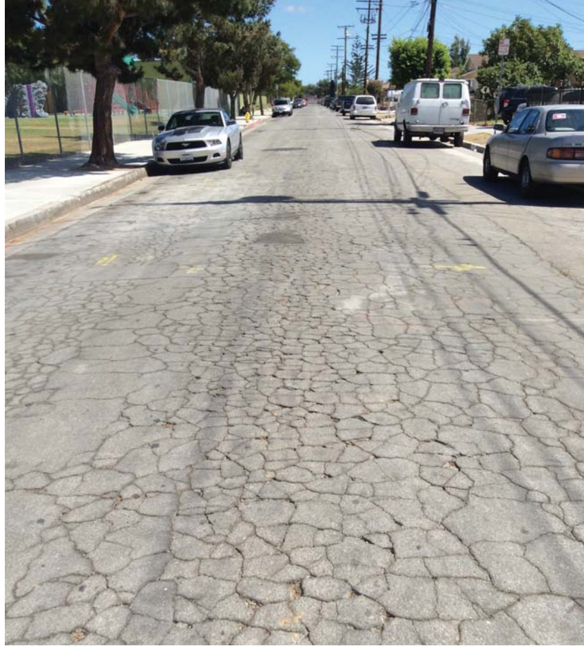
Above: Significant alligator and map cracking was observed at the site prior to the project’s undertaking.
