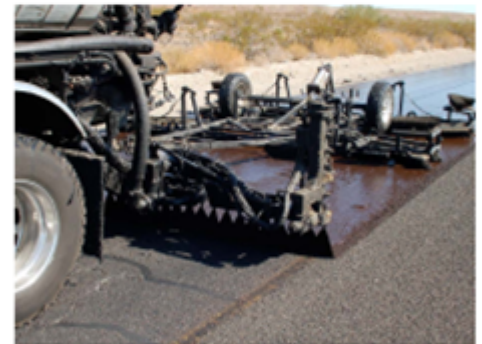
Application of PASS CR for the scrub seal
