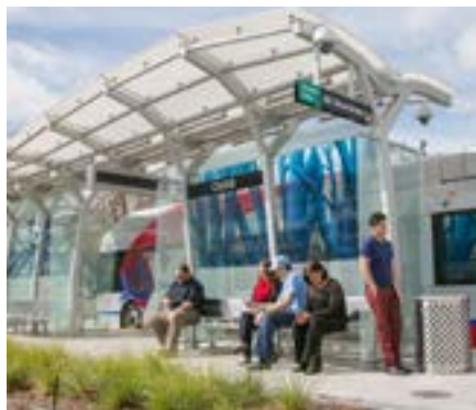
sbX BRT Shelter, San Bernardino, CA
