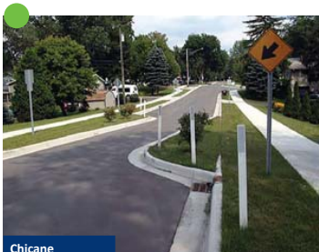
Chicane Chicanes provide alternating narrow and wide sections, and a curved driving path similar to a slalom. Chicanes increase the amount of public space available on a corridor and can be activated using benches, bicycle parking, and other amenities.
