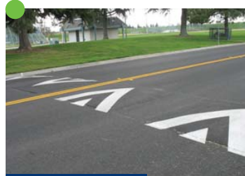
Speed Cushion Speed cushions work by lifting the entire wheelbase of a vehicle to lower its speed and have wheel cutouts that enable larger emergency vehicles to pass without any impact, while still reducing the speed of passenger cars.
