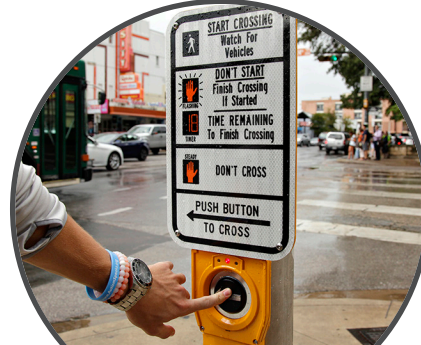
ACCESSIBLE PEDESTRIAN SIGNAL
