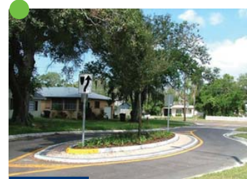
Median Island Median islands are raised islands located along the street centerline that narrow the travel lanes at that location. They are a pedestrian benefit, because they can serve as a place of refuge for pedestrians who cross a street midblock or at intersections.
