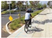
1B - Curb-separated cycletrack (bi-directional)
