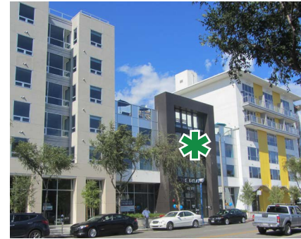
* Varied heights along corridor
