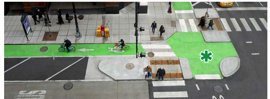
* Bike queuing space at intersection protected by curb extensions Chicago, IL (Source: John Greenfield)
