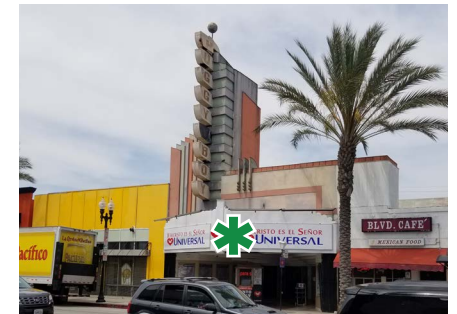
* Preserved unique historic building
