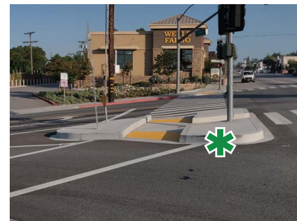
* Curb ramp with refuge island La Crescenta, LA County UA (Source: LA County)
