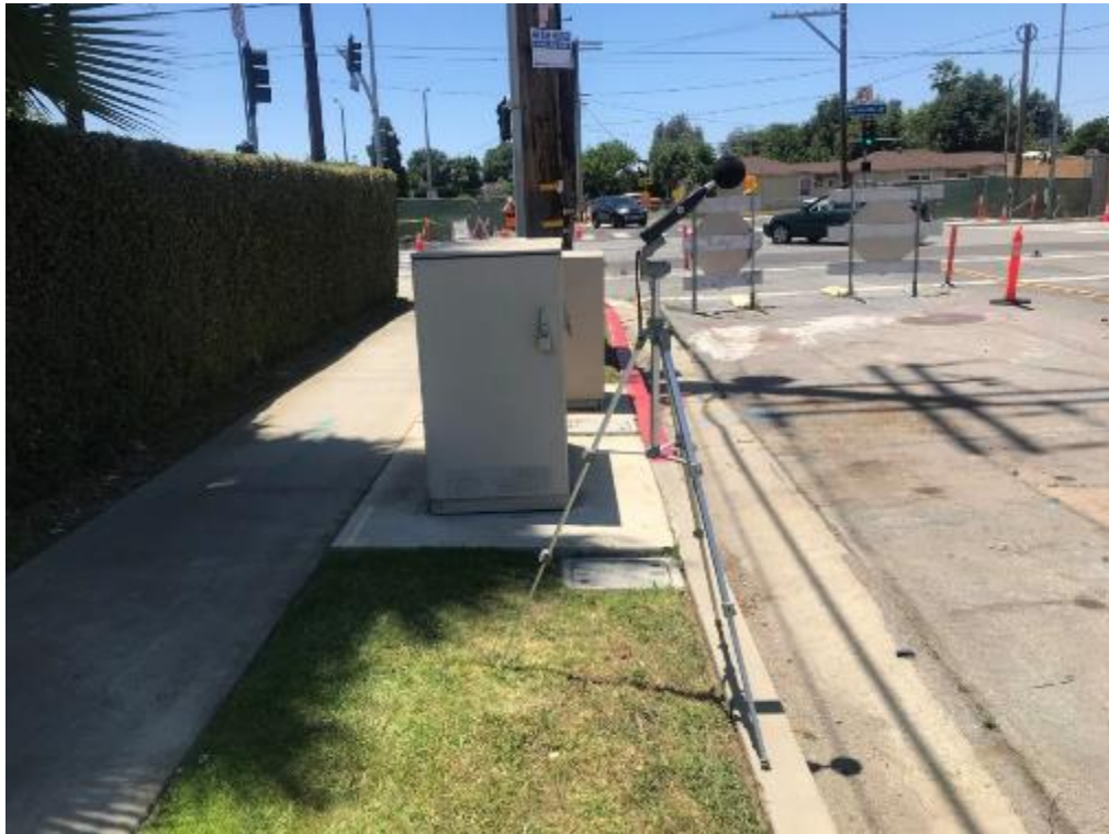
ST3 looking West
