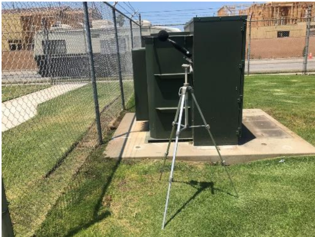
ST2 looking West
