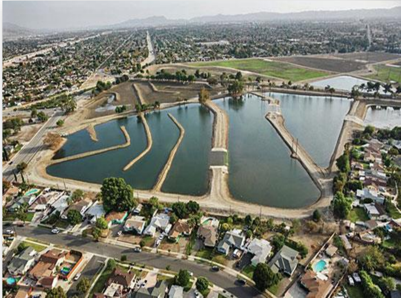
Pacoima Spreading Grounds
