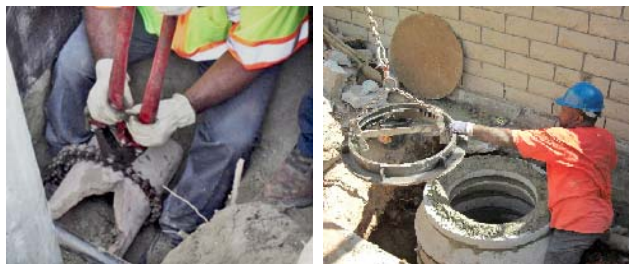
Construction workers fixing sewer pipe (left) and adjusting manhole to surface level (right).
