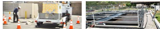
Worker is checking pump station in the City of South El Monte (left) Treatment Plant in Malibu (right).
