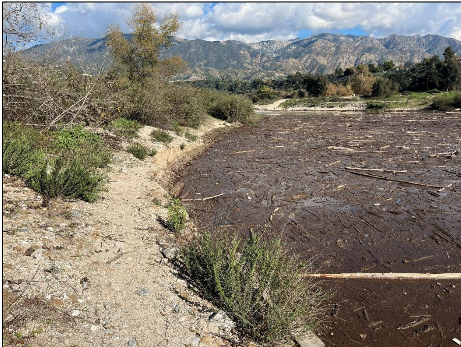
Photo 12: Overview Side Slopes
