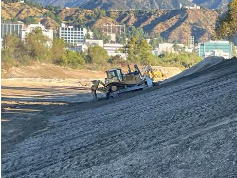
Bulldozer_grading_hillside_faceNorth.jpg -118.17278408888889 34.18987609722222
