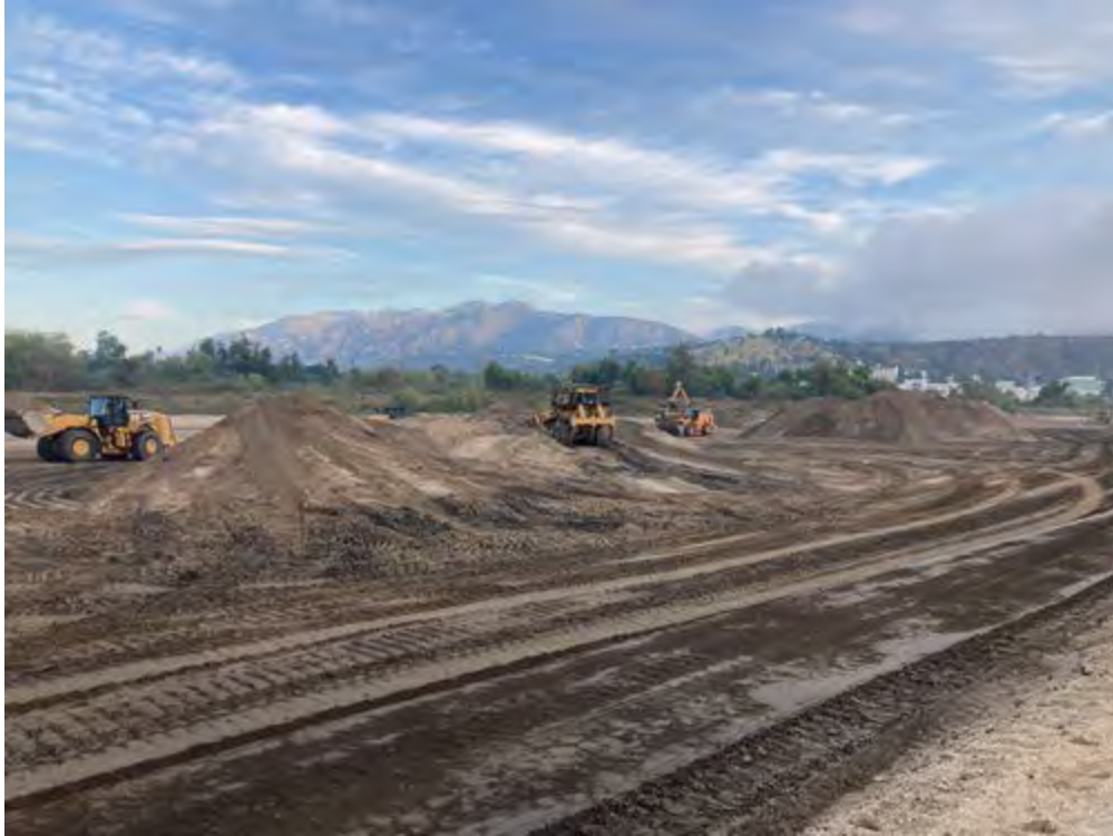
Crew_hauling_sediment_out_of_basin_before_facingNorthwest.jpg -118.17337816666667 34.18886282222222
