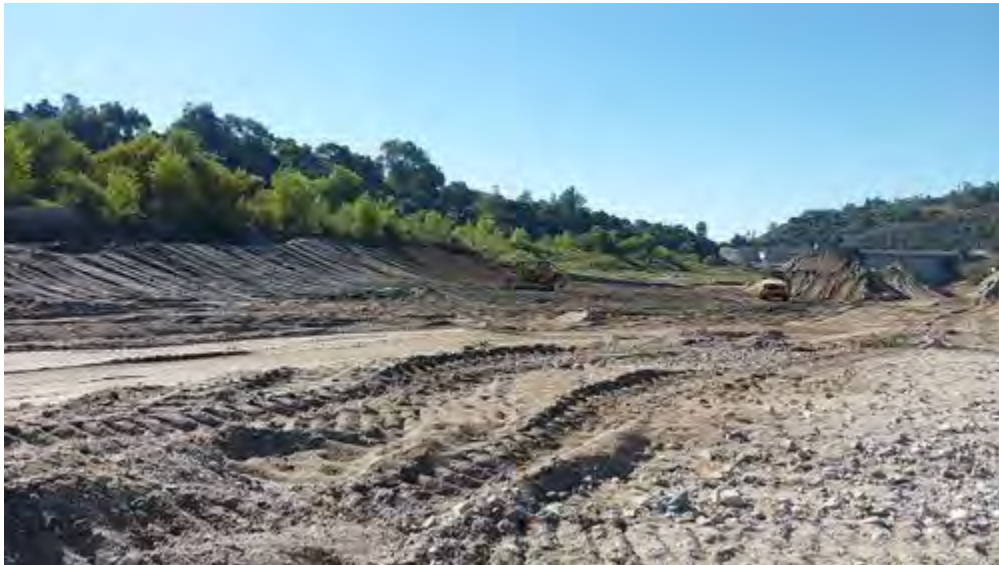
bulldozer_compacting_bank_reconstruction_facingSouthSoutheast.jpg
