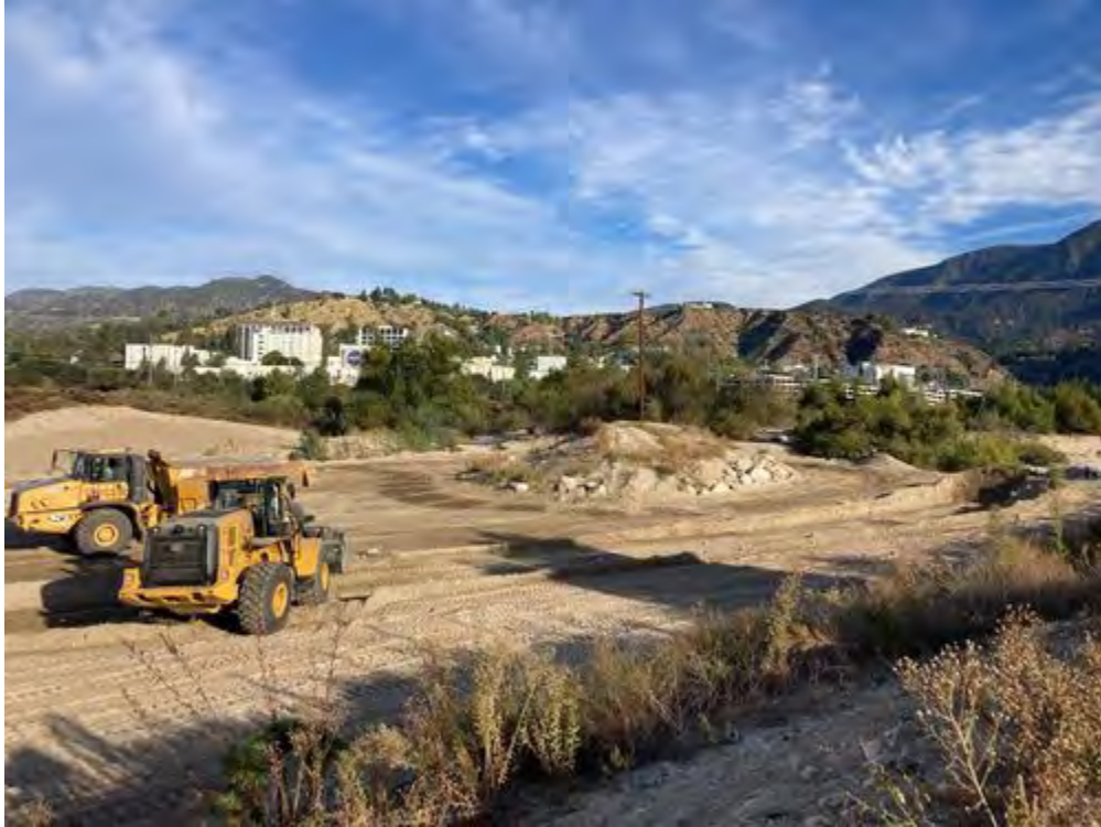
Hauling_sediment_out_of_north_end_of_basin_facingNorth.jpg -118.17085803611111 34.19404538888889
