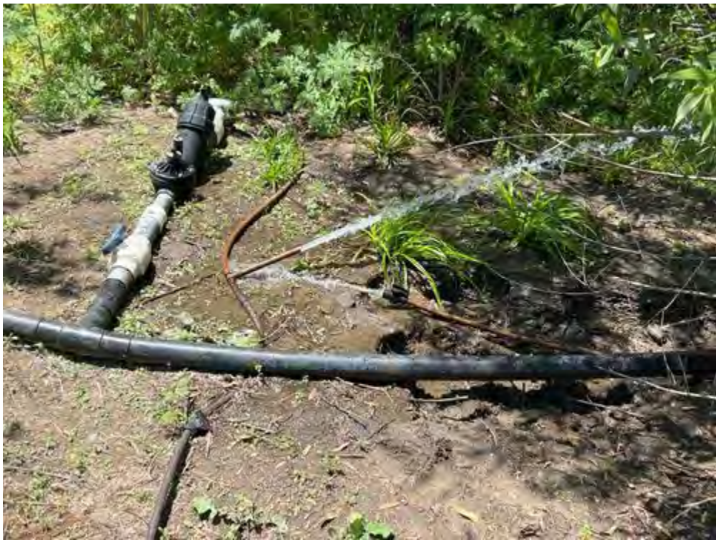
Irrigation_leak_DG-W-2.jpg -118.17462861111112 34.19238029444444
