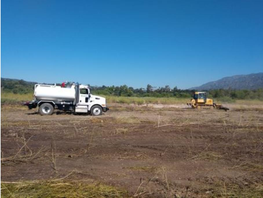
450j and water truck conducting vegetation removal along eastern project boundary
