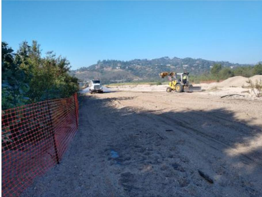
**Box scraping and water deposition of potential eastern haul road**
