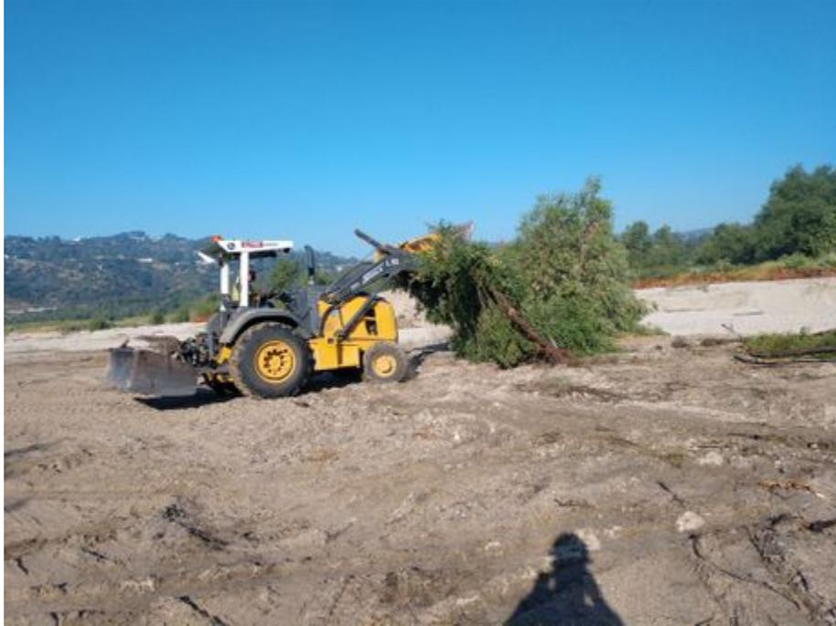
**Front-end loader removing vegetation along eastern project boundary near proposed haul road**
