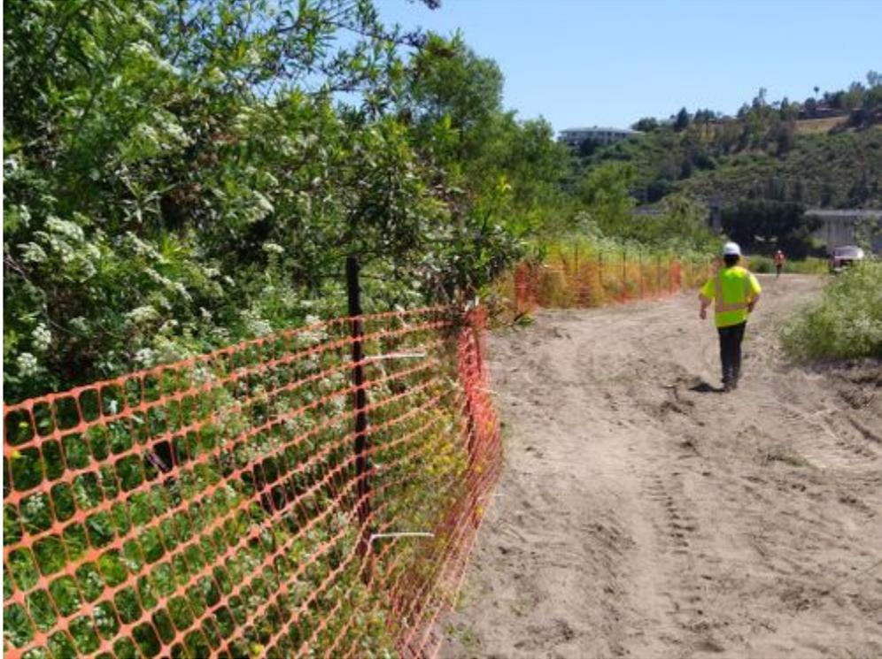
photo\_3-esa fence installed.jpg
