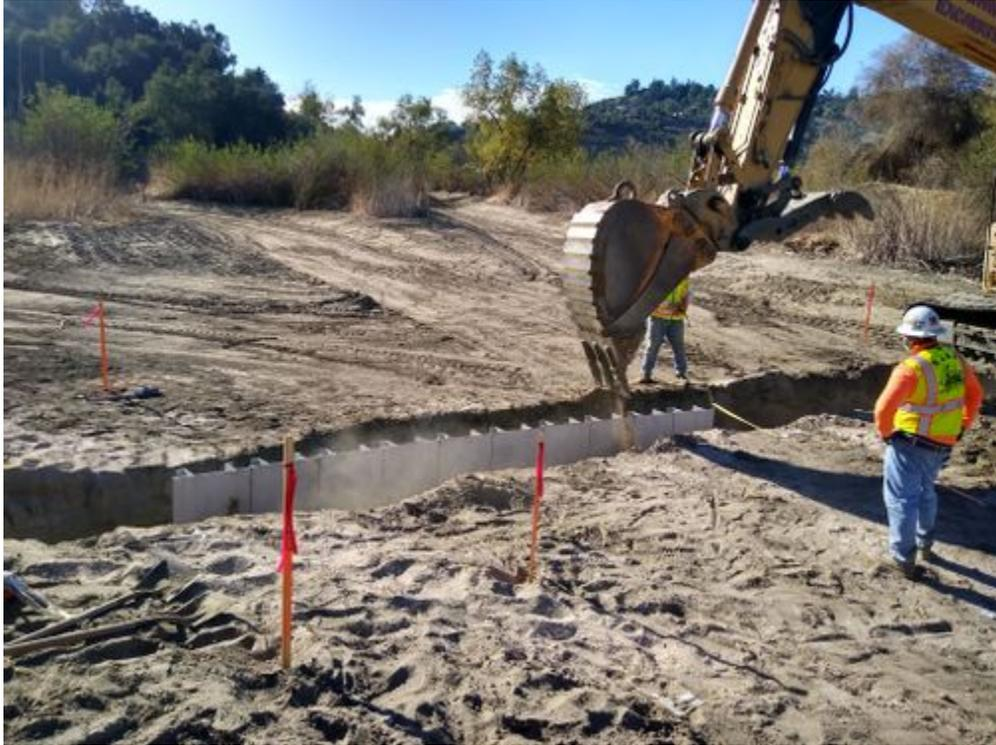
photo\_3-sheet pile install.jpg
