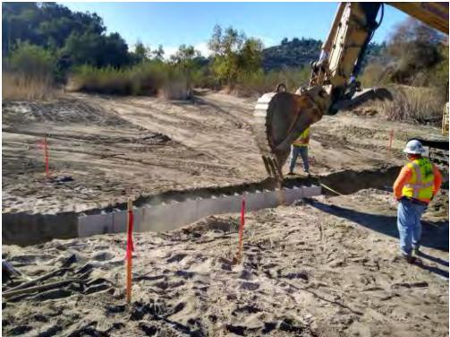
photo\_3-sheet pile install.jpg -118.17194 34.19092
