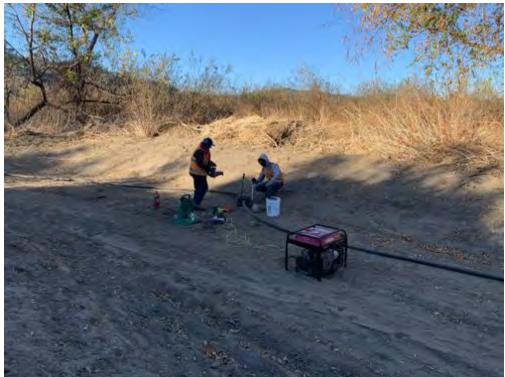
Fusing\_irrigation\_pipes\_during\_facingW.jpg -118.17218 34.19014
