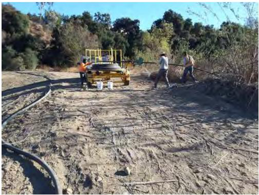
Pipe straightening machine\_DG-W-1.jpg -118.17186 34.19102
