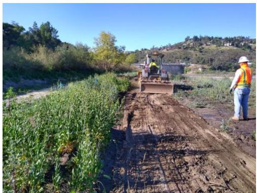
photo\_1-skip loader clearing esa fenceline.jpg -118.17276 34.18913
