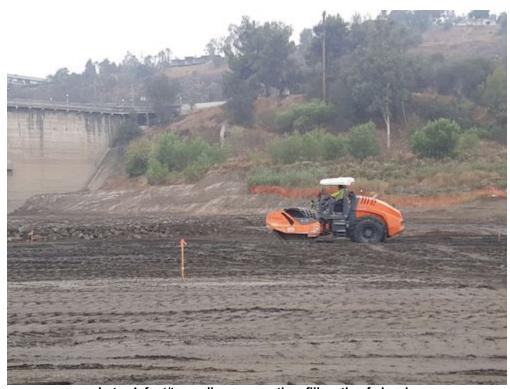
photo\_4\_foot/toe\_roller\_compacting\_fill\_noth\_of\_dam.jpg -118.1753 34.18709
