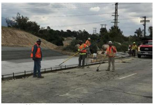
4/3/19 – Pouring concrete pavement for west access road driveway.
