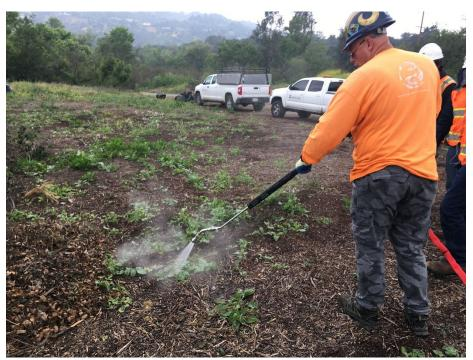
Crew using hot water vapor machine that uses clean water heated to a steam to shock and kill nonnative weeds
