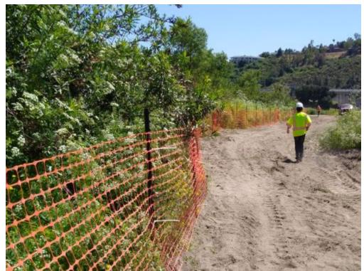
photo\_3-esa fence installed.jpg -118.17269 34.18906
