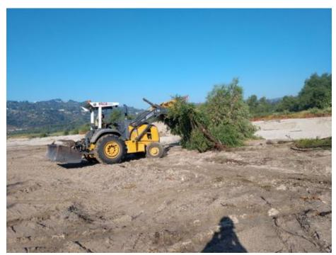
Front-end loader removing vegetation along eastern project boundary near proposed haul road -118.17234 34.19204
