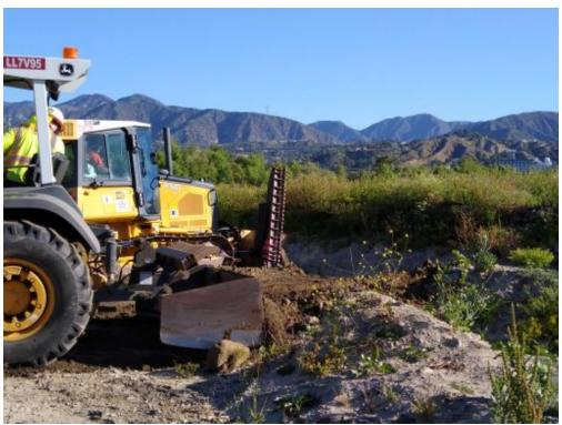
photo\_1-pushing emergent vegetation off slope.jpg -118.17616 34.18687
