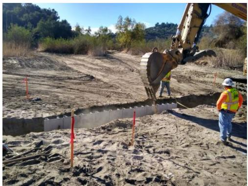
photo\_3-sheet pile install.jpg -118.17194 34.19092
