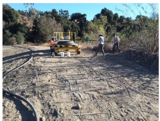
Pipe straightening machine\_DG-W-1.jpg -118.17186 34.19102
