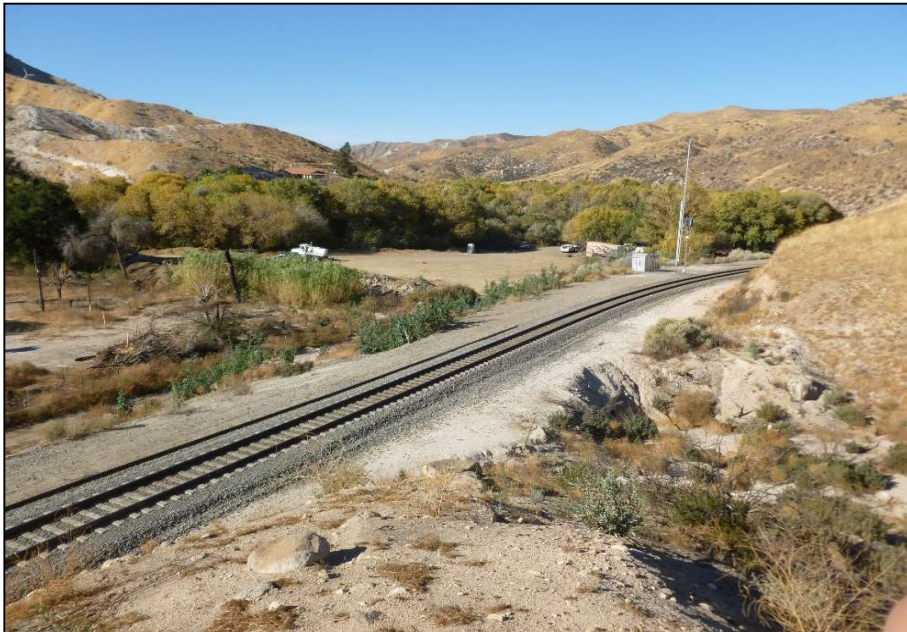
Photograph 2 - The floodplain of the Santa Clara River and a residence on a neighboring property. Looking west-southwest from the westernmost corner of the northern sub-parcel.
