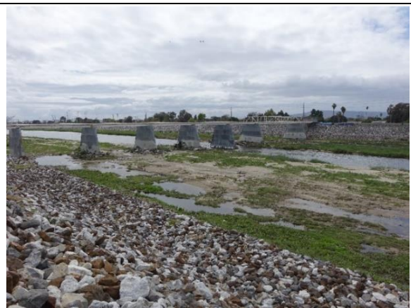
Photo 2: View of the LA River looking southwest from near the LA River Bike Path access point at DeForest Avenue and West 25th Street
