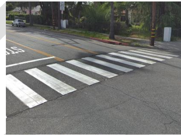
Continental Style Crosswalk, Source: Google Maps
