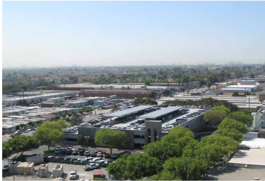
Existing parking structure with Photovoltaic cells
