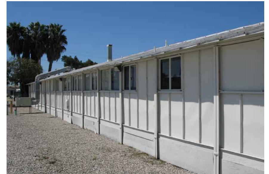
Typical WWII barrack structure
