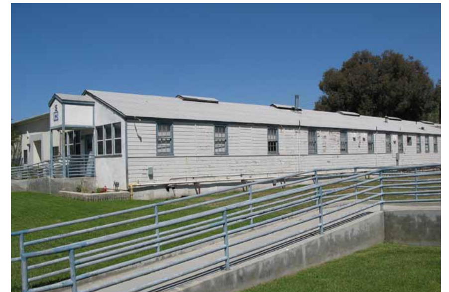
Typical WWII barrack structure
