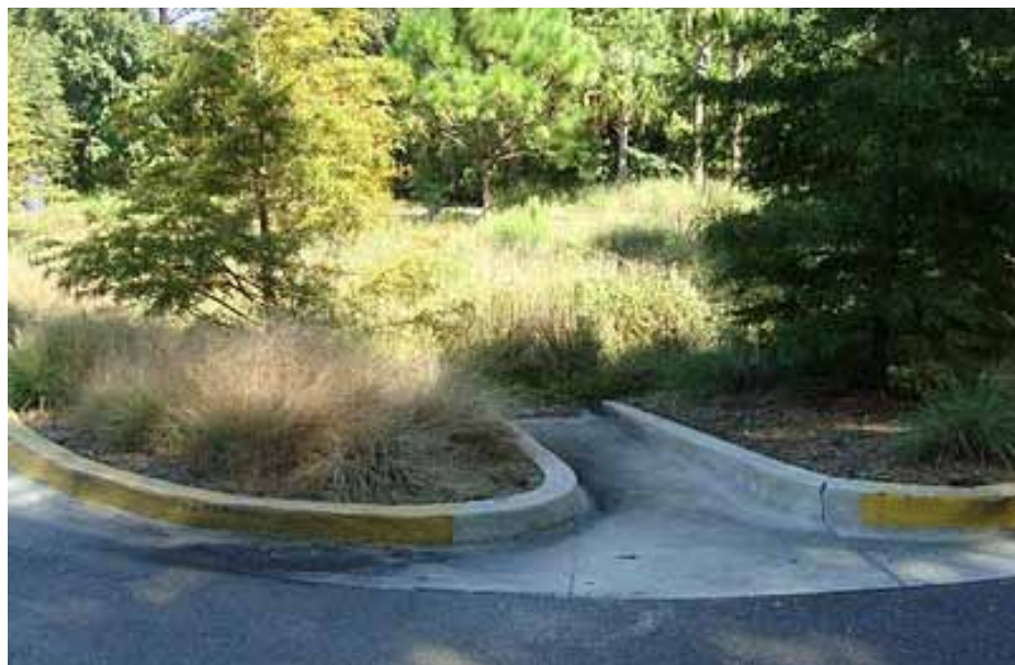
Stormwater directed into bioretention areas
