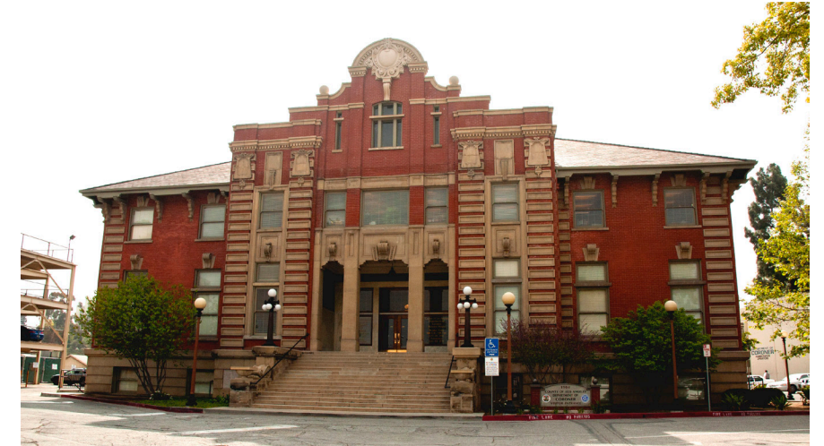
5.79 Historic Hospital Administration Building
