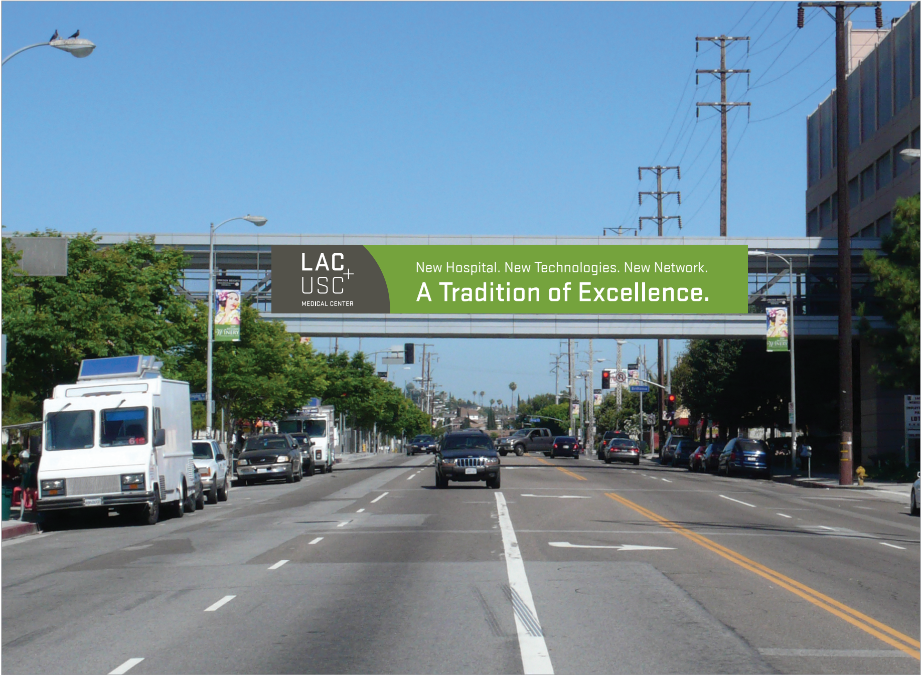
5.116 Marengo Street Pedestrian Bridge from Parking
