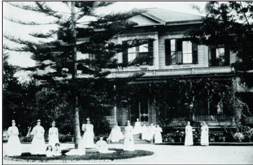
2.02 Original Wood Frame Hospital
