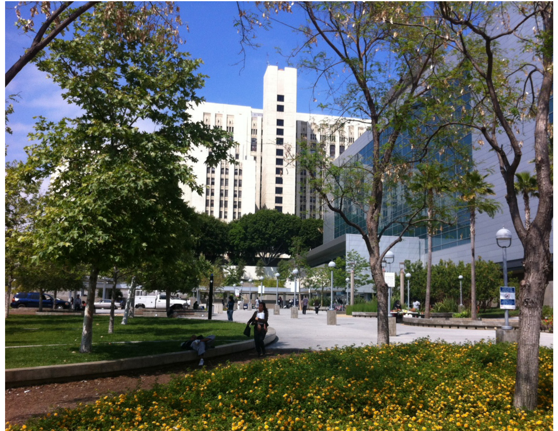
4.16 View of General Hospital through Clinic Tower Courtyard Area
