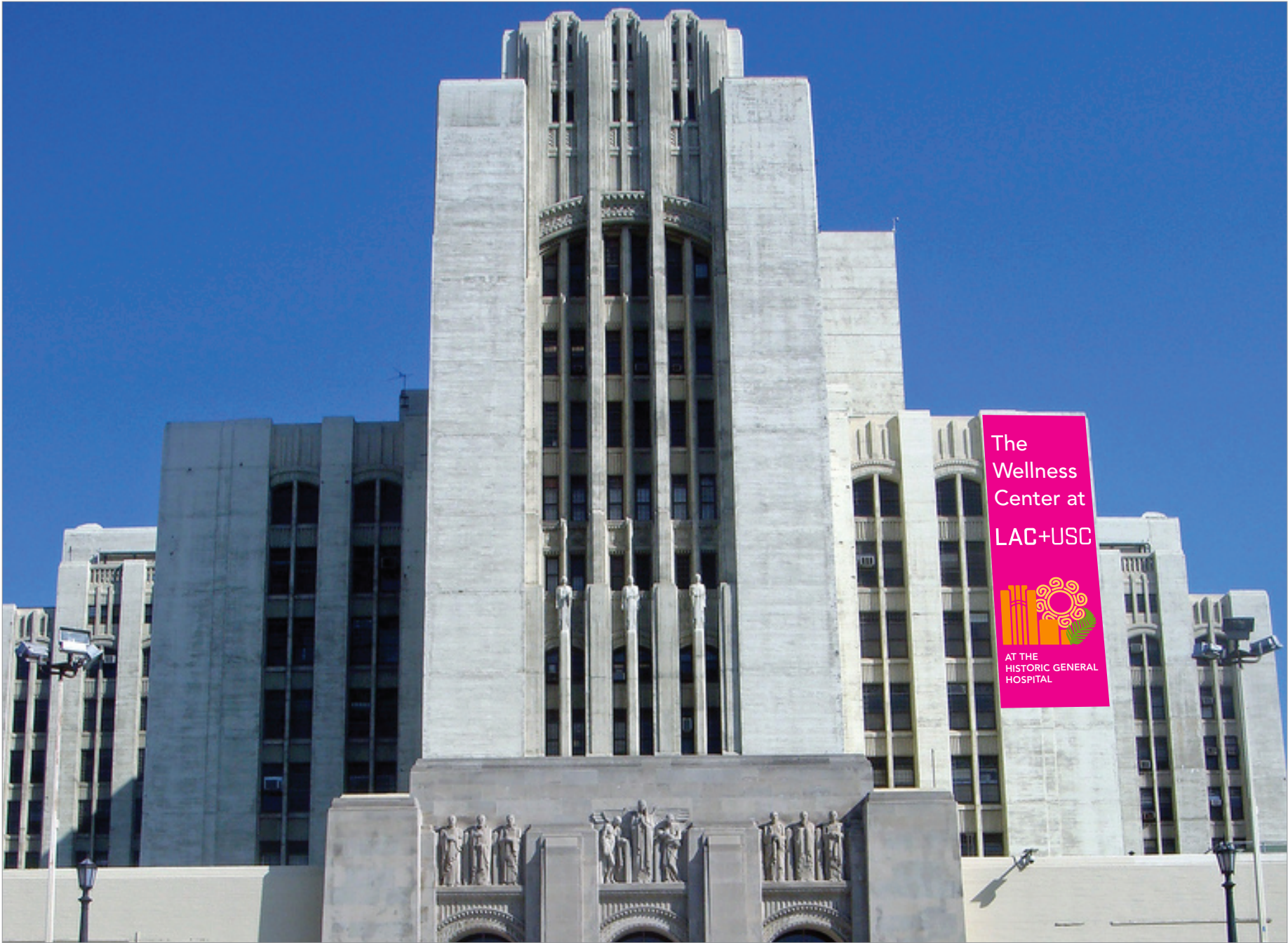
5.114 Historic General Hospital
