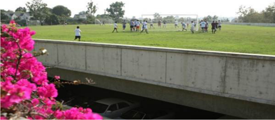
3.09 LMU Drollinger Parking Structure & Leavey Field
