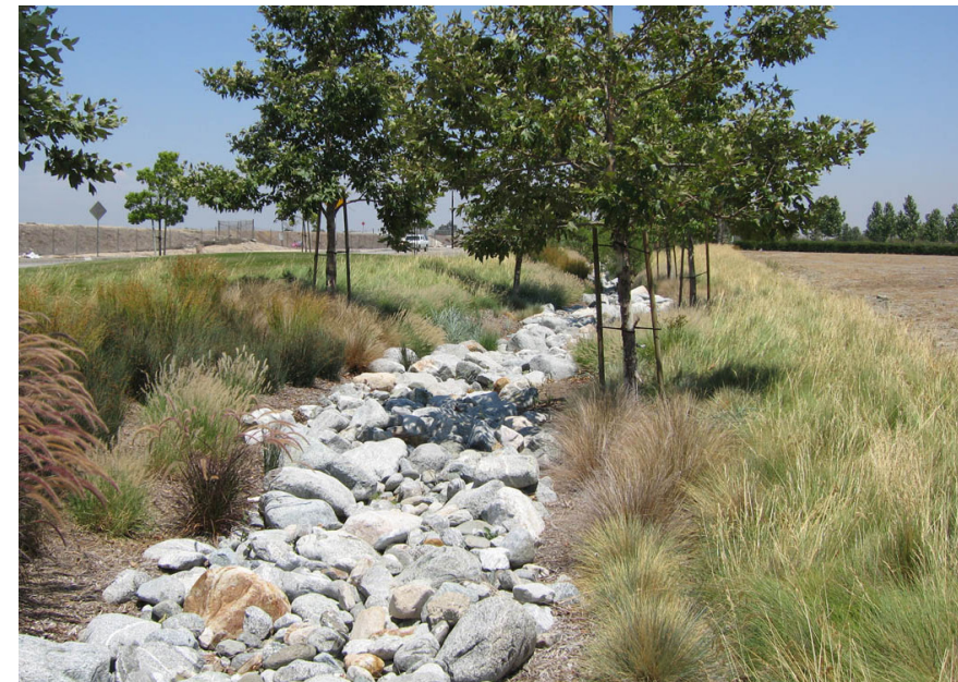
5.100 Storm Water Treatment
