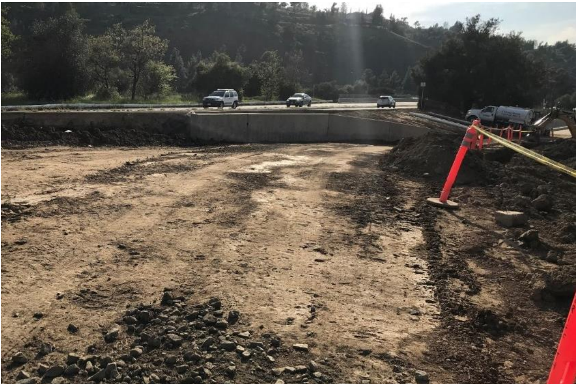
3/26/19 – Imported fill is building up east access road for direct access off Oak Grove Drive.
