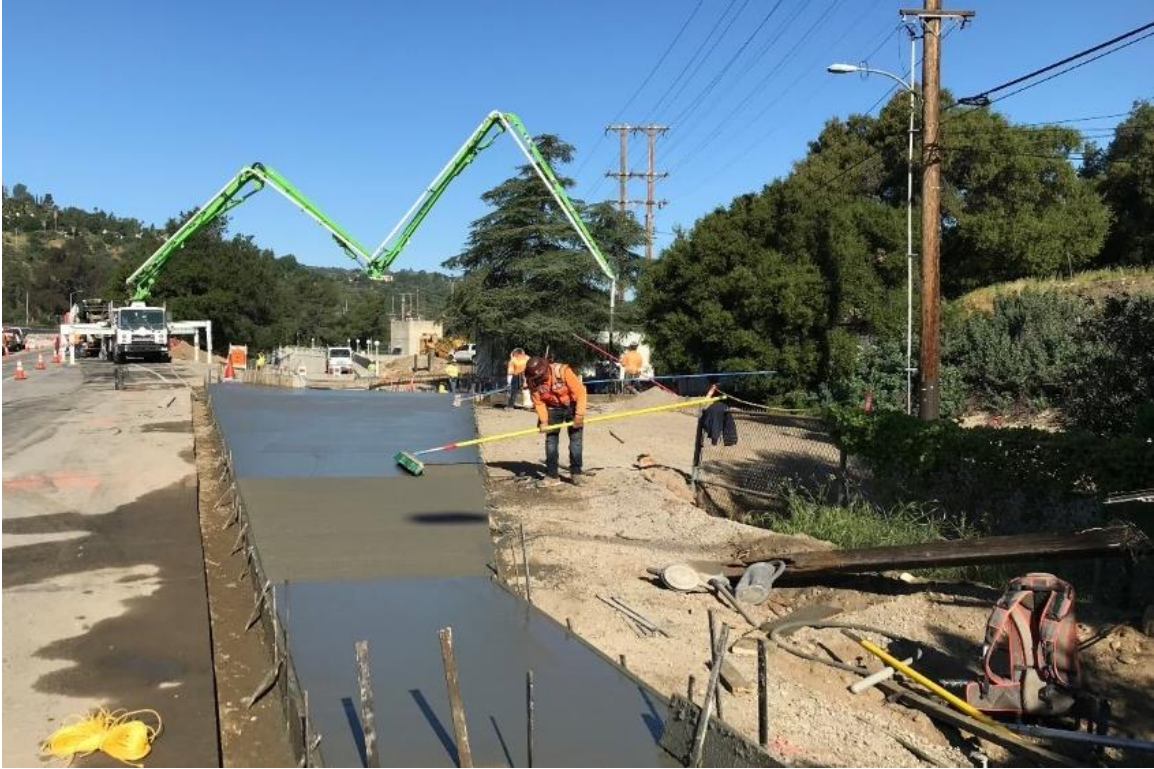
4/12/19 – Pouring concrete for east access road
