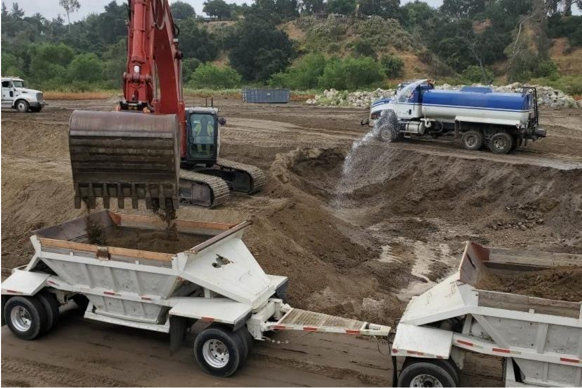
6/5/20 – Watering operation at excavation area while loading sediment haul trucks
