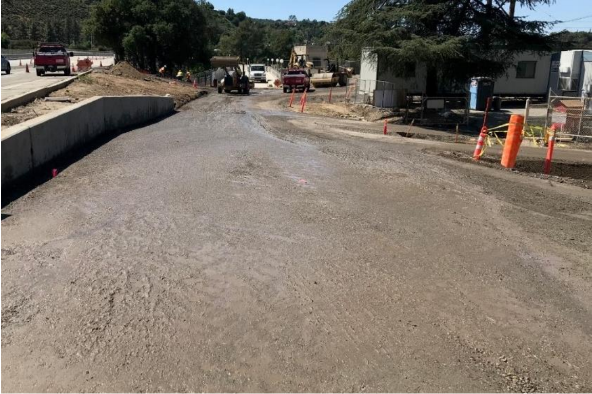
4/10/19 – Base material compacted on east access road.
