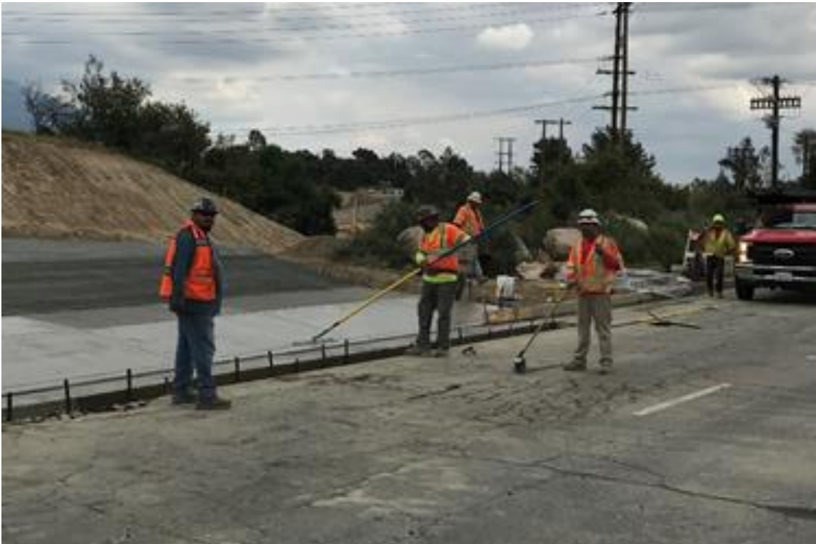
4/3/19 – Pouring concrete pavement for west access road driveway.
