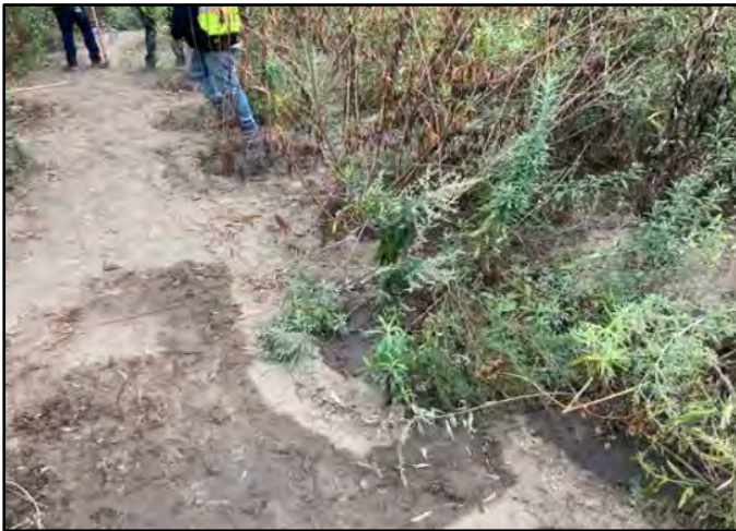
Photo Number: 41 Location: DG-2/DG2B Description: Before Basin Maintenance
