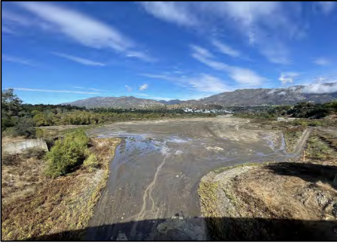
Photo Number: 22 Date: 11/01/2022 Description: Post-Annual Maintenance Cleanout Overview Project
