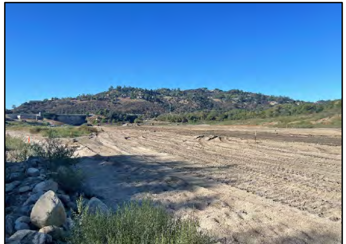
Photo Number: 18 Date: 9/20/2022 Description: Upstream Portion View Looking South
