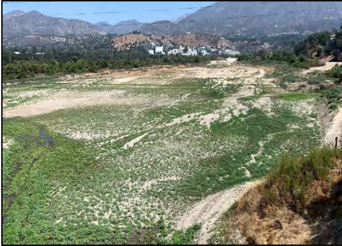
Photo Number: 15 Date: 8/28/2022 Description: Pre-Annual Maintenance Cleanout Overview
