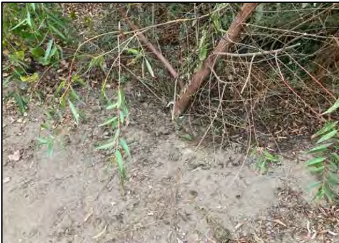
Photo Number: 33 Location: DG-2B Area Description: Before Basin Maintenance
