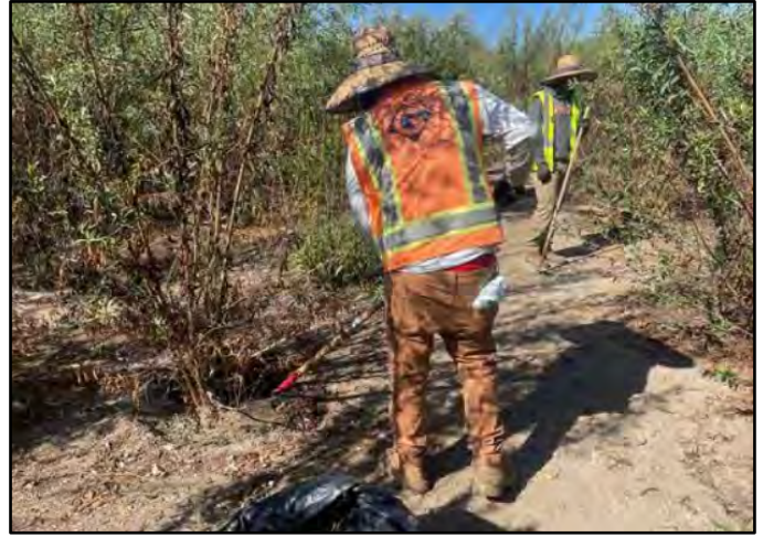
Photo Number: 40 Location: DG-W-1 (Johnson Field) Description: Reshaping Basins
