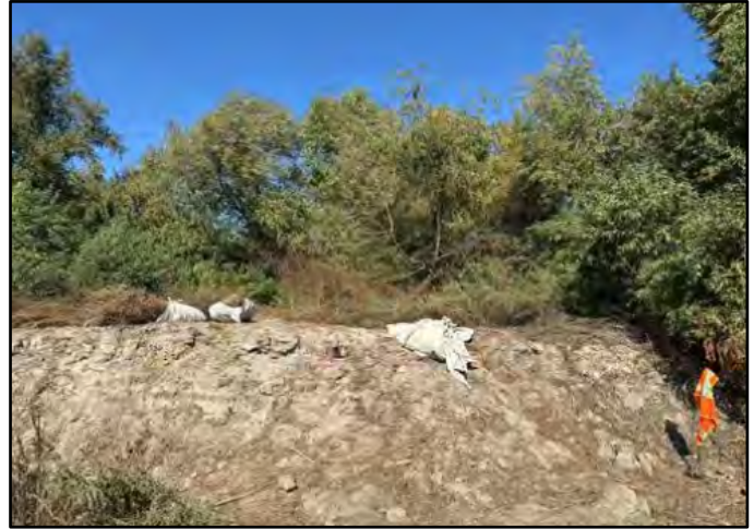
Photo Number: 44 Location: DG-4A Slope Description: After Weed Removal
