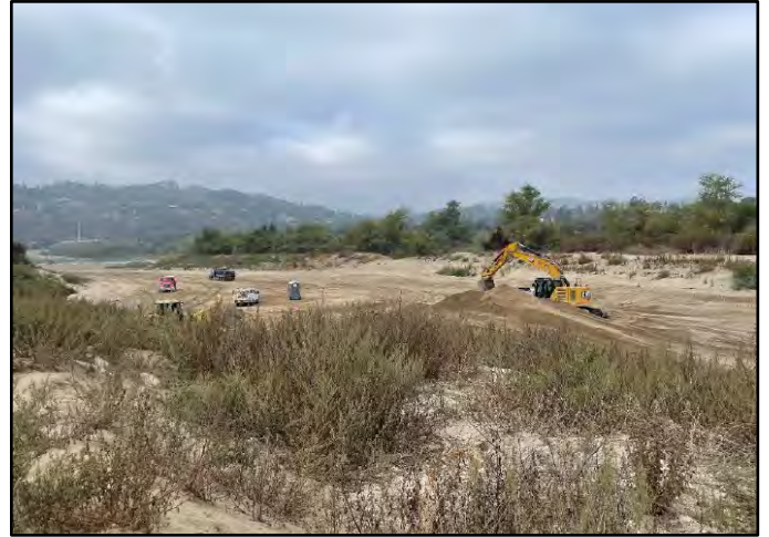
Photo Number: 20 Date: 10/12/2022 Description: Crew Working on Site
