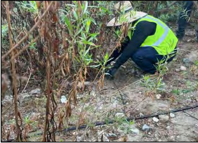
Photo Number: 39 Location: DG-W-1 (Johnson Field) Description: Fixing Irrigation Line
