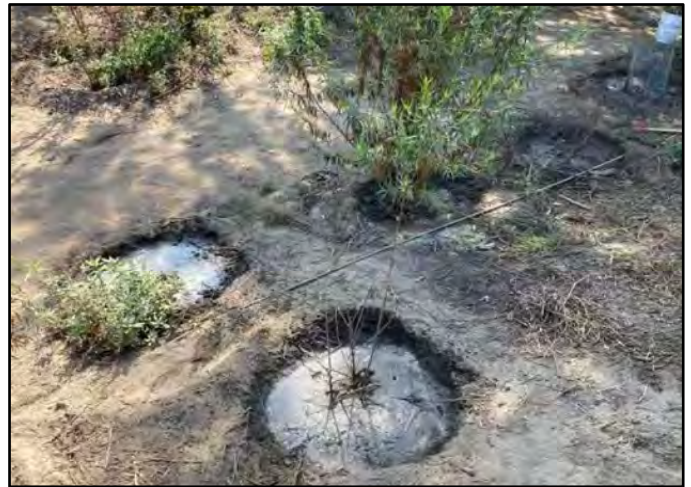
Photo Number: 42 Location: DG-2/DG2B Description: After Basin Maintenance
