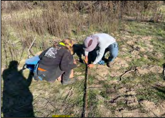
Photo Number: 31 Location: DG-4 Area Description: Irrigation Maintenance
