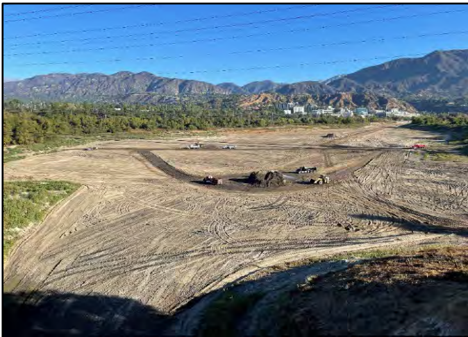
Photo Number: 17 Date: 9/20/2022 Description: Start of Sediment Hauling Overview of Site
