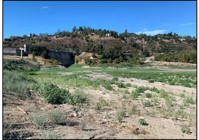
Photo Number: 16 Date: 8/28/2022 Description: Upstream Portion View Looking South
