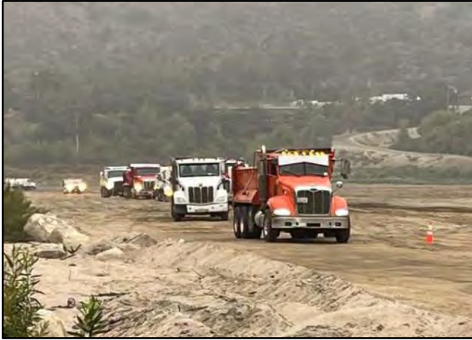
Photo Number: 13 Location: North of the Reservoir Description: Dump Trucks Lining up to Collect Sediment
